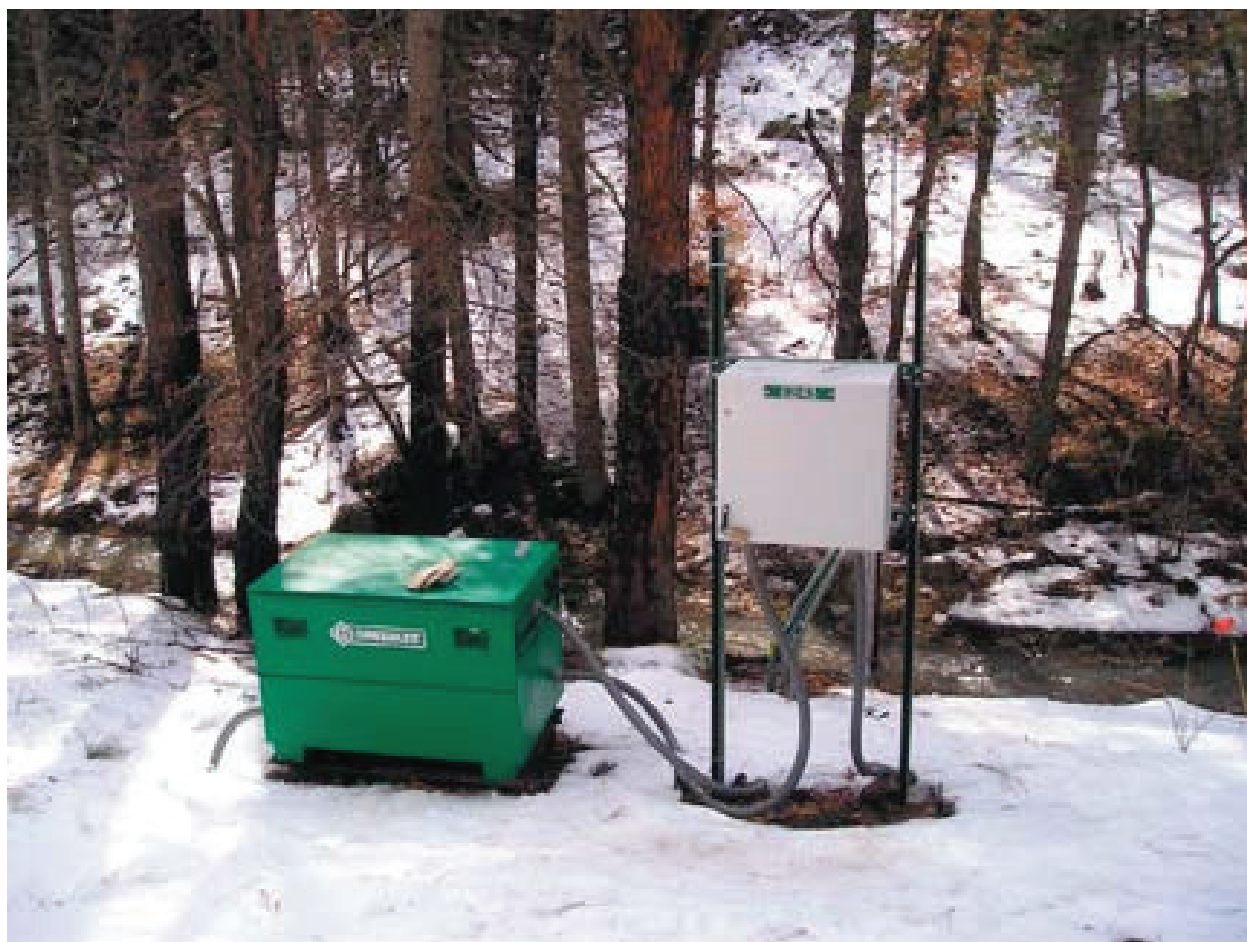
E243 Stream gaging station, downstream view
