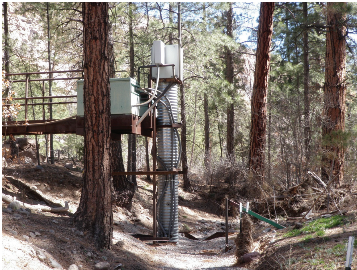
E030 Stream gaging station, downstream view
