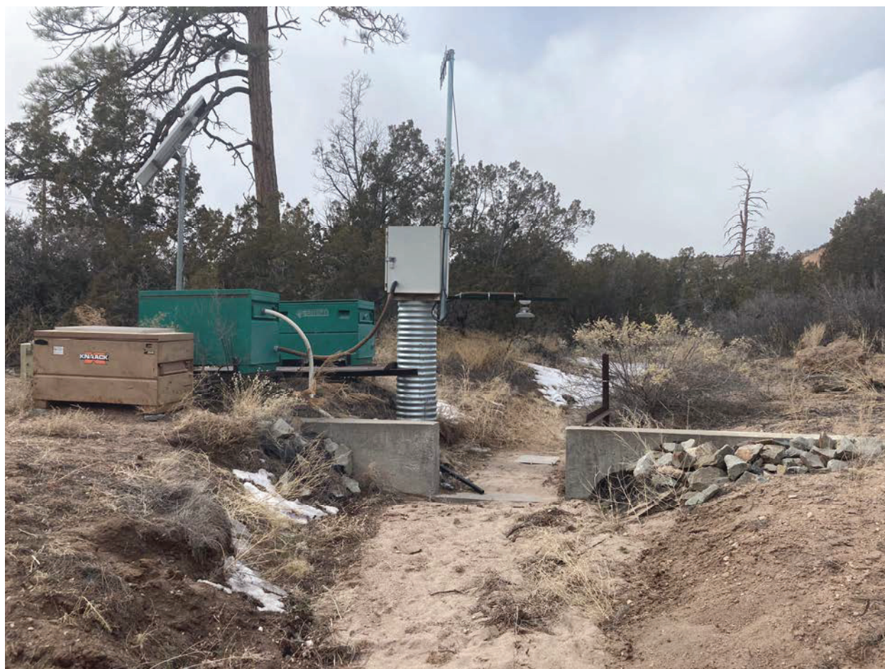
E125 Stream gaging station, upstream view
