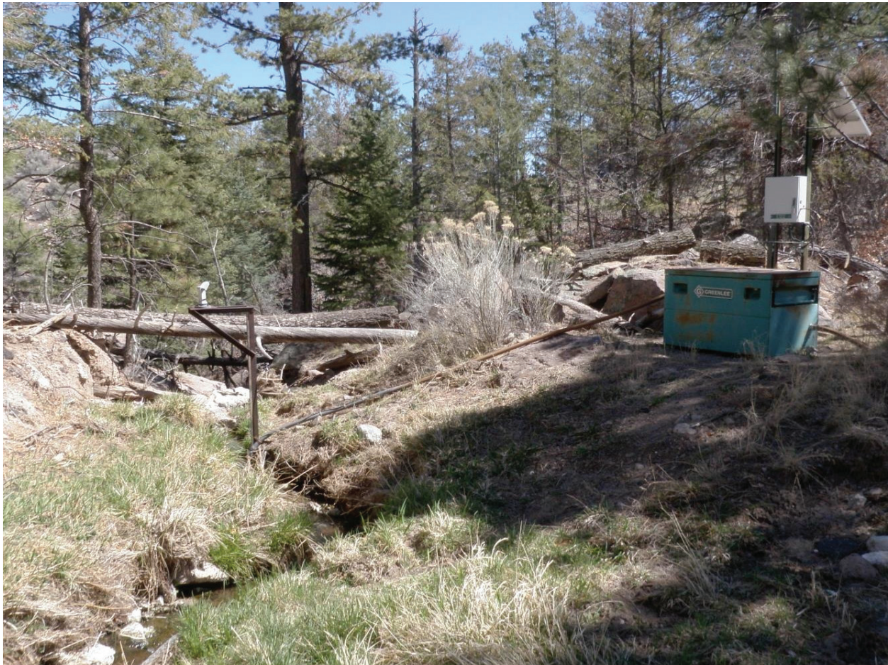
E122 Stream gaging station, downstream view
