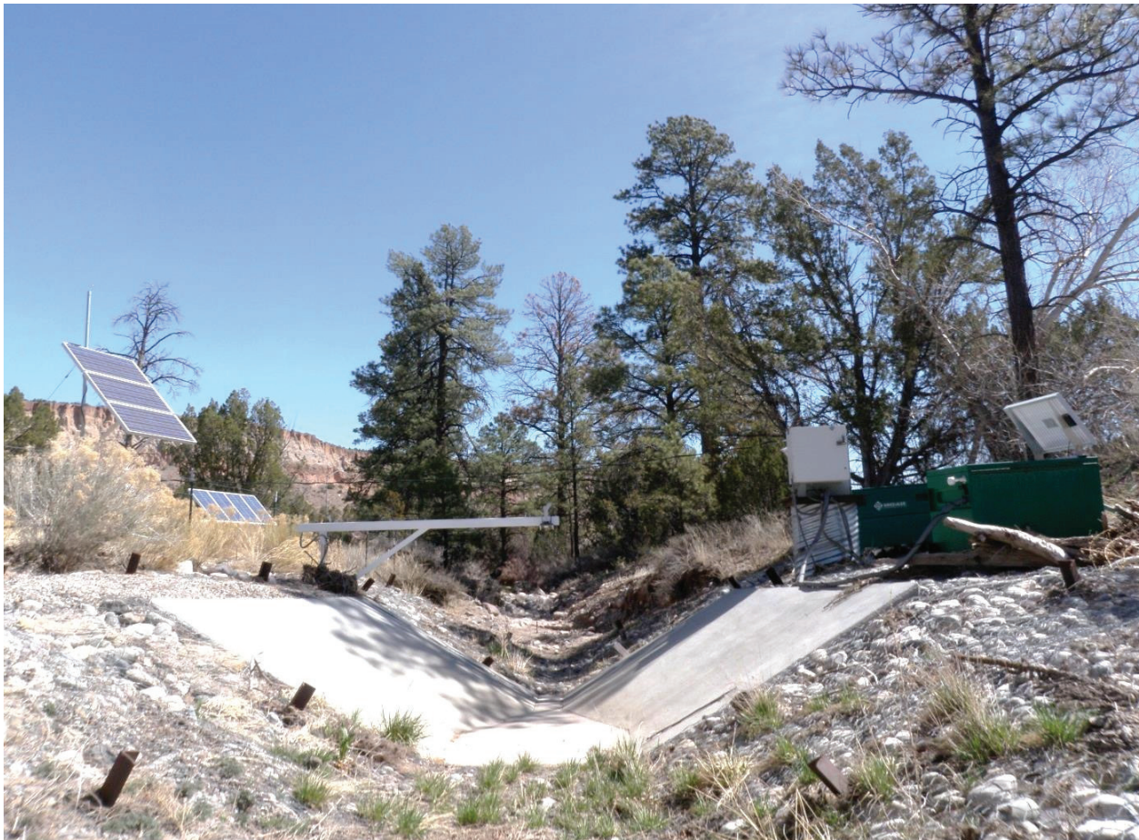
E050.1 Stream gaging station, downstream view
