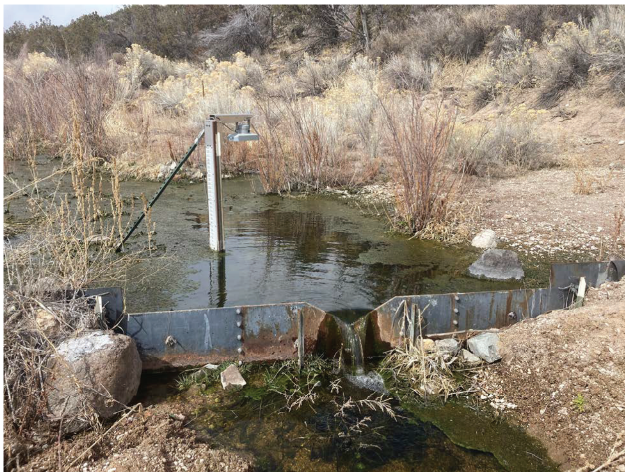
E059.8 Stream gaging station, upstream view
