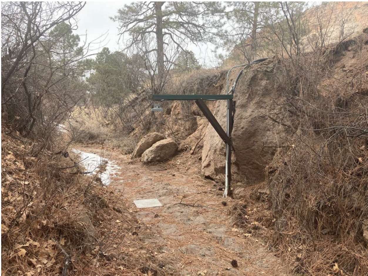
E124 Stream gaging station, downstream view
