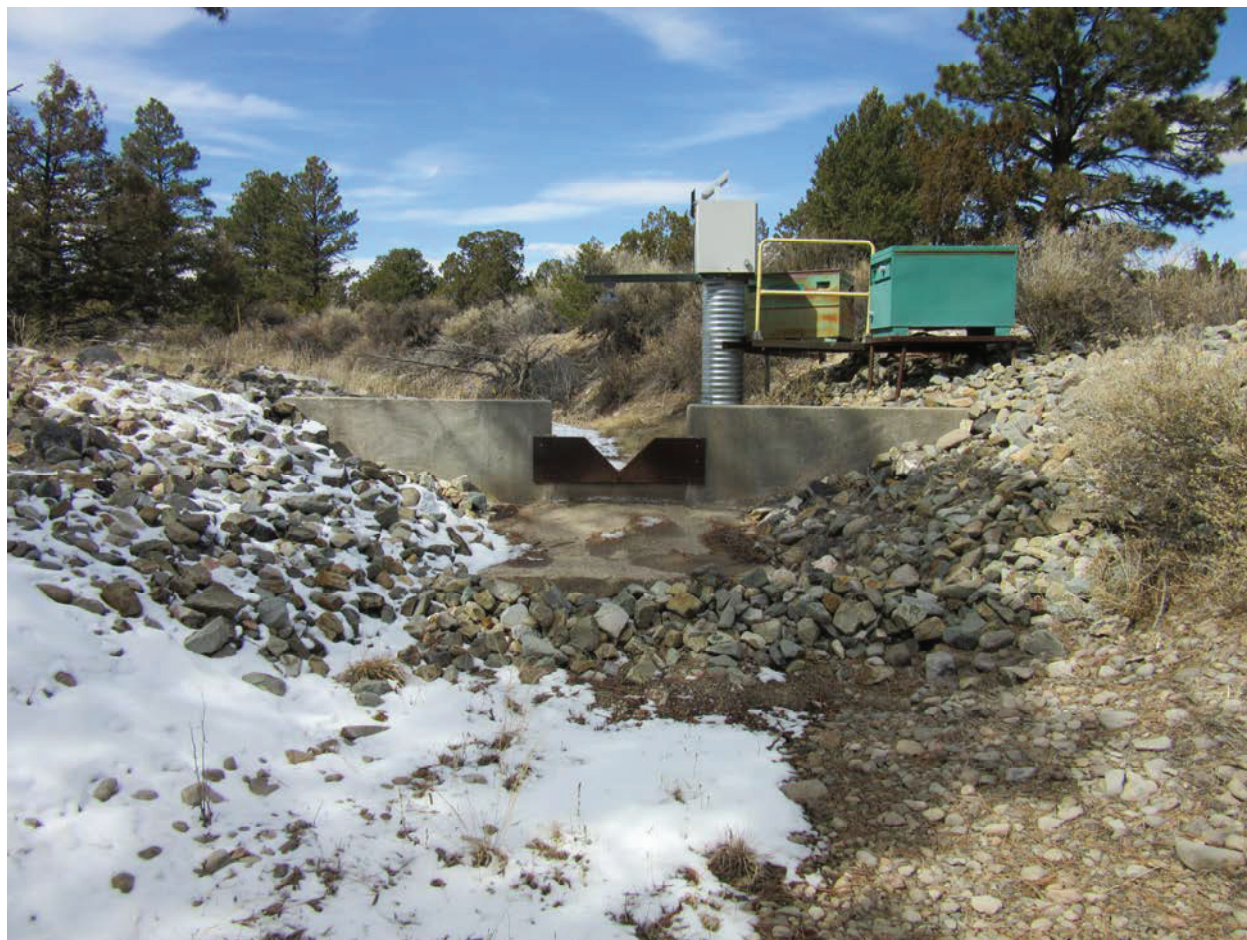
E250 Stream gaging station, upstream view
