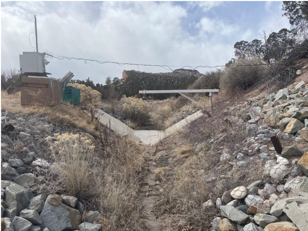
E060.1 Stream gaging station, upstream view
