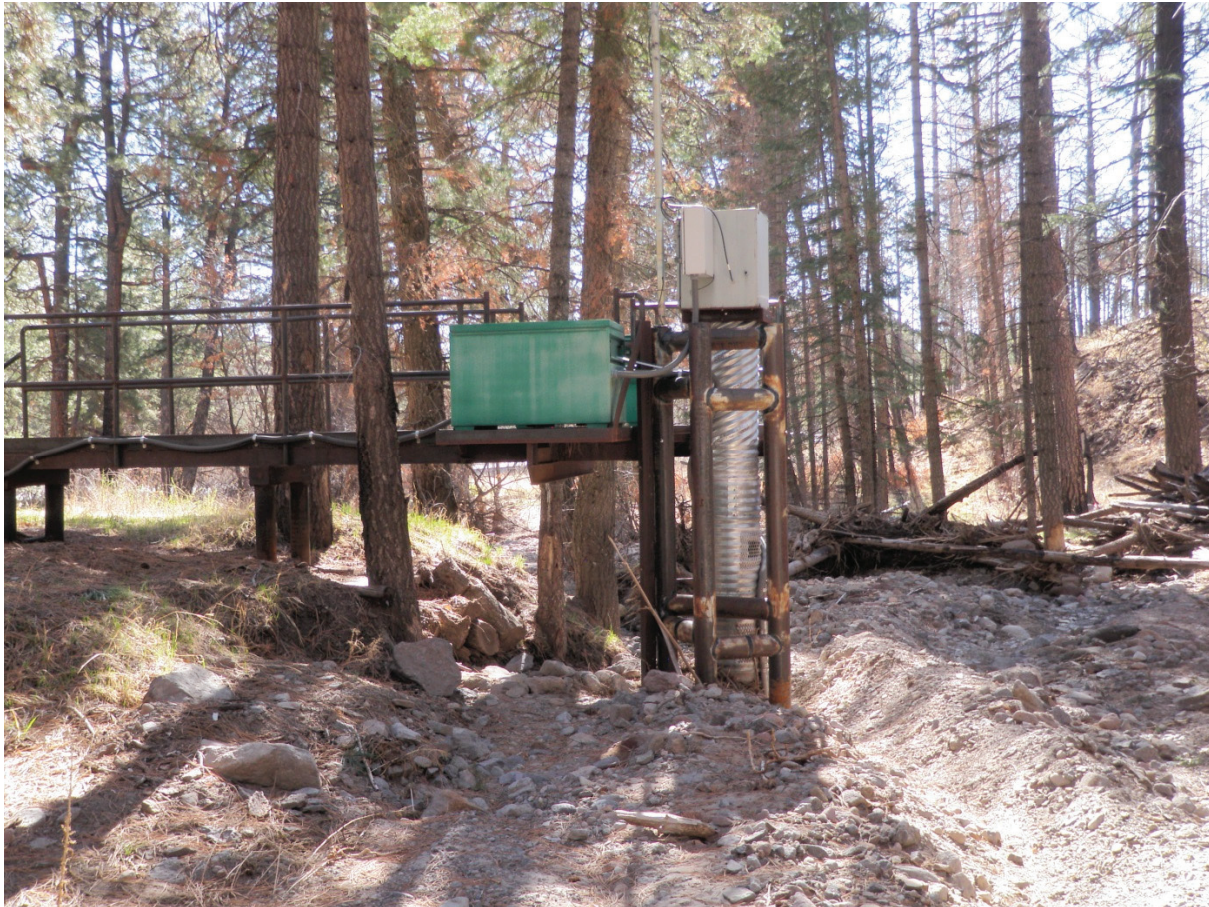
E252 Stream gaging station, downstream view
