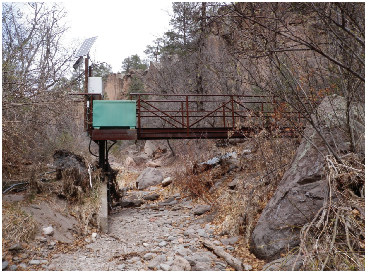
E055 Stream gaging station, upstream view
