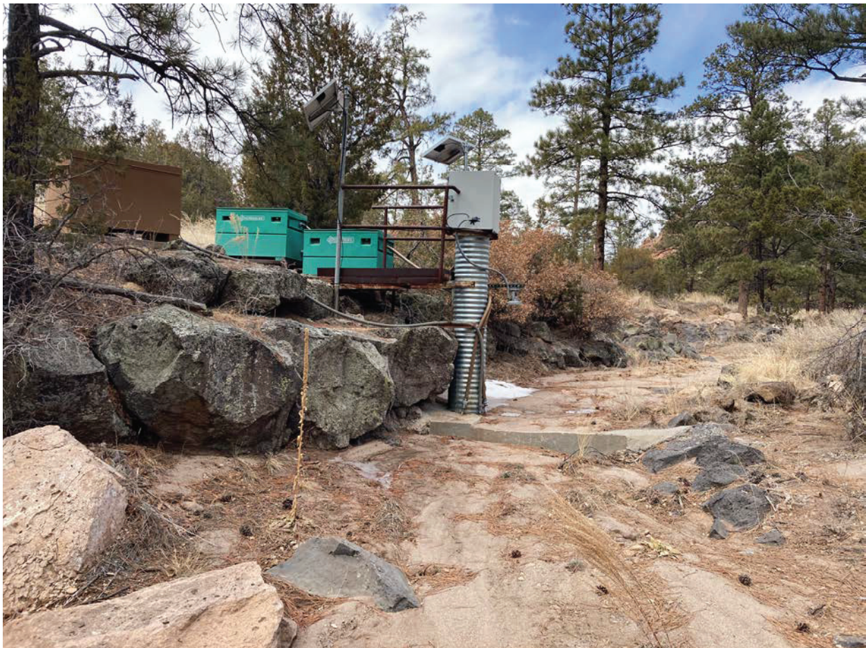
E275 Stream gaging station, upstream view
