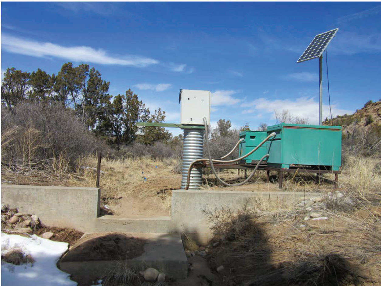
E267 Stream gaging station, upstream view
