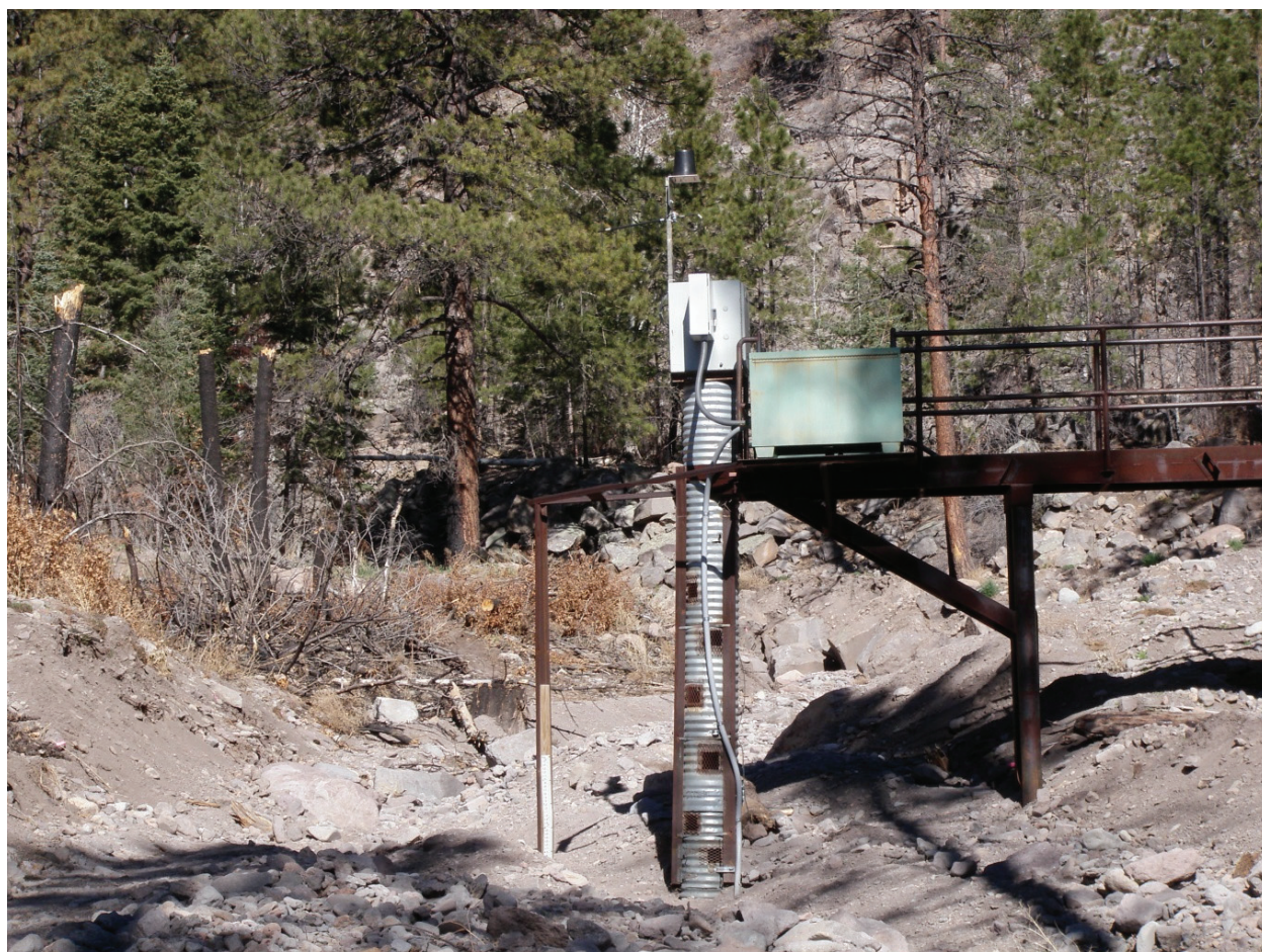
E253 Stream gaging station, upstream view
