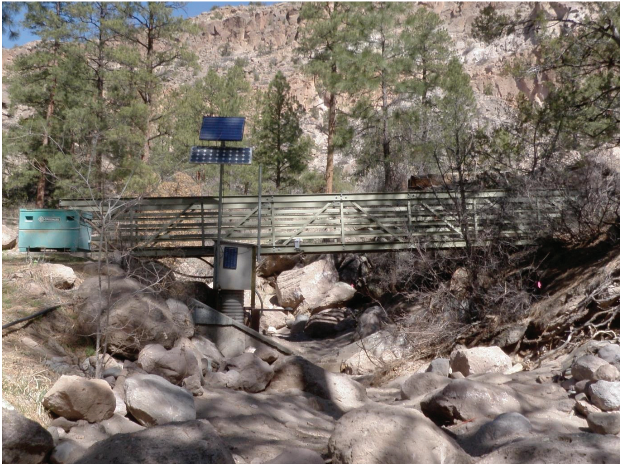
E040 Stream gaging station, upstream view
