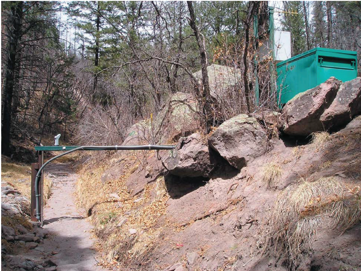
E244 Stream gaging station, upstream view
