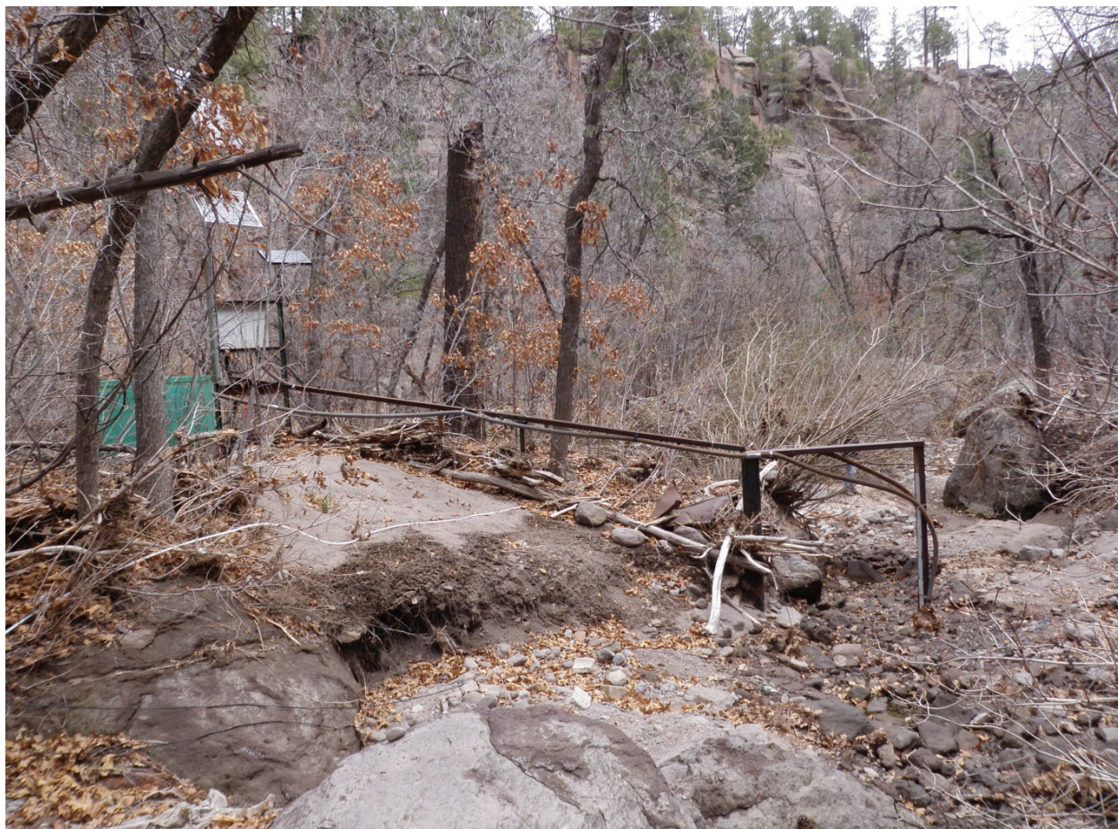
E056 Stream gaging station, downstream view
