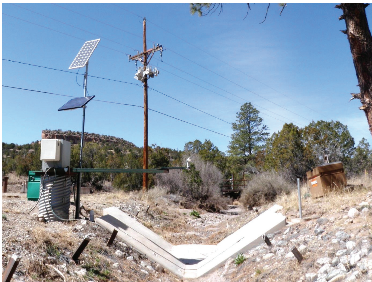
E042.1 Stream gaging station, upstream view
