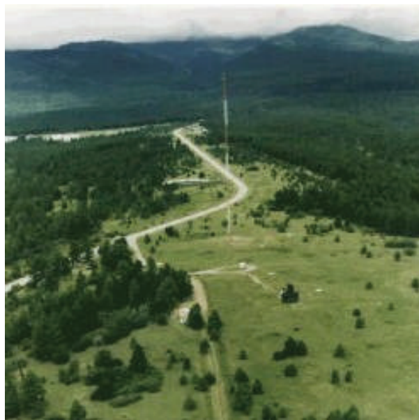
RG-TA-06 Meteorological tower
