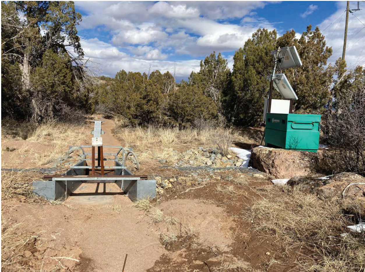
E229.3 Stream gaging, downstream view
