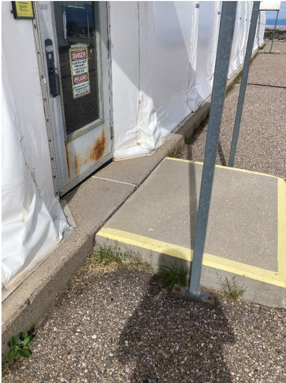
Pictures of exterior stoops to show alignment of asphalt, stoop, and awning pinning.
