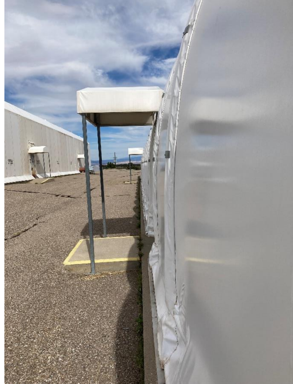
Pictures of exterior stoops to show alignment of asphalt, stoop, and awning pinning.
