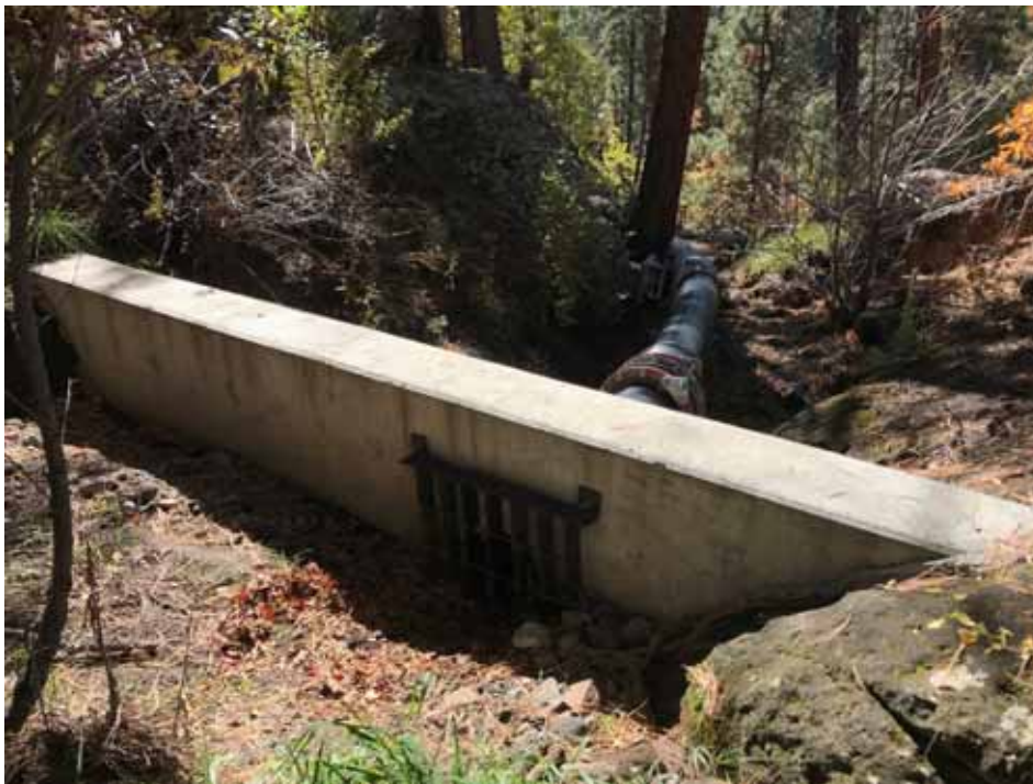
Photo C-3.4-2 October 2022—Pipeline headwall
