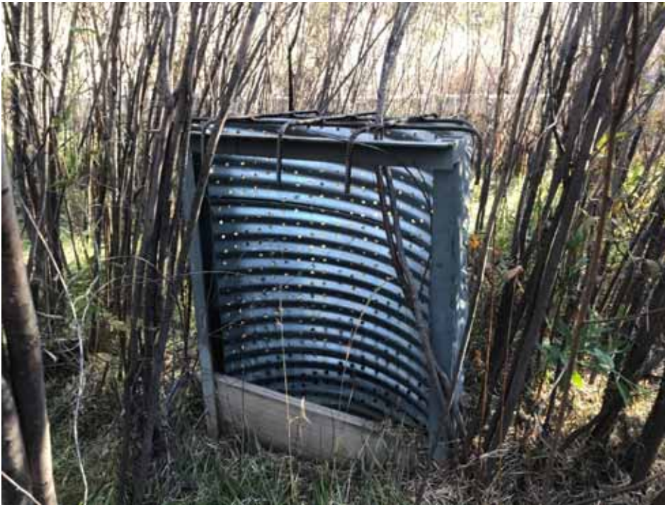
Photo C-2.3-2 October 2022—Standpipe. Sediment level is approximately 1 ft below wood stop board. No significant change since last inspection. Continue to monitor.
