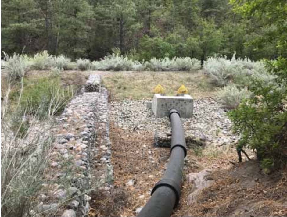
Photo C-3.4-11 May 2022—Pipeline outlet, energy dissipater, and gabion overflow structure
