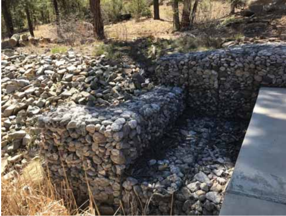
Photo C-2.4-1 May 2022—GCS spillway and flow-way, looking south
