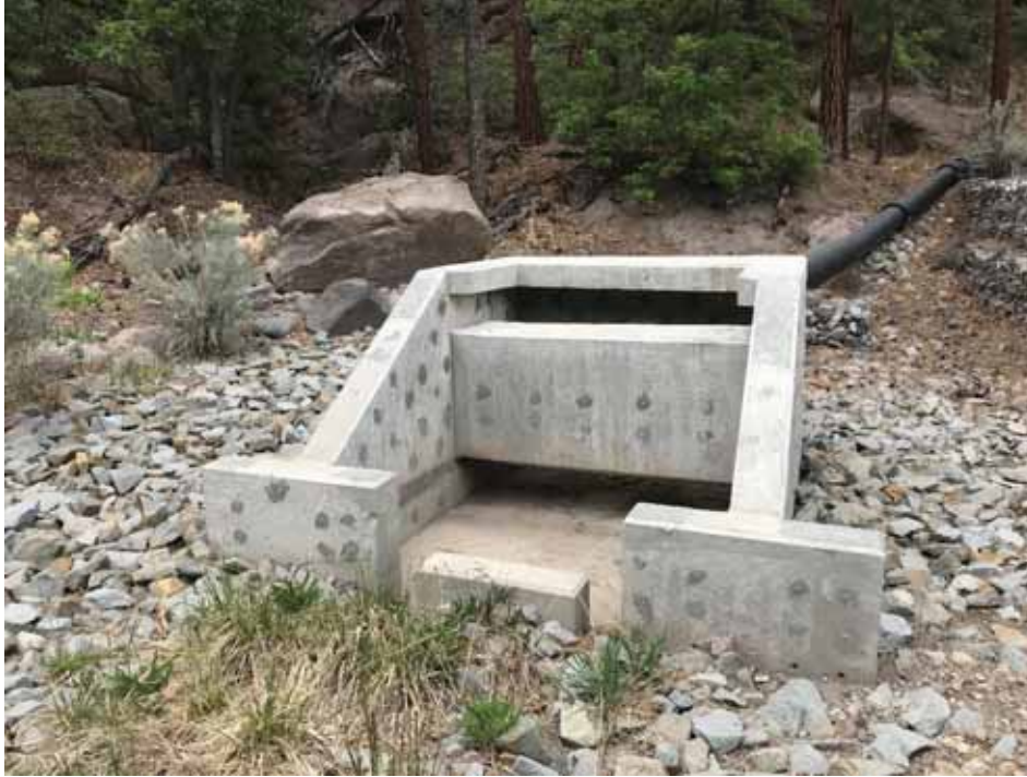
Photo C-3.4-13 May 2022—Pipeline energy dissipater
