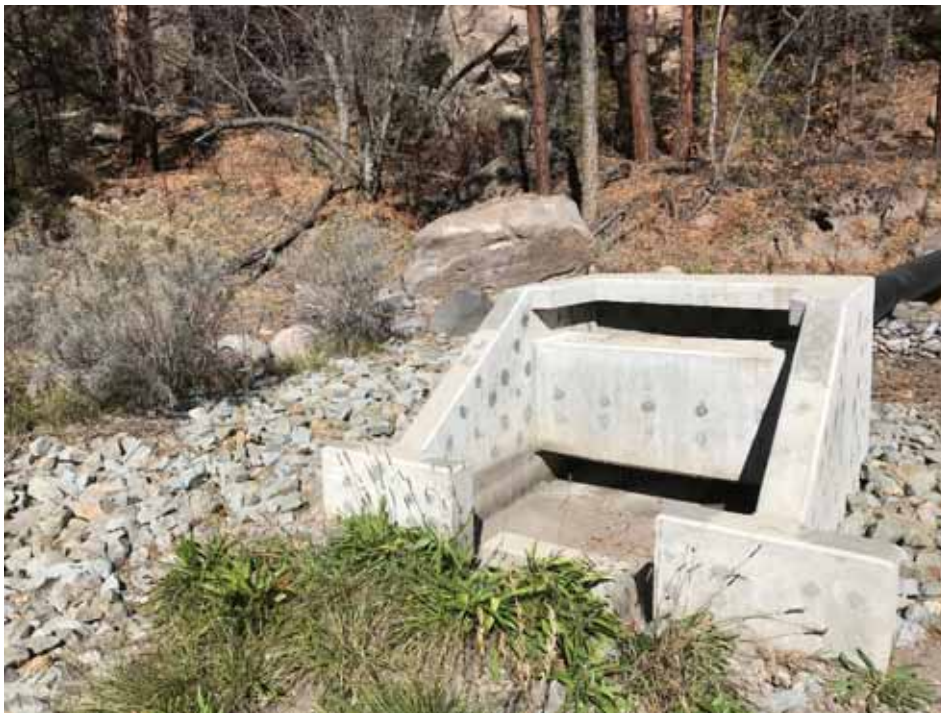
Photo C-3.4-14 October 2022—Pipeline energy dissipater
