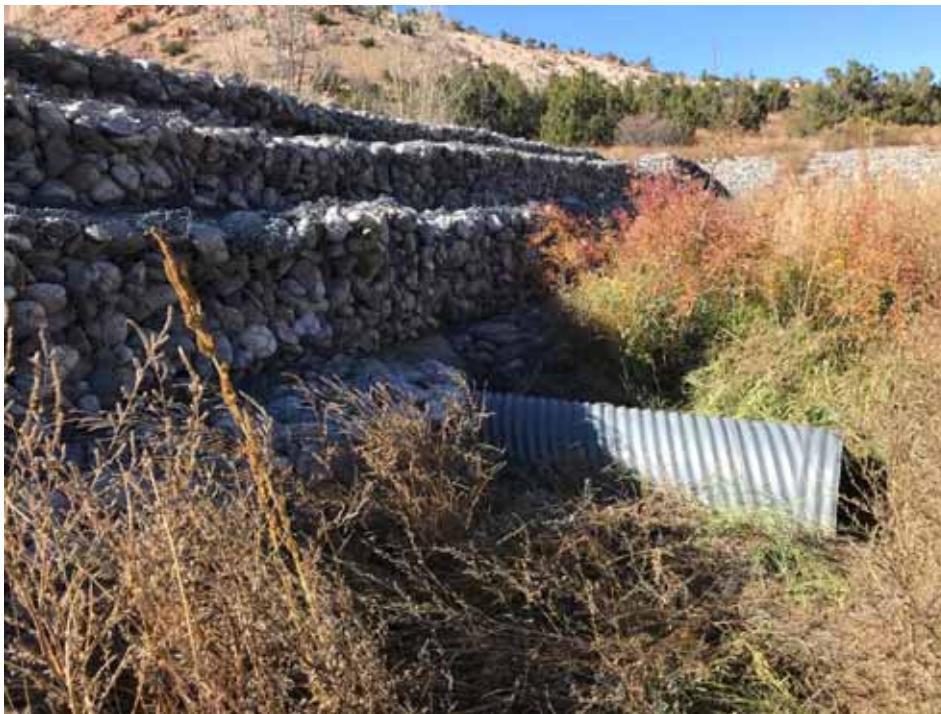
Photo C-4.5-2 October 2022—Weir outlet. Approximately 4 ft of culvert is undercut; continue monitoring.
