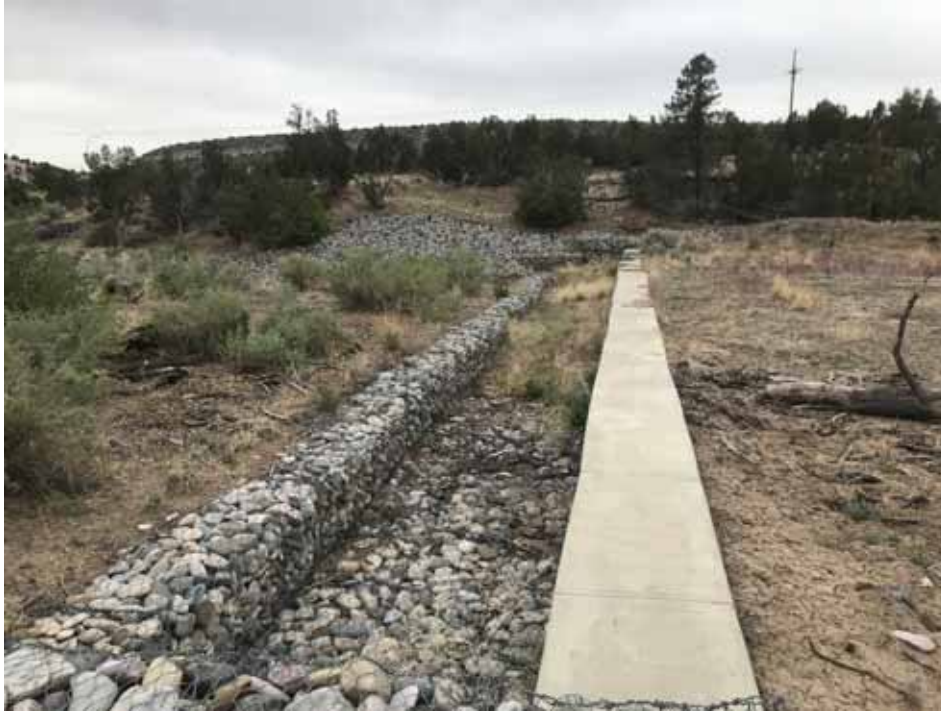
Photo C-5.2-1 May 2022—Weir crest and flow-ways, looking south
