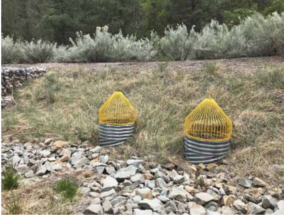
Photo C-3.4-15 May 2022—Discharge culvert inlets and trash racks
