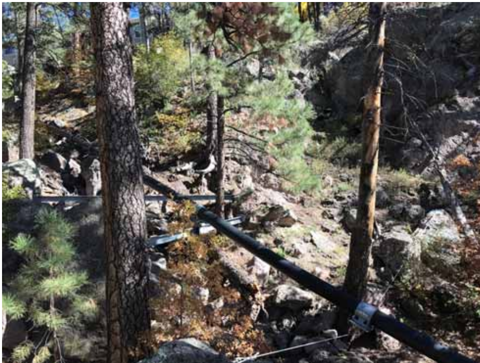
Photo C-3.4-4 October 2022—Pipeline supports. Downed tree was removed from support beam.
