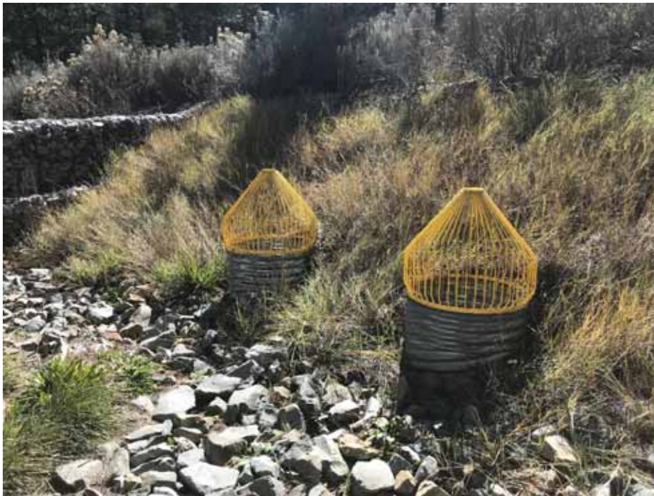
Photo C-3.4-16 October 2022—Discharge culvert inlets and trash racks
