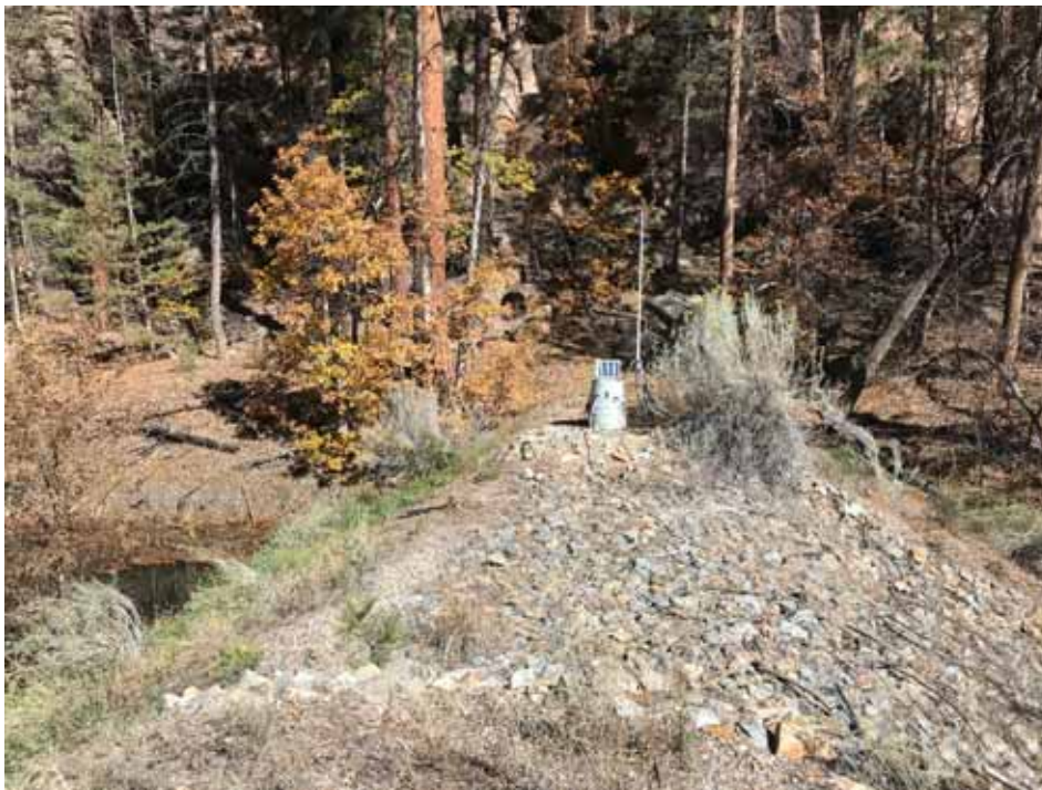
Photo C-3.2-2 October 2022—Lower basin spillway, looking north. Vegetation was removed from spillway during inspection.
