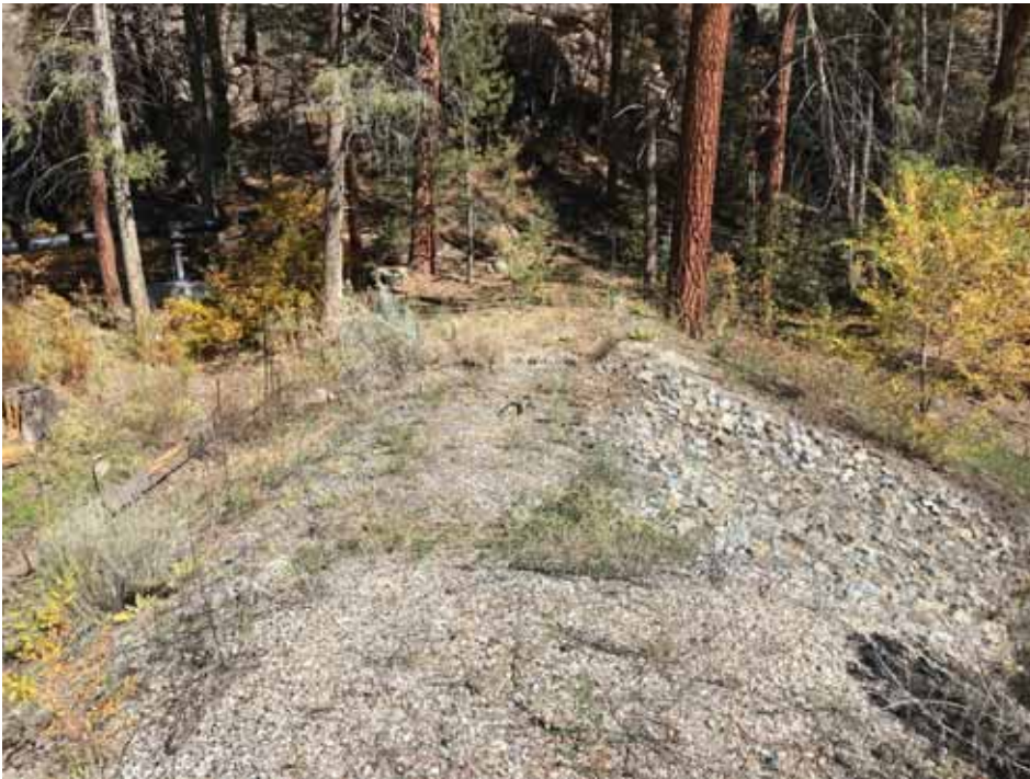
Photo C-3.2-4 October 2022—Upper basin spillway, looking north. Vegetation was removed from spillway during inspection.
