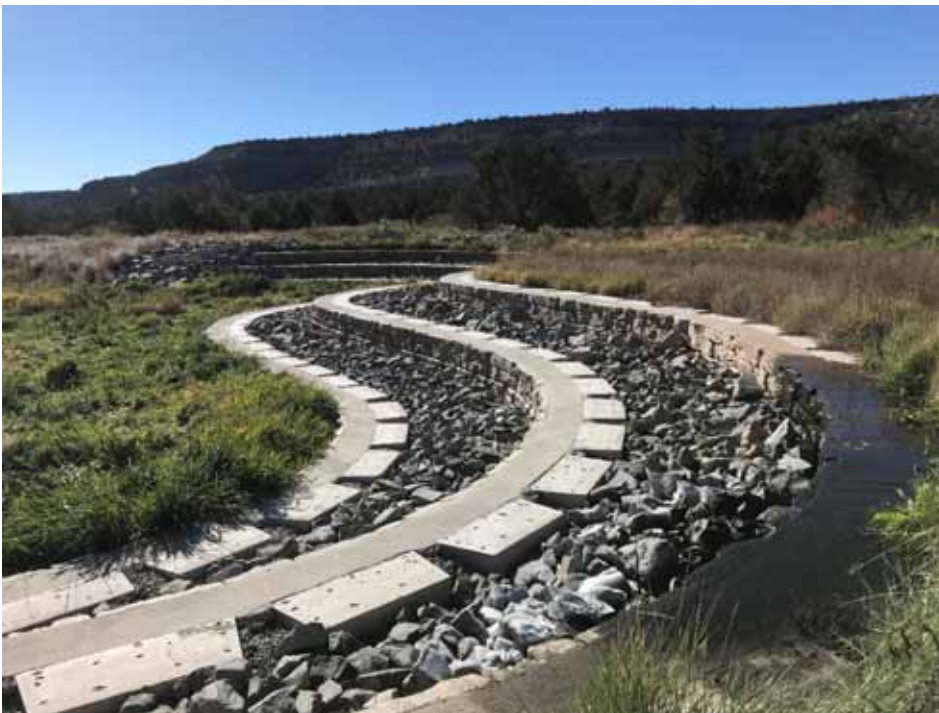
Photo C-6.1-4 October 2022—Redi-Rock block structure, looking southeast. Note flow over crest.
