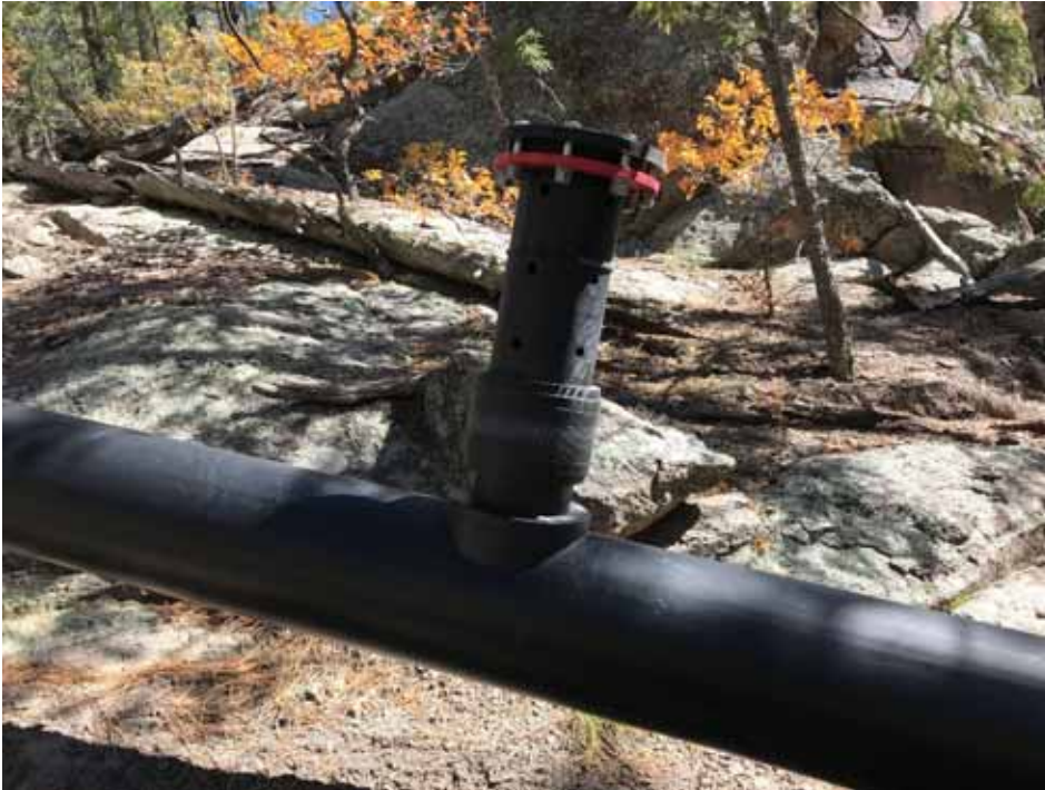
Photo C-3.4-8 October 2022—Pipeline vacuum breaker
