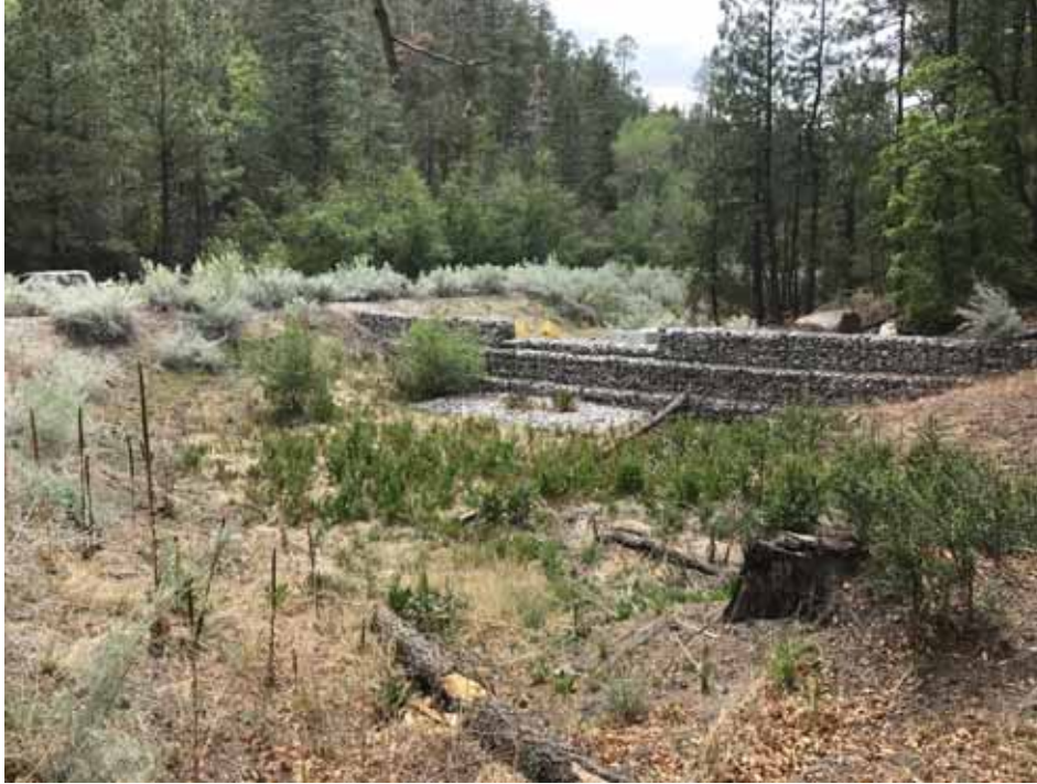
Photo C-3.1-3 May 2022—Upper basin, looking southwest at gabion overflow structure
