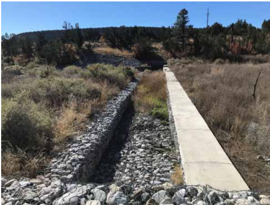
Photo C-5.2-2 October 2022—Weir crest and flow-ways, looking south
