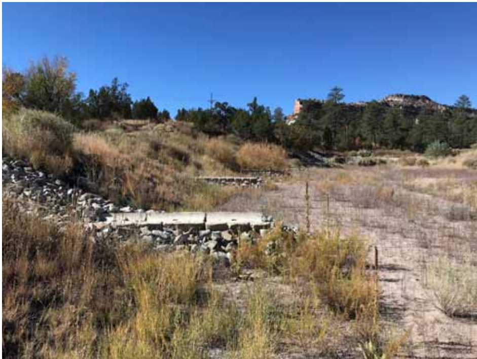
Photo C-5.4-2 October 2022—Redi-rock spurs, looking west/upstream
