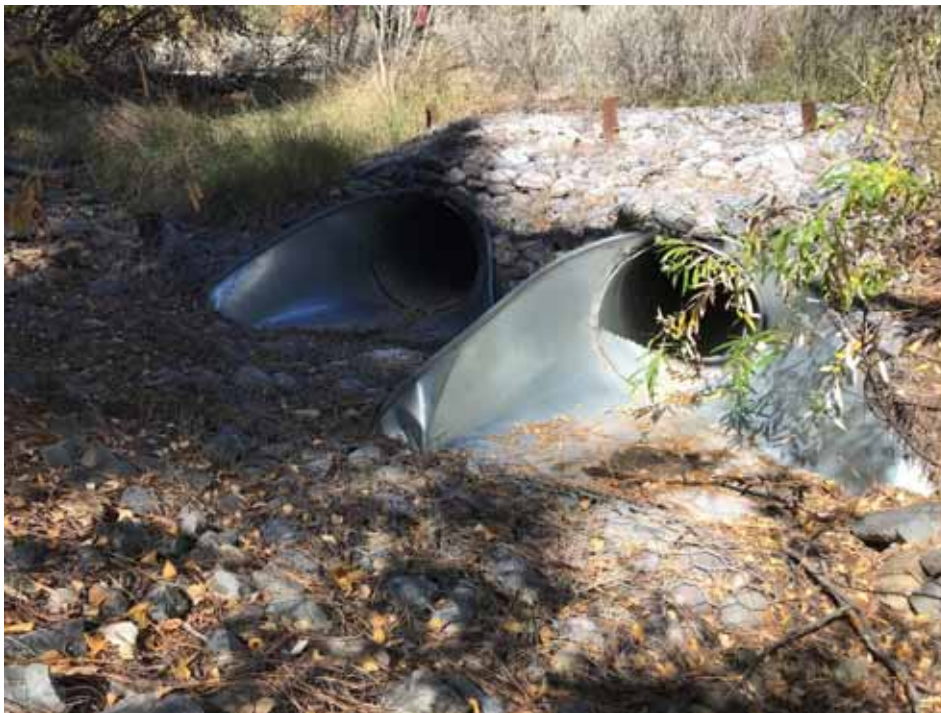
Photo C-3.4-18 October 2022—Discharge culvert outlets and bank protection
