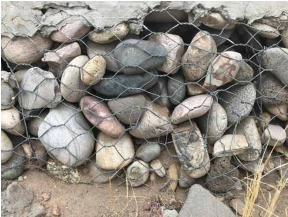
Photo C-5.5-2 May 2022—Repaired flow-way gabion basket
