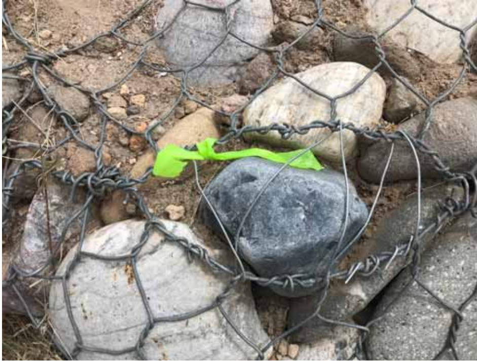
Photo C-5.5-1 May 2022—Repaired flow-way gabion basket seam
