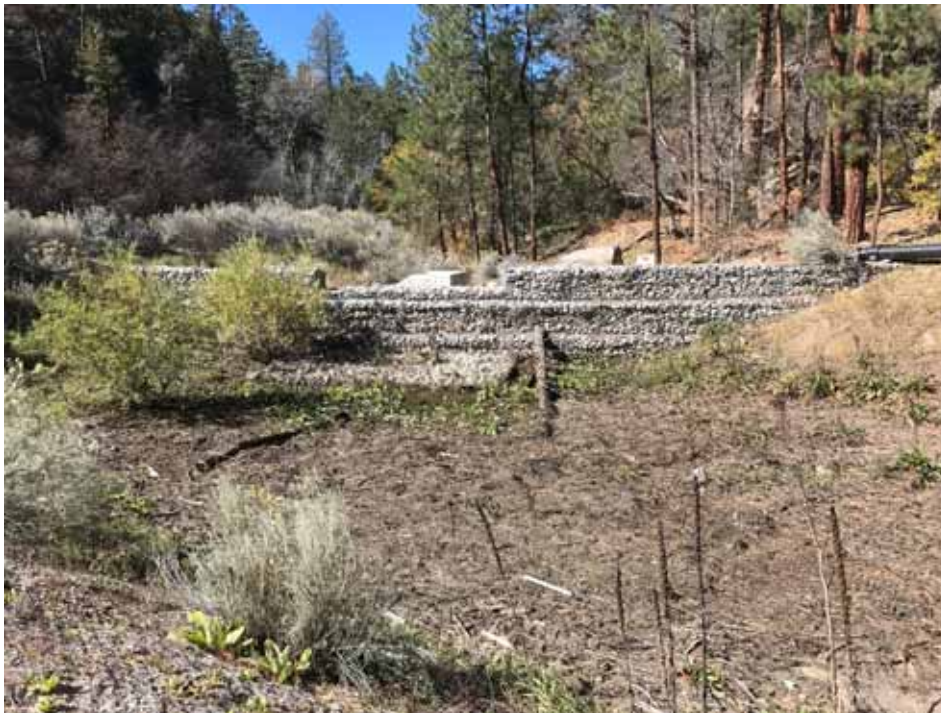
Photo C-3.1-4 October 2022—Upper basin, looking west at gabion overflow structure
