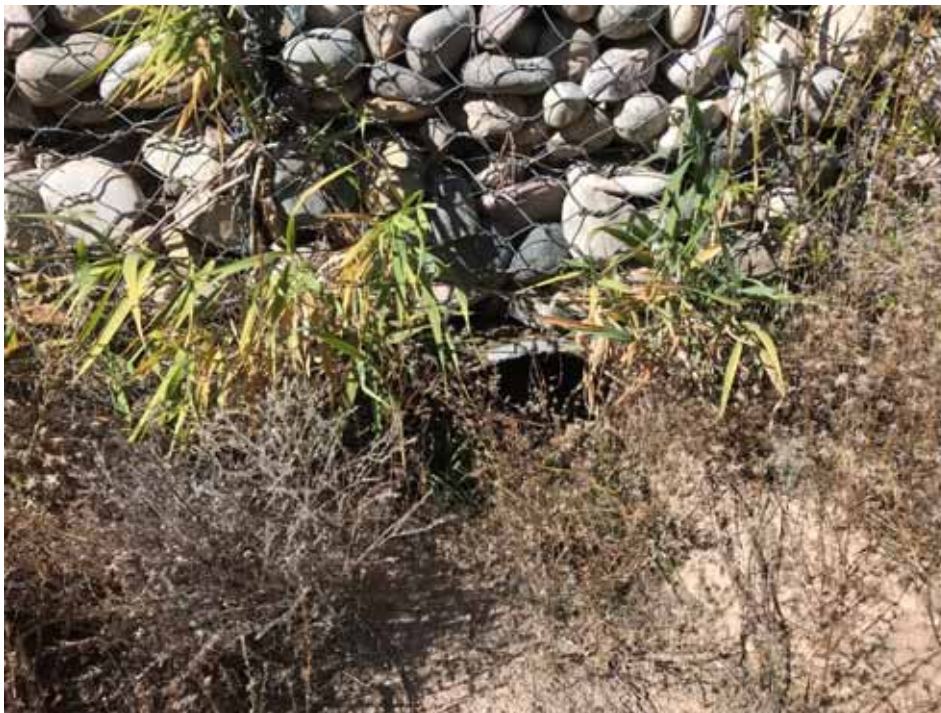
Photo C-5.3-4 October 2022—Outlet is approximately two-thirds below grade and remains functional.
