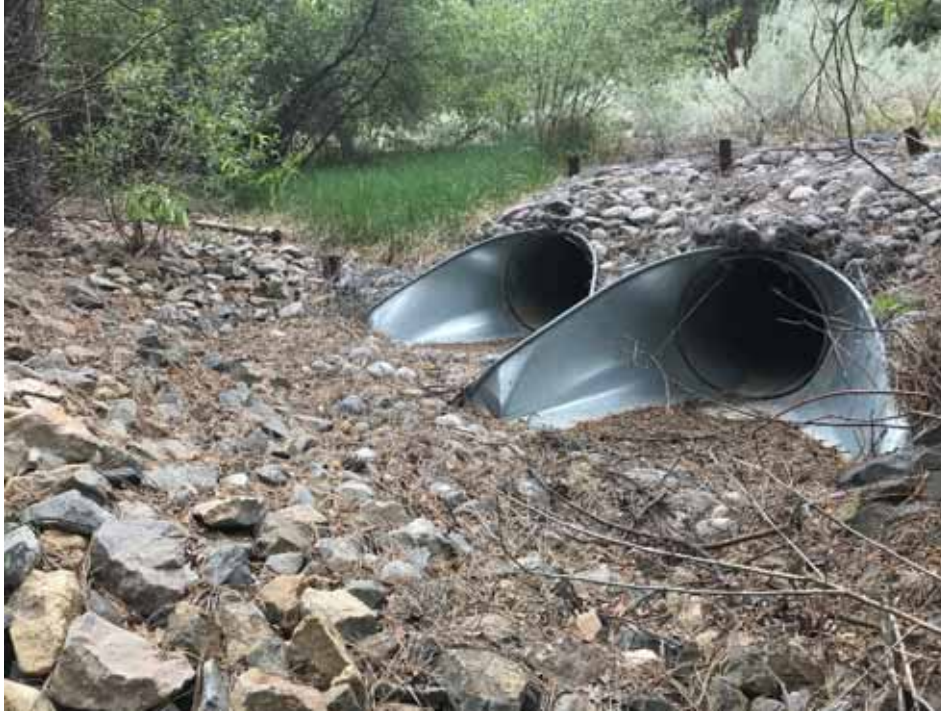
Photo C-3.4-17 May 2022—Discharge culvert outlets and bank protection
