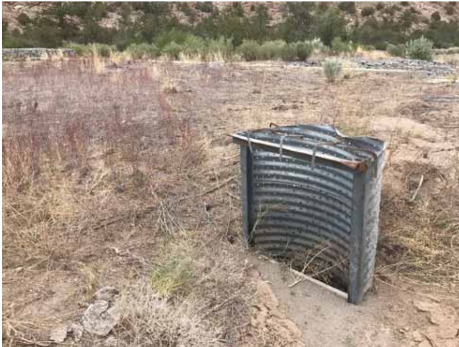
Photo C-5.3-1 May 2022—Outlet culvert standpipe. Outlet is approximately two-thirds below grade and remains functional.
