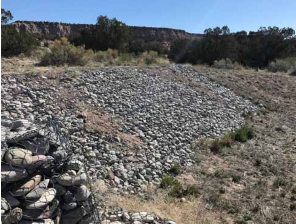
Photo C-4.1-5 May 2022—Downstream northern embankment, looking northeast/downstream. Sediment deposited from runoff coming from dirt roads upgradient of the embankment. No action recommended.
