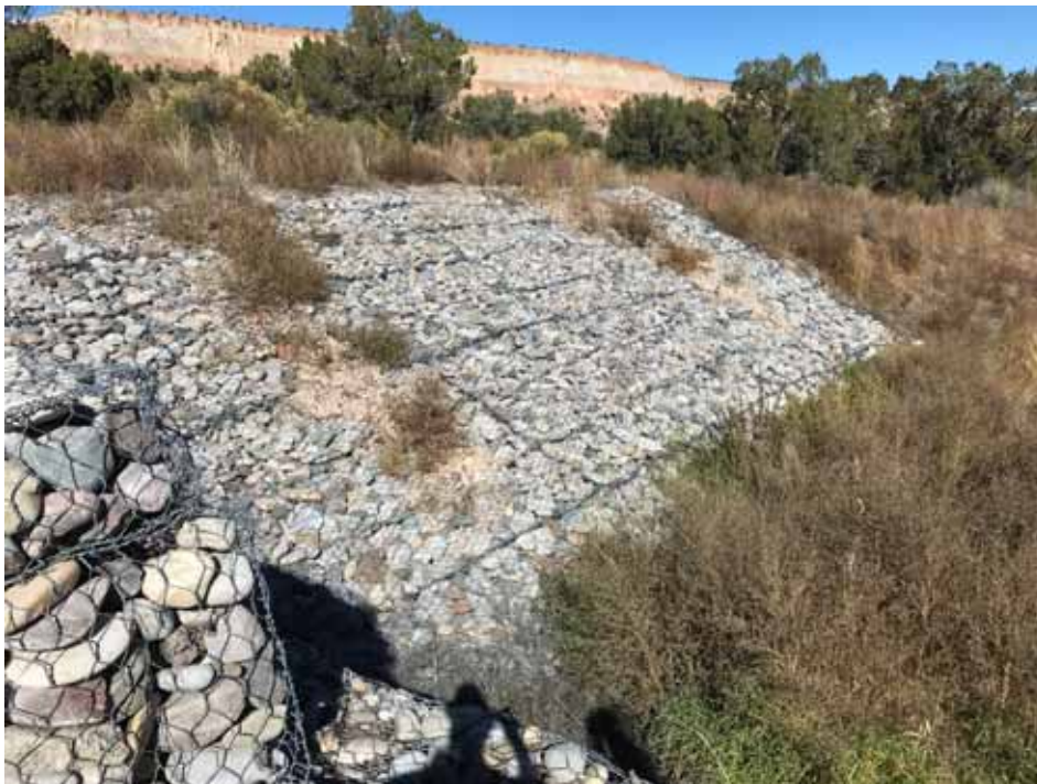
Photo C-4.1-6 October 2022—Downstream northern embankment, looking northeast/downstream. Sediment deposited from runoff coming from dirt roads upgradient of the embankment. No action recommended.
