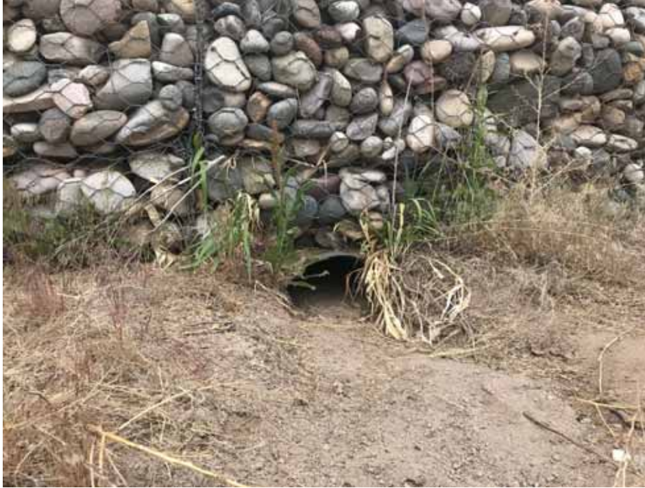
Photo C-5.3-3 October 2022—Outlet is approximately two-thirds below grade and remains functional.
