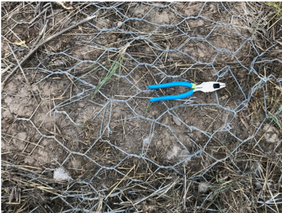
Photo C-4.7-1 October 2022—Hole repaired in gabion
