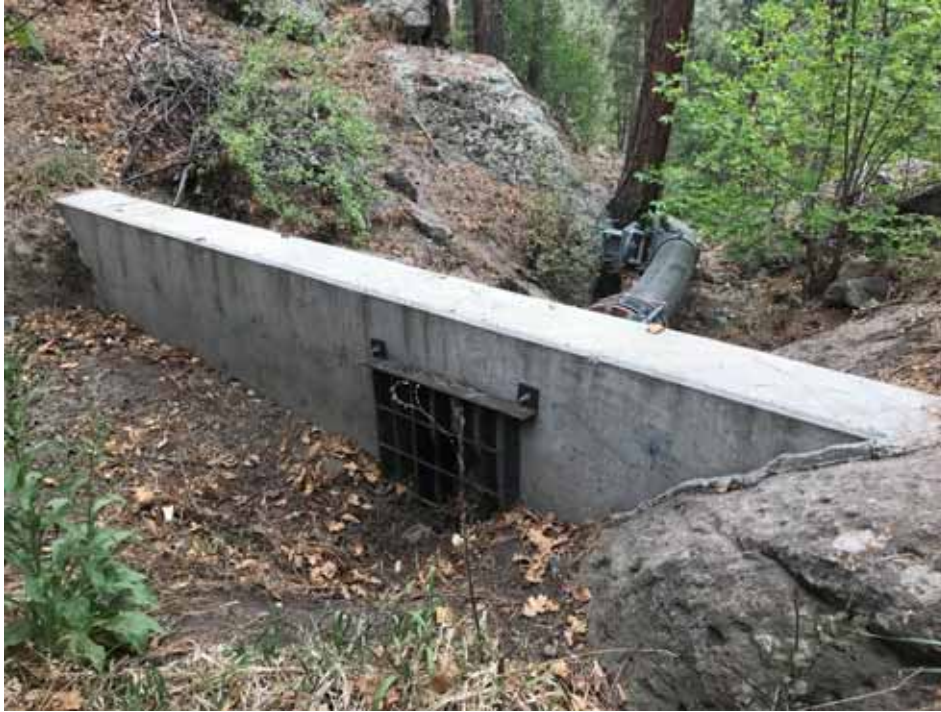
Photo C-3.4-1 May 2022—Pipeline headwall
