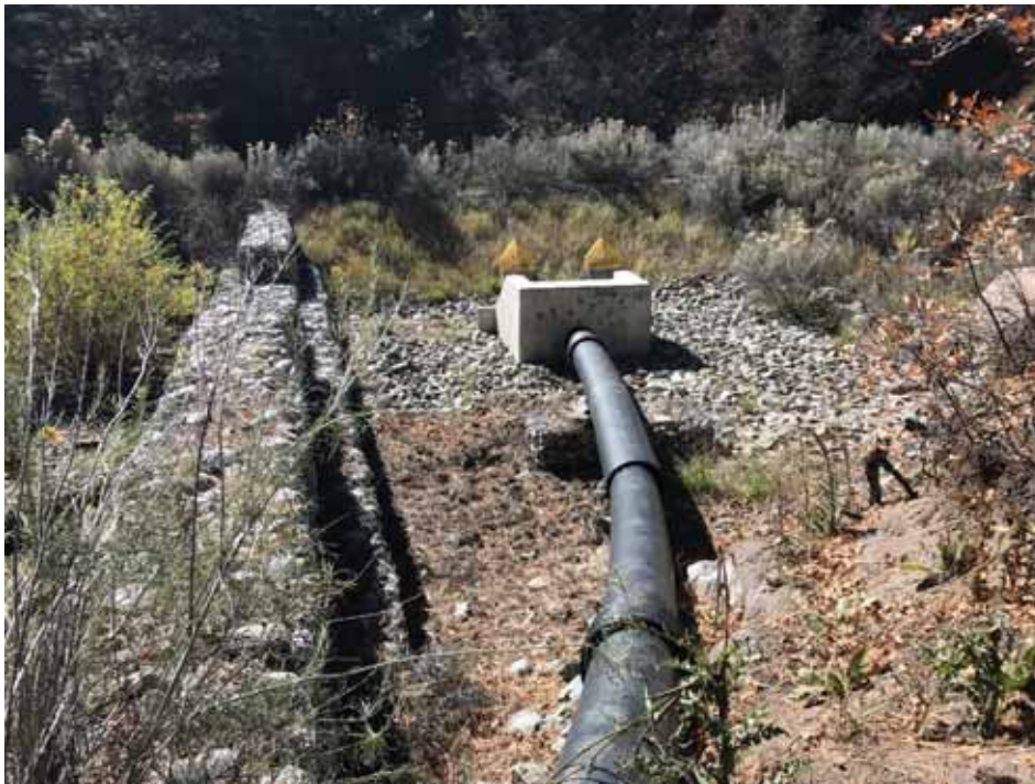
Photo C-3.4-12 October 2022—Pipeline outlet, energy dissipater, and gabion overflow structure
