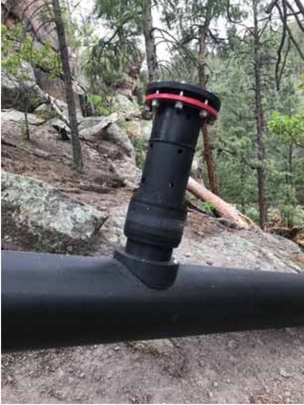
Photo C-3.4-7 May 2022—Pipeline vacuum breaker
