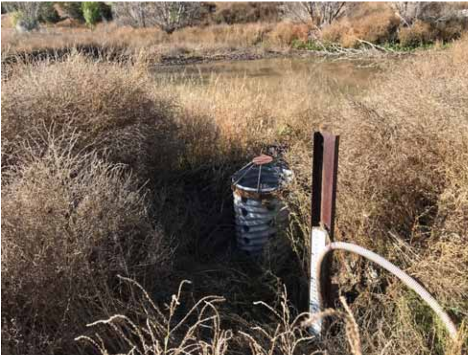
Photo C-4.4-2 October 2022—Standpipe. Debris is at staff plate height 5.4 ft and sediment is at 4.9 ft. No significant change since last inspection.
