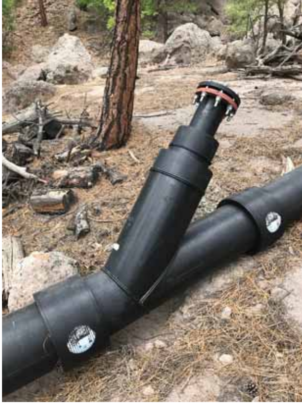
Photo C-3.4-5 May 2022—Pipeline cleanout
