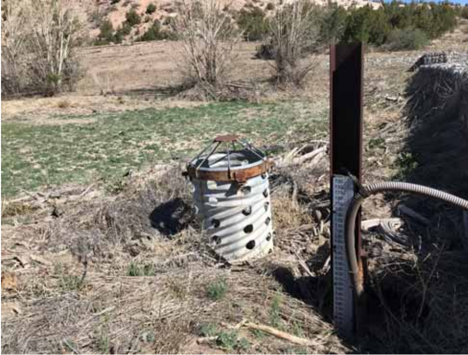
Photo C-4.4-1 May 2022—Standpipe. Debris is at staff plate height 5.1 ft and sediment is at 4.8 ft. No significant change since last inspection.
