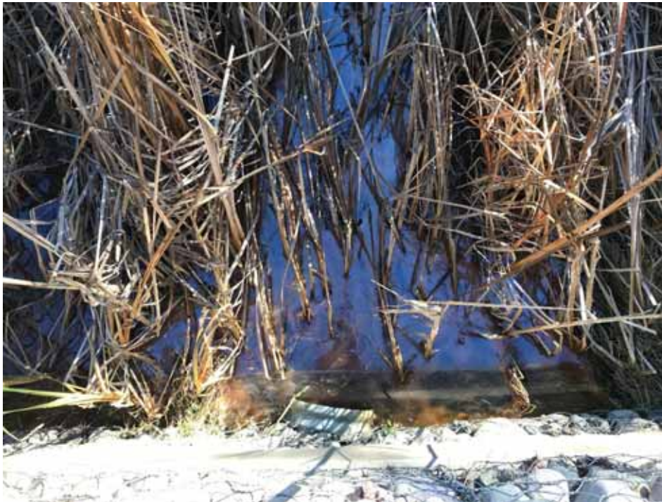
Photo C-2.5-2 October 2022—Outlet. Pond level was above the bottom of the culvert invert at time of inspection.
