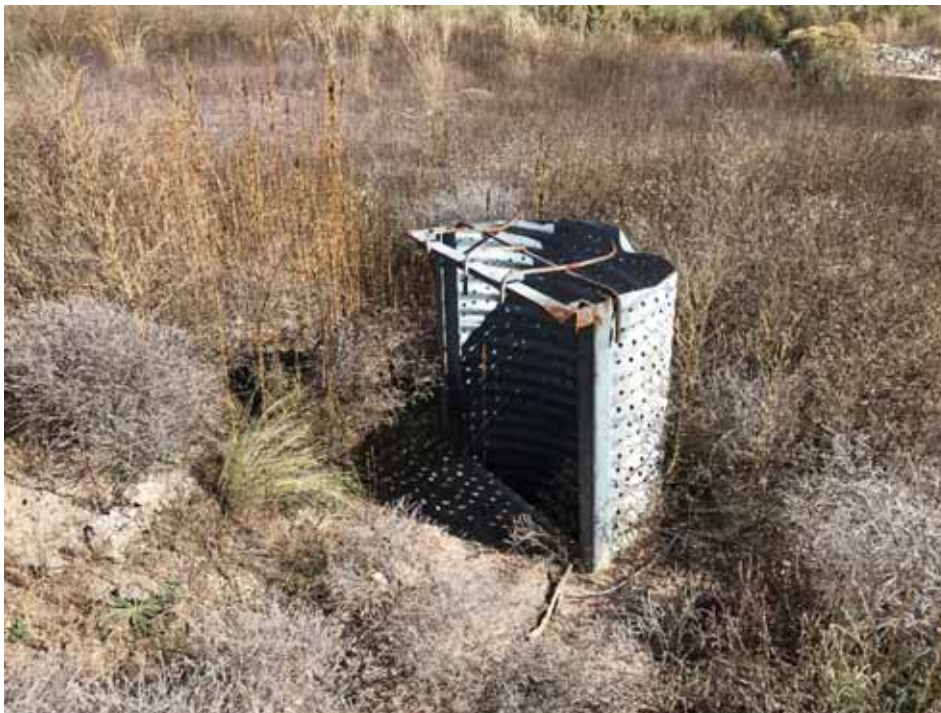
Photo C-5.3-2 October 2022—Outlet culvert standpipe. Outlet is approximately two-thirds below grade and remains functional.
