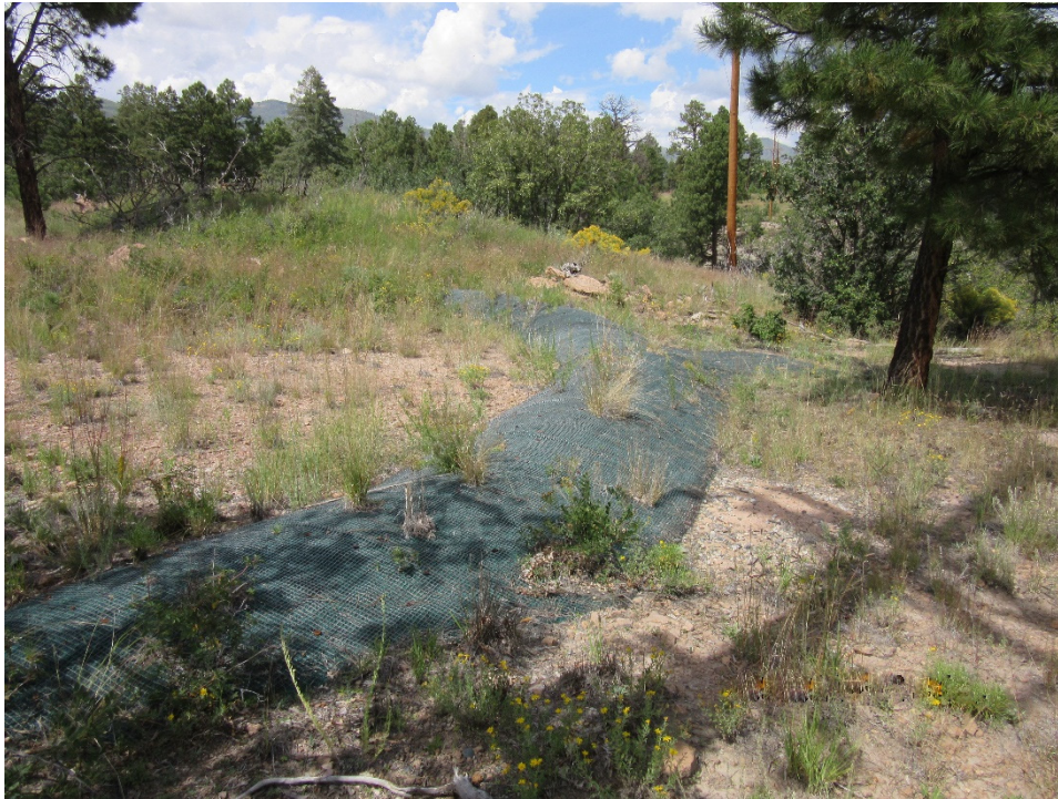
Figure 5 Earthen berm (V00703010027, center of photo) at the top of drainage leading into Fishladder Canyon (September 2022). Note established vegetation. Condition of control: excellent.
