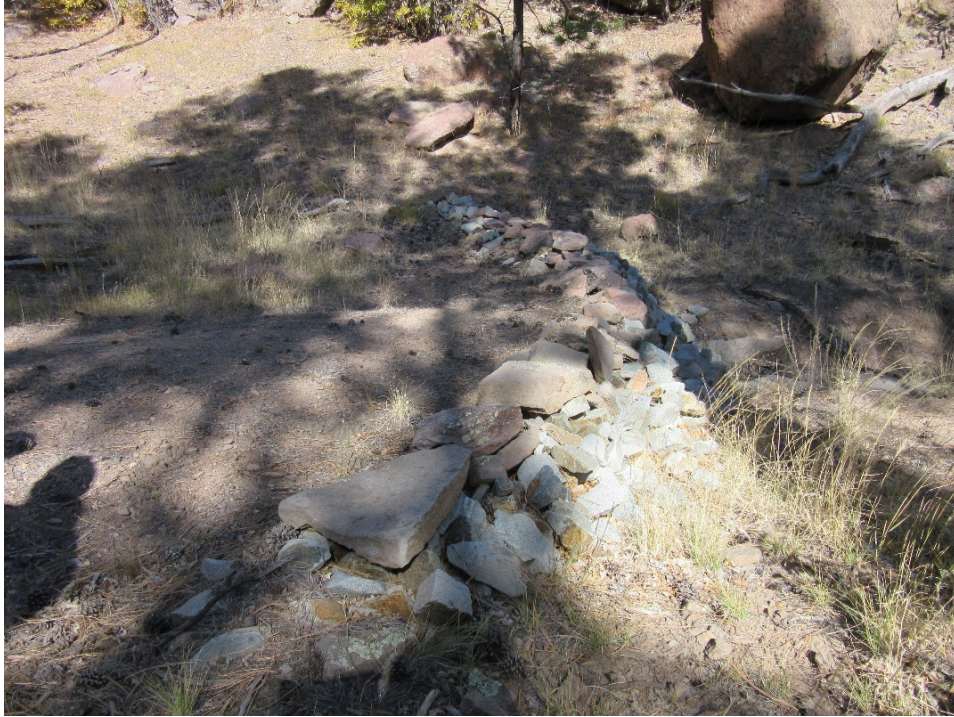
Figure 12 Rock check dam (V00706010024, center of photo) in Fishladder Canyon primary drainage (October 2021). Condition of control: good.
