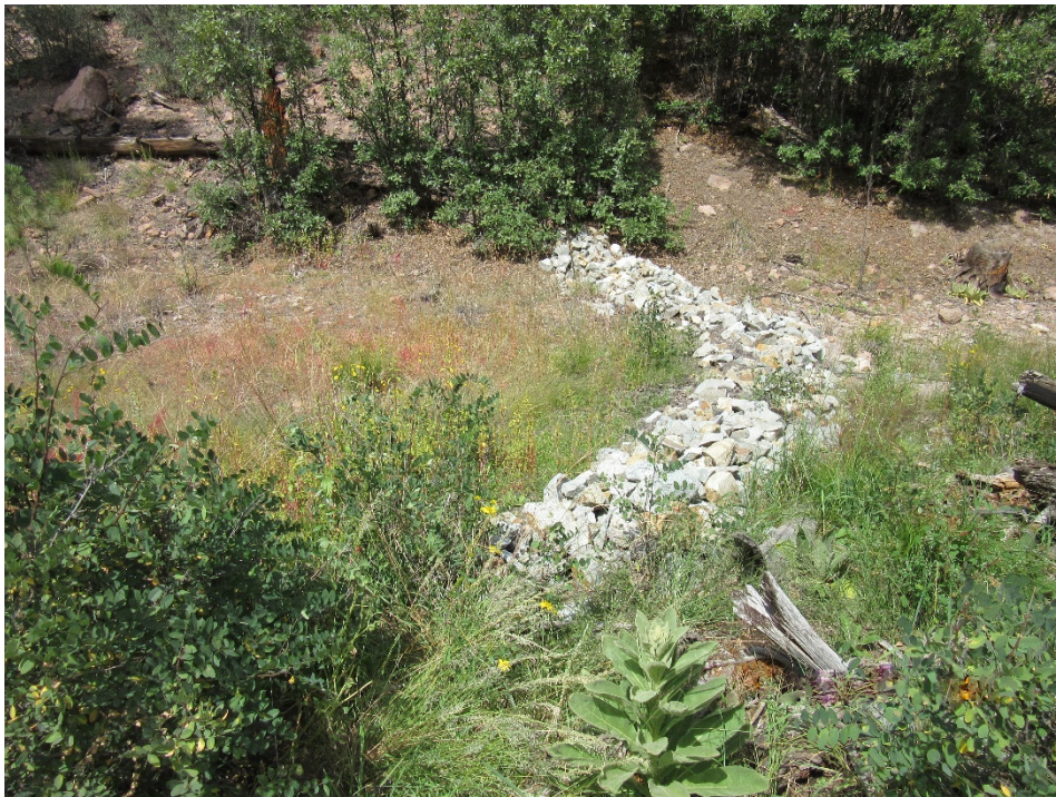
Figure 15 Rock check dam (V00706010025, center of photo) in primary drainage (September 2022). Note established vegetation in channel. Condition of control: excellent.
