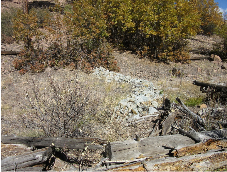
Figure 14 Rock check dam (V00706010025, center of photo) in primary drainage (October 2021). Note established vegetation in channel. Condition of control: excellent.
