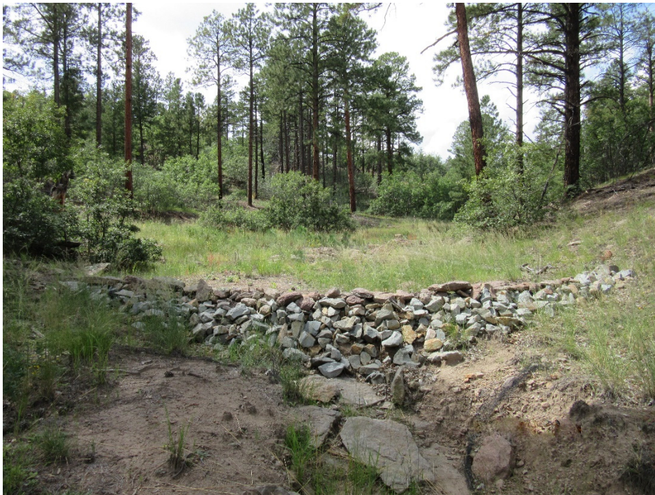
Figure 13 Rock check dam (V00706010024, center of photo) in Fishladder Canyon primary drainage (September 2022). Condition of control: good.
