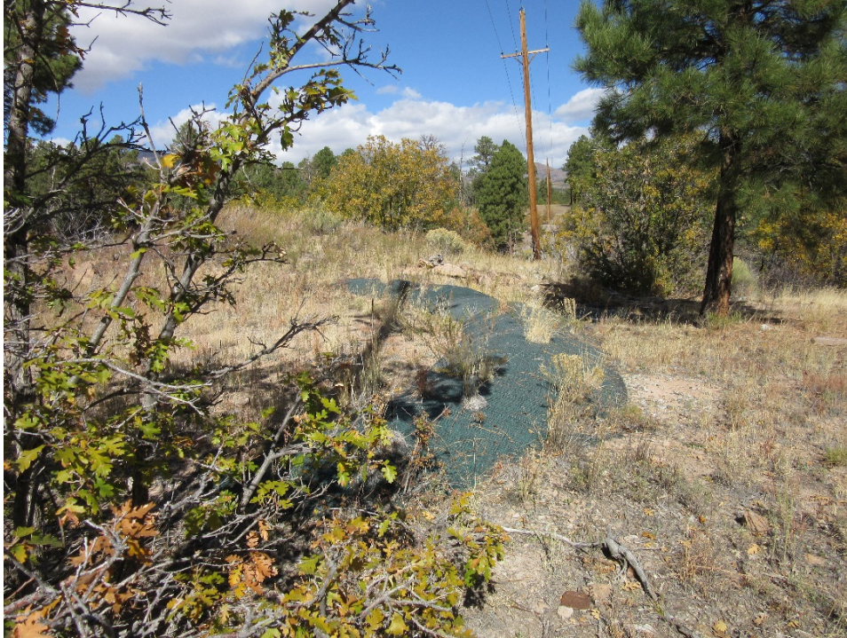
Figure 4 Earthen berm (V00703010027, center of photo) at the top of drainage leading into Fishladder Canyon (October 2021). Note established vegetation. Condition of control: excellent.
