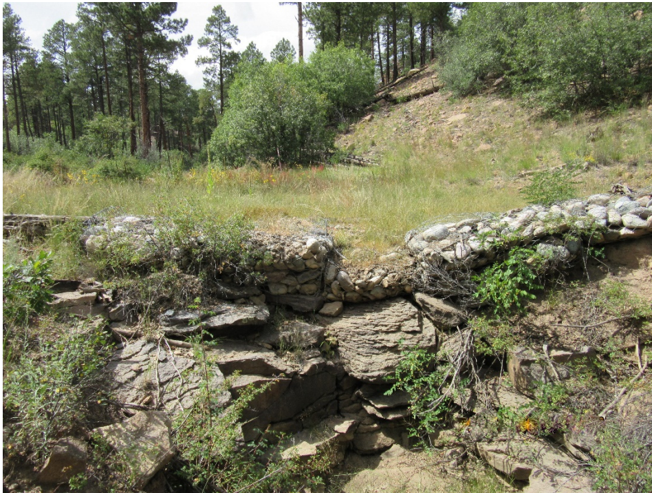
Figure 17 Gabion (V00707010002, center of photo) at access road crossing in Fishladder Canyon (September 2022). Note vegetation in channel upstream of control. Condition of control: good.
