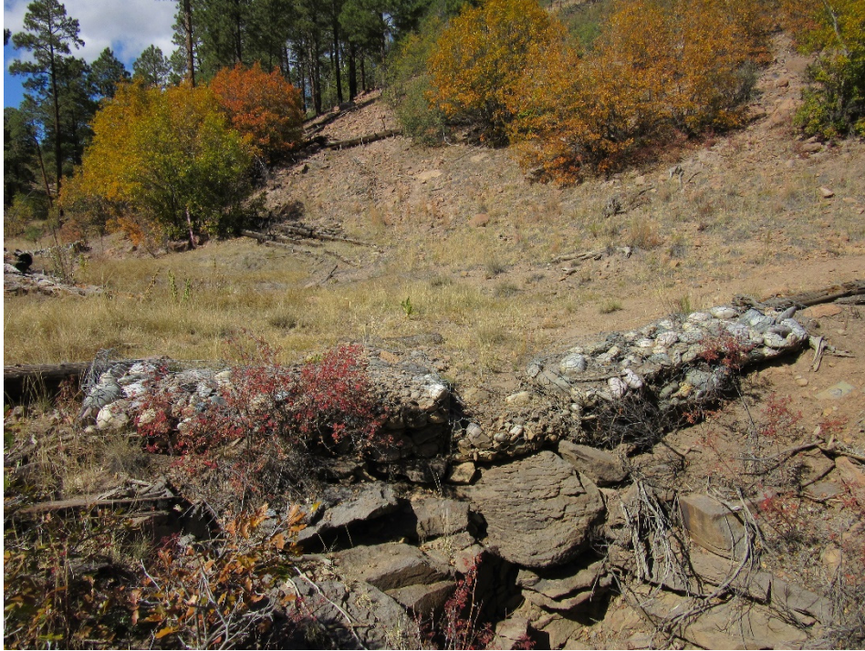
Figure 16 Gabion (V00707010002, center of photo) at access road crossing in Fishladder Canyon (October 2021). Note vegetation in channel upstream of control. Condition of control: good.
