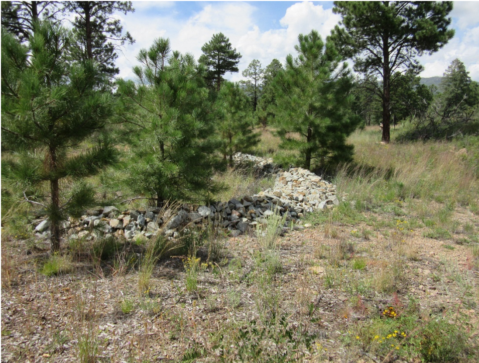
Figure 3 Rock berm (V00703120026, center of photo) at the top of drainage leading into Fishladder Canyon (September 2022). Note established vegetation. Condition of control: excellent.
