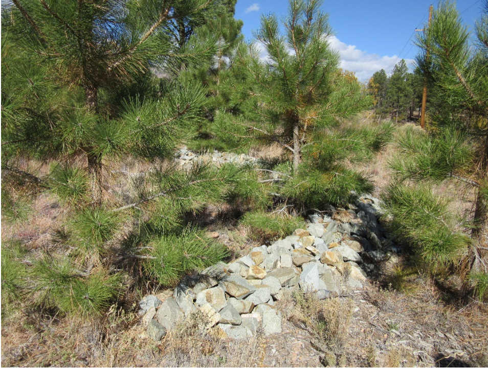
Figure 2 Rock berm (V00703120026, center of photo) at the top of drainage leading into Fishladder Canyon (October 2021). Note established vegetation. Condition of control: excellent.
