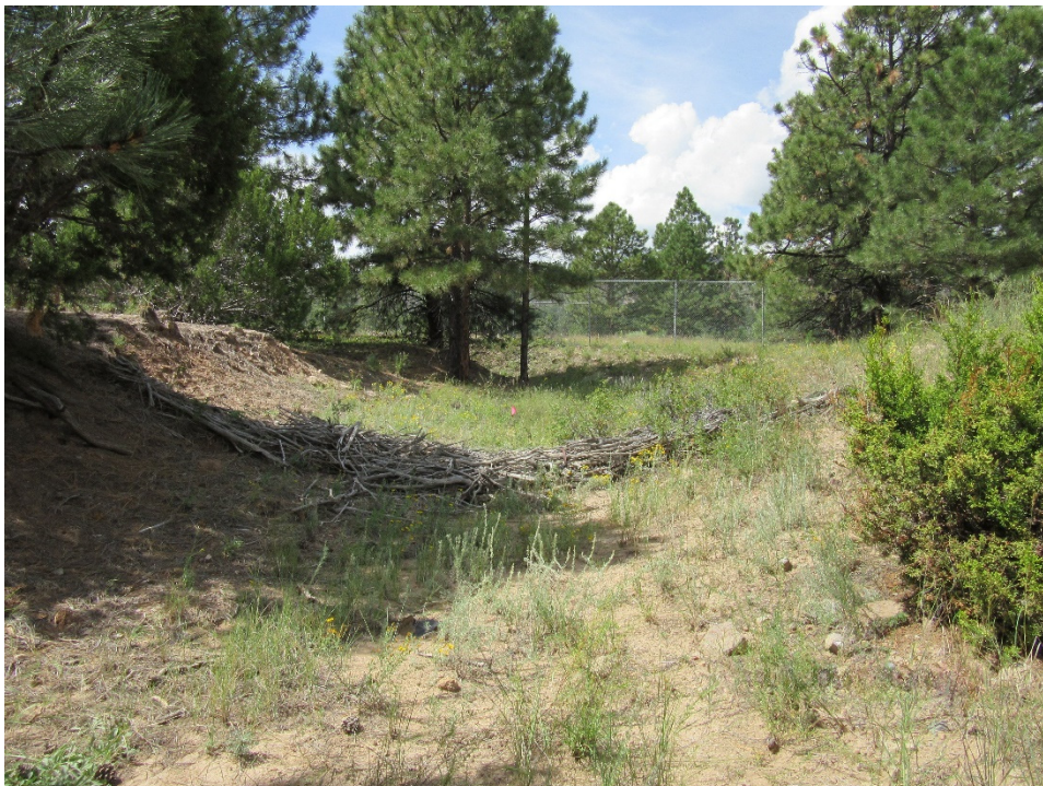
Figure 8 Juniper bale check dam located in drainage channel to 90s Line Pond, September 2022. Note vegetation in channel.
