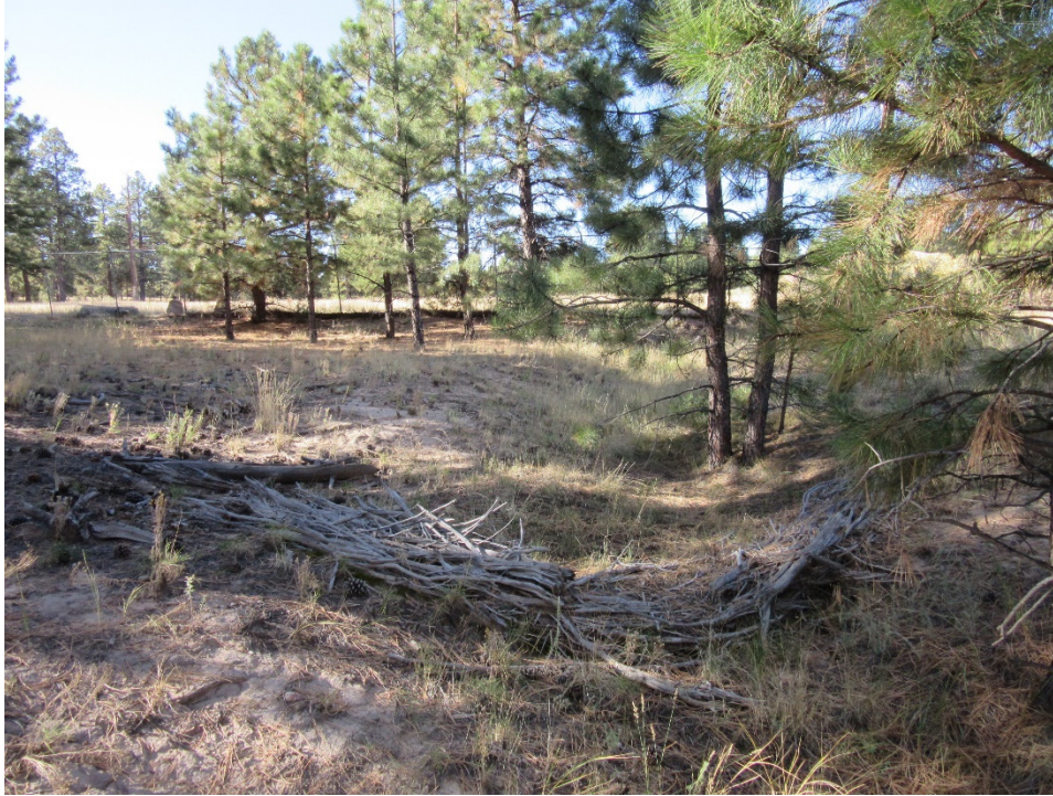
Figure 9 Juniper bale check dam located in drainage channel to 90s Line Pond, October 2021. Note vegetation in channel.
