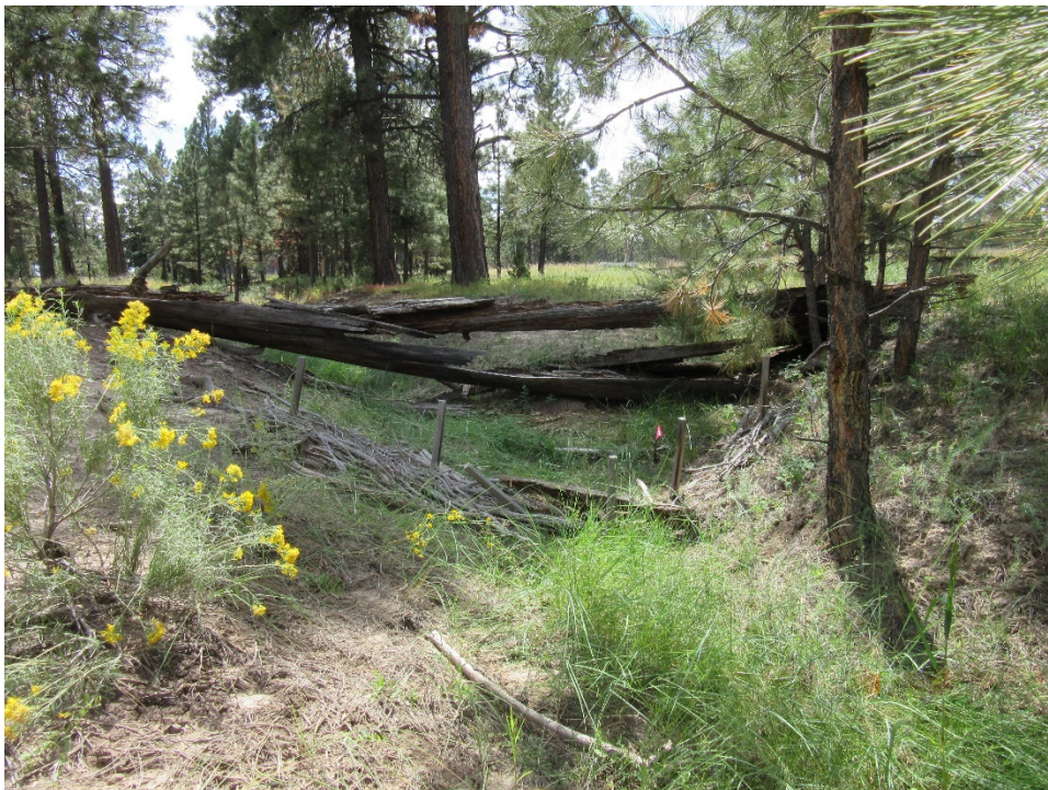
Figure 12 Juniper bale check dam located in drainage channel to 90s Line Pond, September 2022. Note vegetation in channel.
