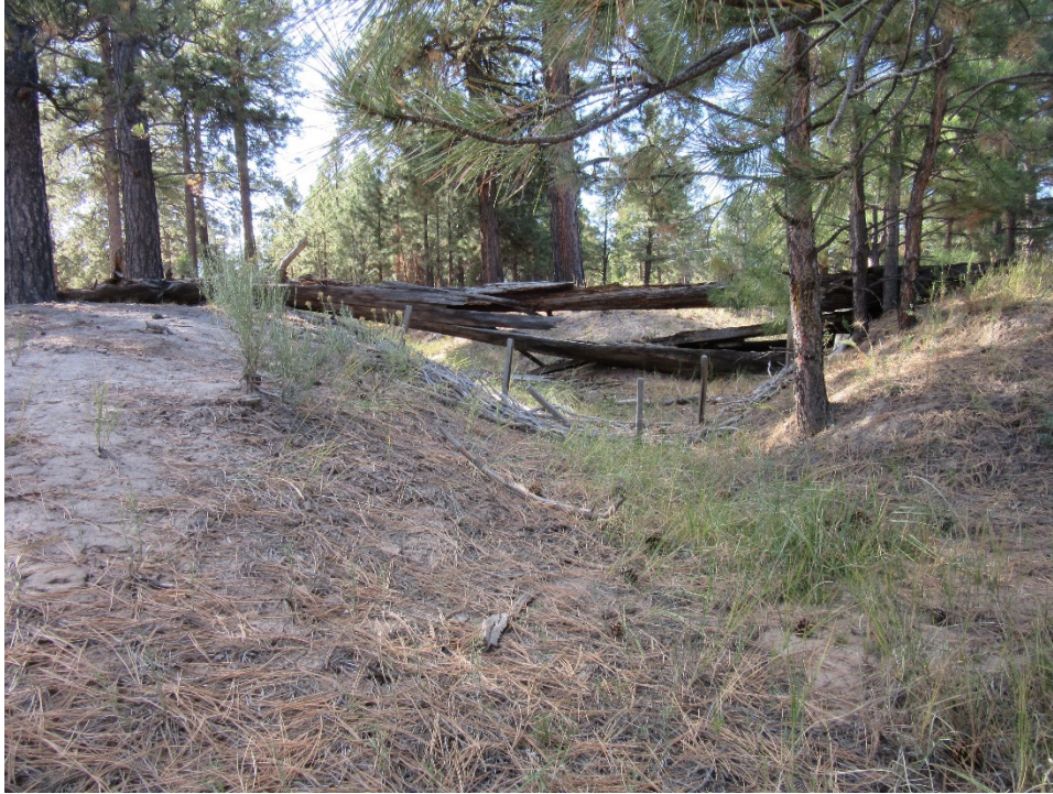
Figure 11 Juniper bale check dam located in drainage channel to 90s Line Pond, October 2021. Note vegetation in channel.
