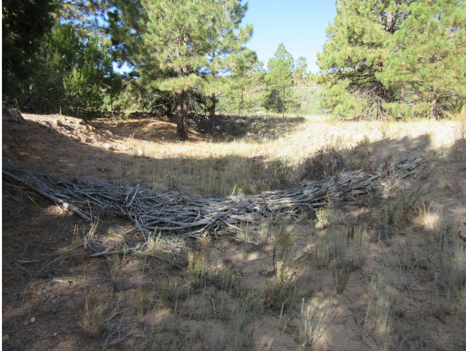
Figure 7 Juniper bale check dam located in drainage channel to 90s Line Pond, October 2021. Note vegetation in channel.
