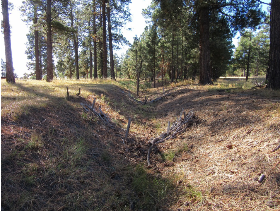
Figure 5 Juniper bale check dams located in drainage channel to 90s Line Pond, October 2021. Note vegetation in channel.
