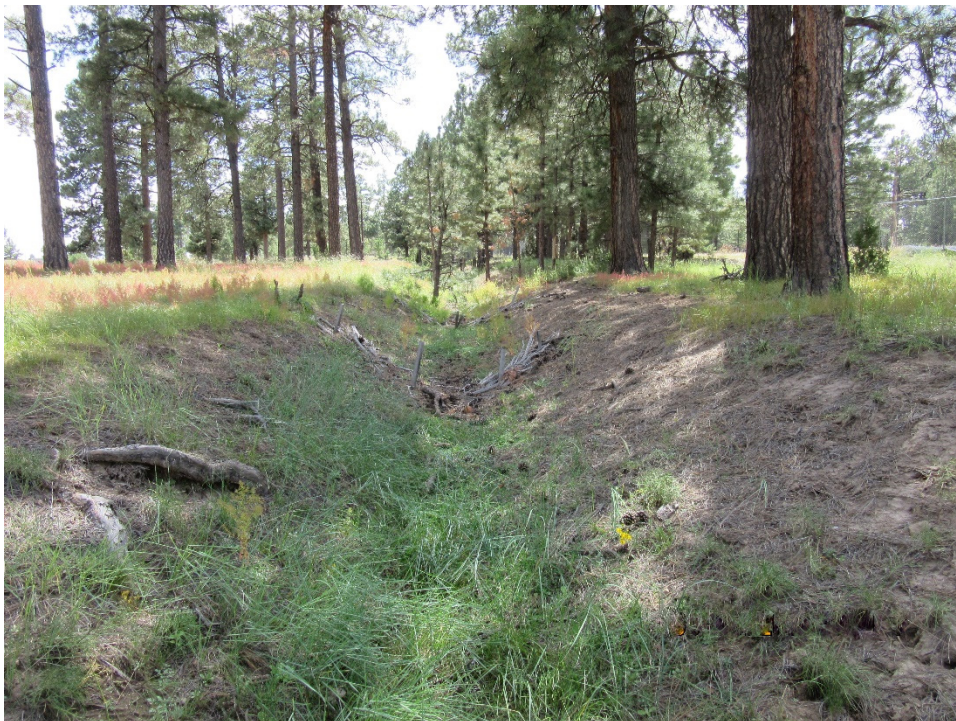
Figure 6 Juniper bale check dams located in drainage channel to 90s Line Pond, September 2022. Note vegetation in channel.
