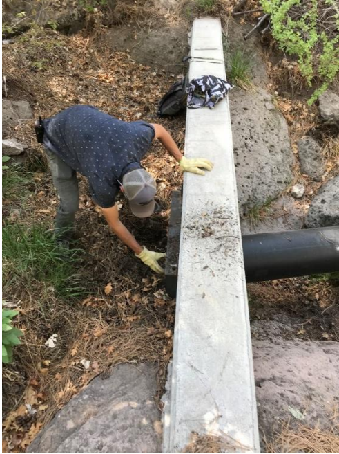
Photo C-3.4-1 May 2021—Pipeline headwall. Needlecast blockage removed.
