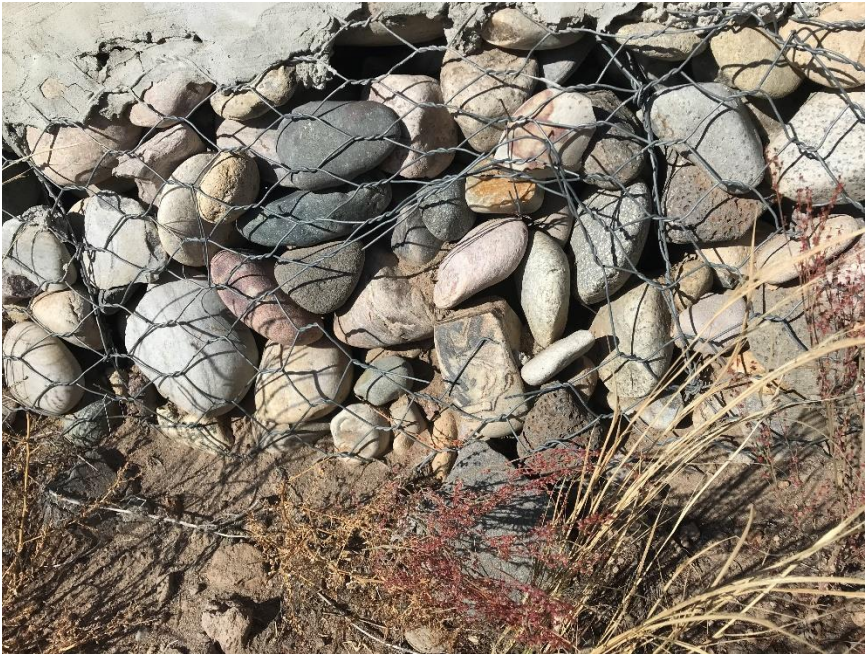
Photo C-5.5-1 October 2021—Identified broken wire in gabions at weir. Maintenance will be done during spring 2022 inspection.
