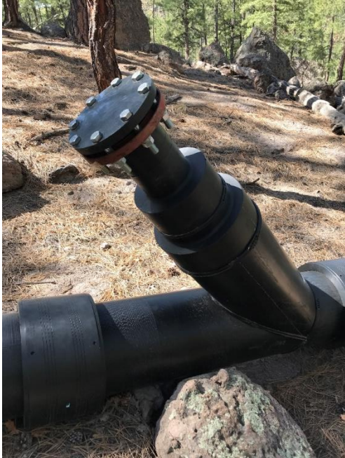
Photo C-3.4-7 May 2021—Pipeline cleanout
