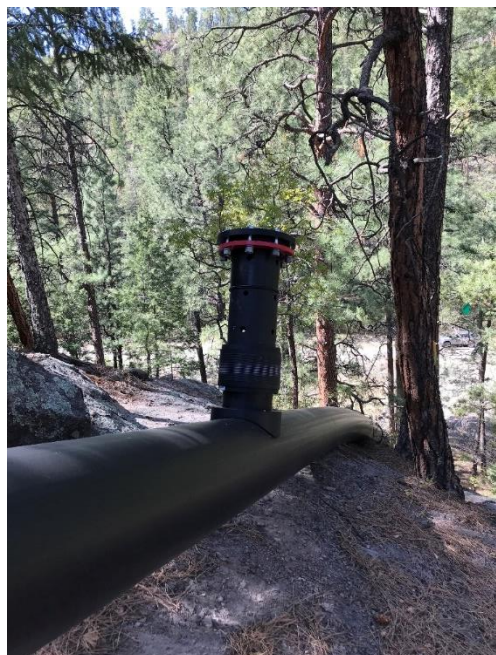
Photo C-3.4-9 May 2021—Pipeline vacuum breaker
