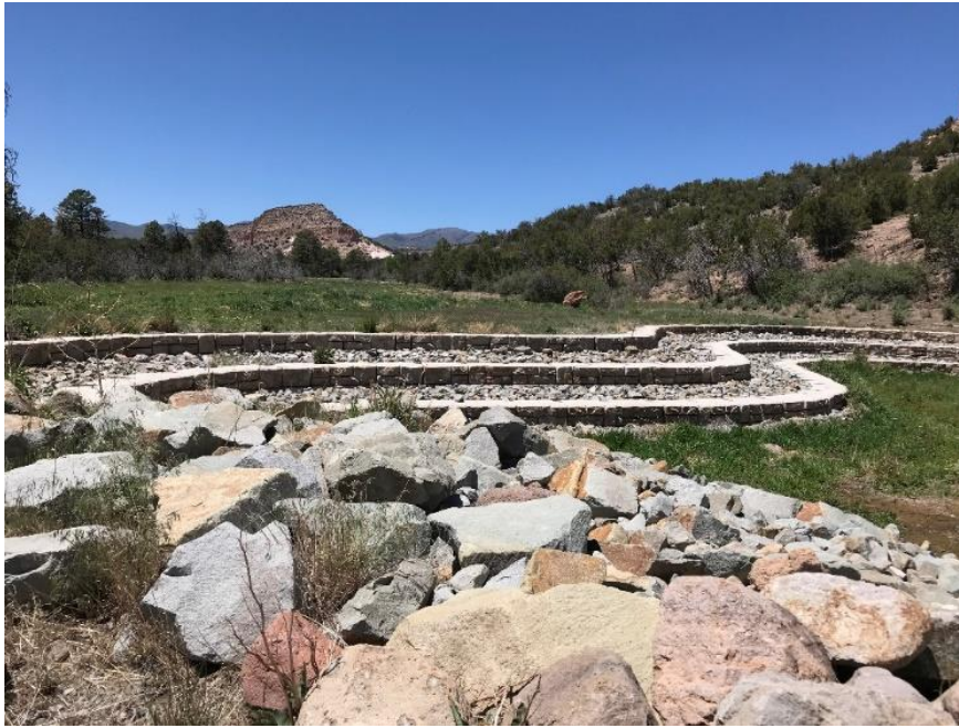
Photo C-6.1-1 May 2021—Redi-Rock block structure, looking west/upstream
