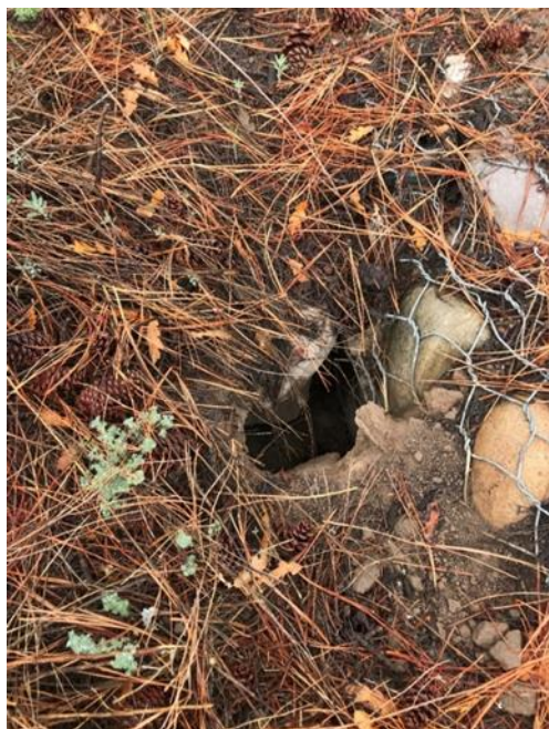
Photo C-2.6-2 May 2021—Filled piping hole with riprap.
