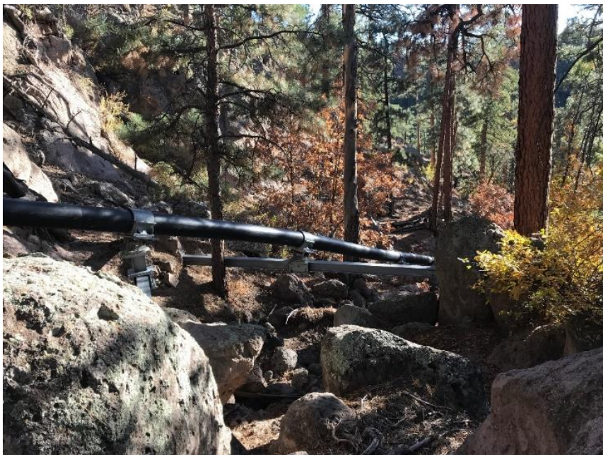
Photo C-3.4-6 October 2021—Pipeline beam supports
