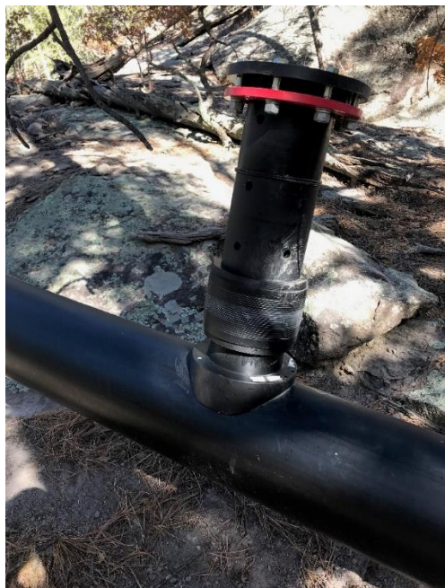
Photo C-3.4-10 October 2021—Pipeline vacuum breaker
