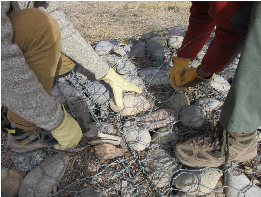
Photo C-4.7-1 May 2021—Repair of holes in gabion baskets noted in earlier inspections. Trash was also picked up from weir ponding area.
