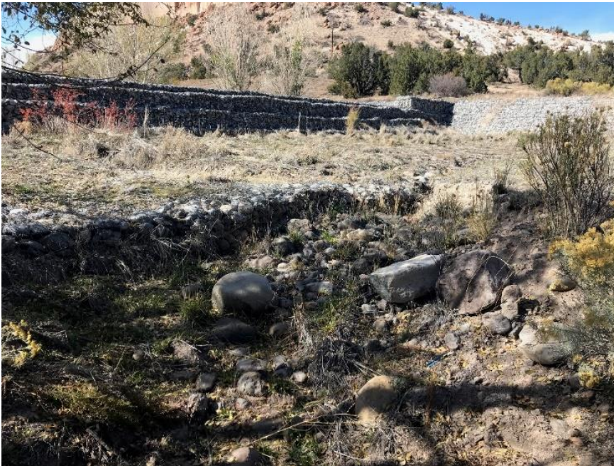
Photo C-4.5-4 October 2021—Headcut at edge of gabion mattress, downstream of weir outlet, looking west/upstream. Continue to monitor.
