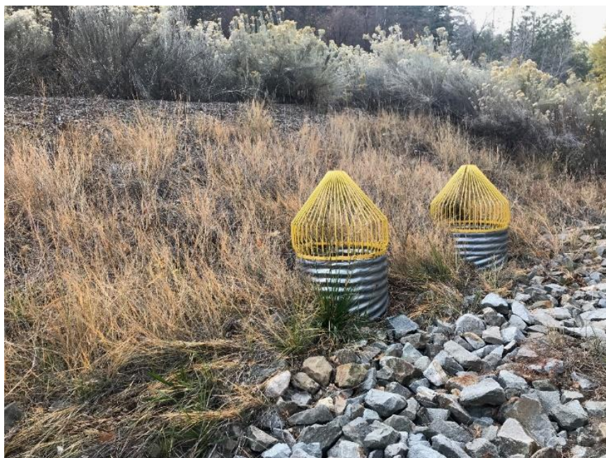
Photo C-3.4-18 October 2021—Discharge culvert inlets and trash racks
