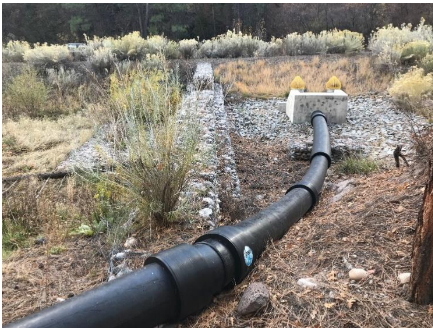
Photo C-3.4-14 October 2021—Pipeline outlet, energy dissipater, and gabion overflow structure
