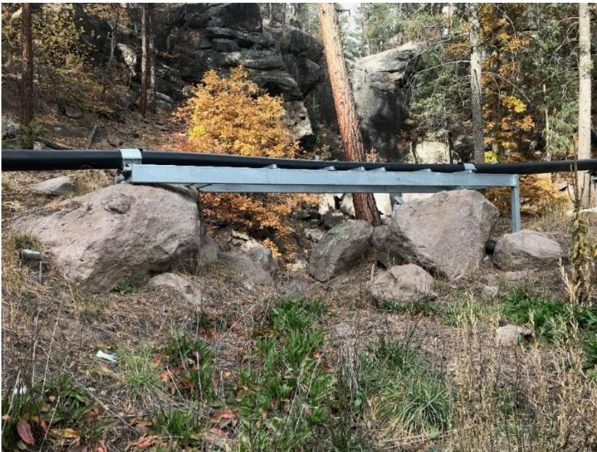
Photo C-3.4-12 October 2021—Pipeline bridge structure
