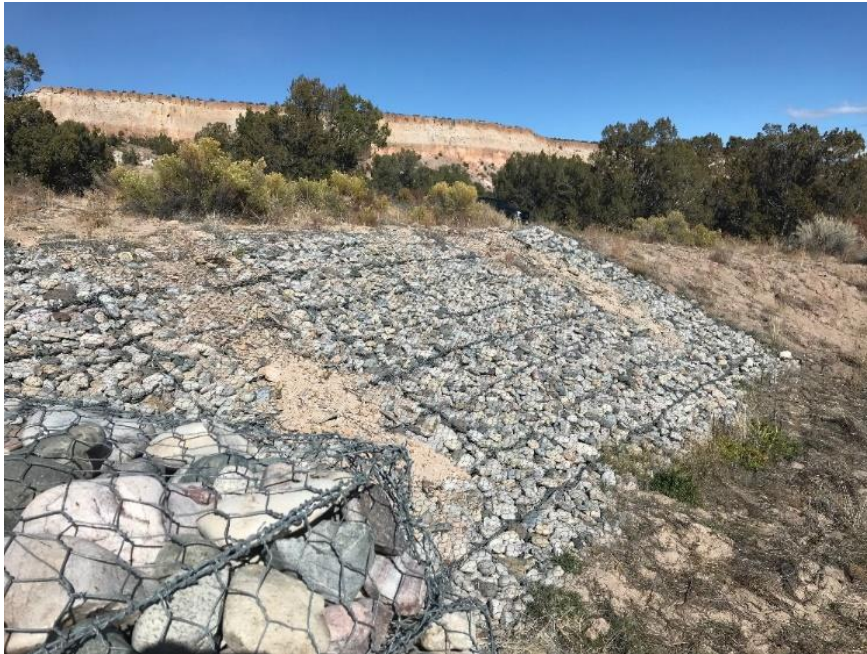
Photo C-4.1-6 October 2021—Downstream northern embankment, looking east/downstream. Sediment deposited from runoff coming from dirt roads upgradient of the embankment. No action recommended.
