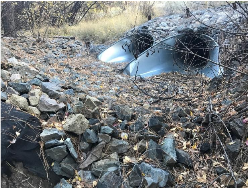
Photo C-3.4-20 October 2021—Discharge culvert outlets and bank protection
