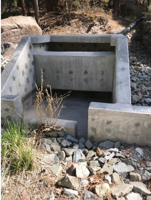
Photo C-3.4-15 May 2021—Pipeline energy dissipater
