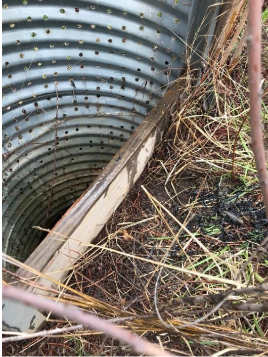
Photo C-2.3-1 May 2021—Standpipe. Sediment level is approximately 1 ft below wood stop board. No significant change since last inspection. Continue to monitor.
