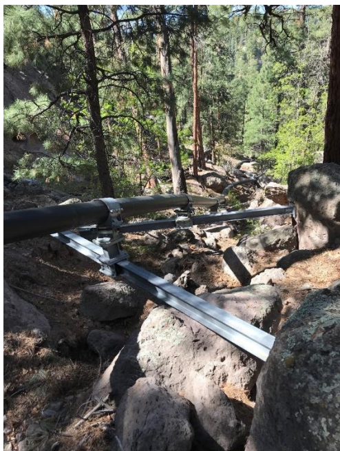
Photo C-3.4-5 May 2021—Pipeline beam supports
