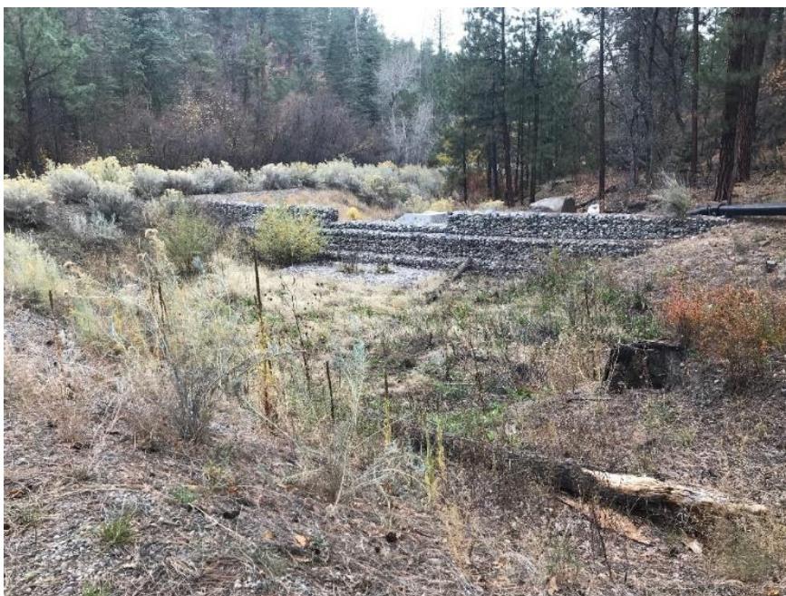
Photo C-3.1-4 October 2021—Upper basin, looking southwest at gabion overflow structure
