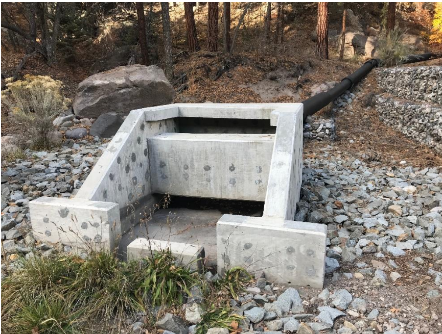
Photo C-3.4-16 October 2021—Pipeline energy dissipater
