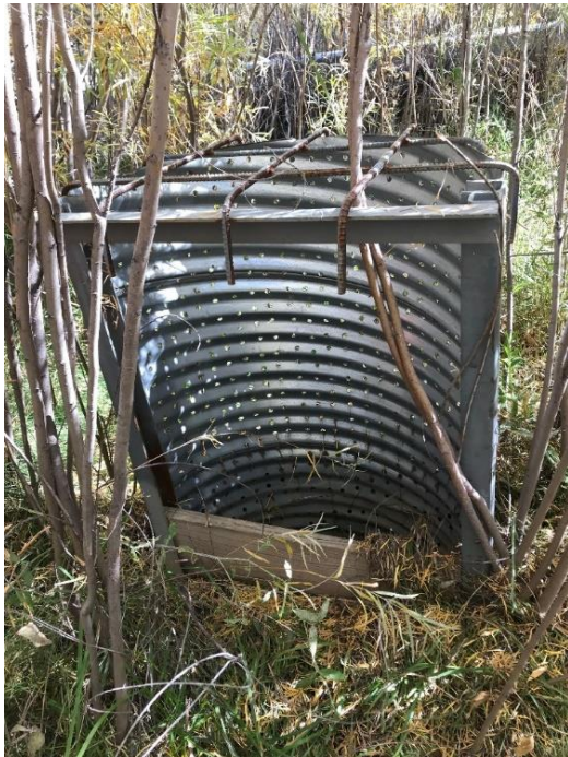
Photo C-2.3-2 October 2021—Standpipe. Sediment level is approximately 1 ft below wood stop board. No significant change since last inspection. Continue to monitor.
