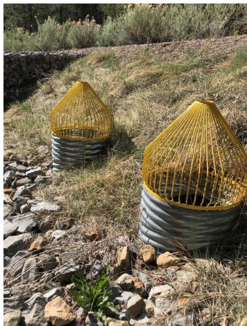
Photo C-3.4-17 May 2021—Discharge culvert inlets and trash racks
