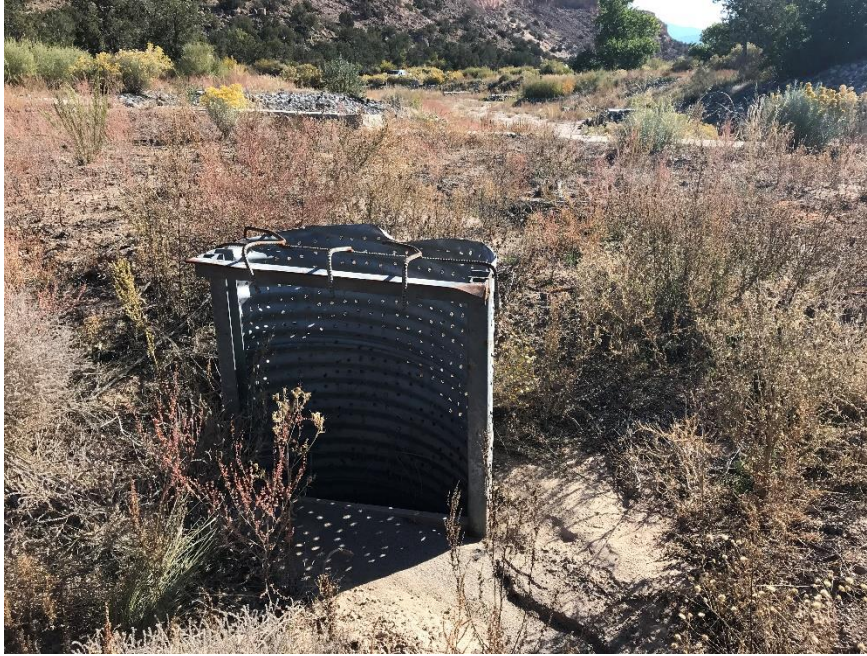
Photo C-5.3-1 October 2021—Outlet culvert standpipe. Outlet is approximately two-thirds belowgrade and remains functional.
