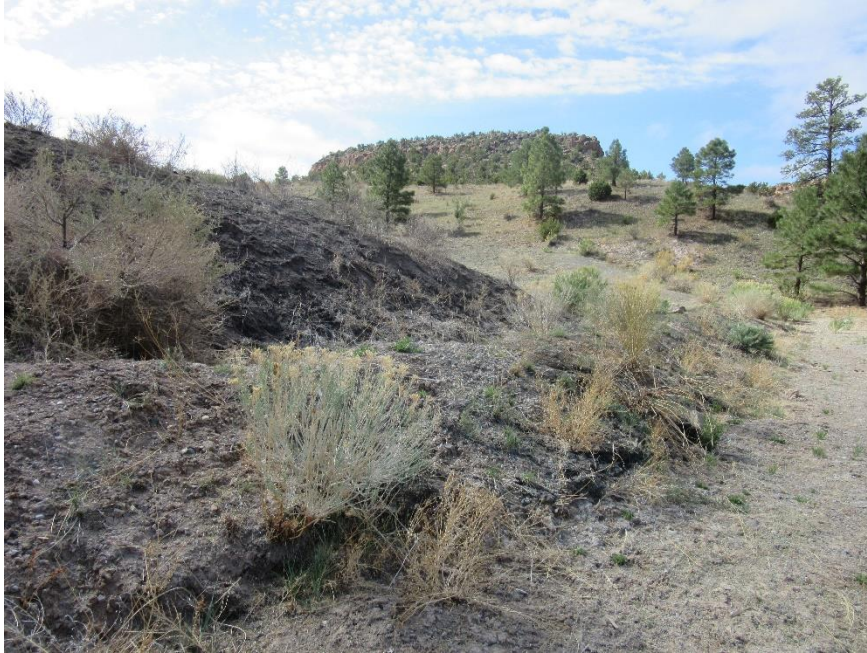
Photo C-4.6-3 May 2021—Borrow pit runoff retention berm. Berm has been impacted by recent Los Alamos County well construction activities. Berm is still functioning and stable, no action recommended. Continue to monitor.
