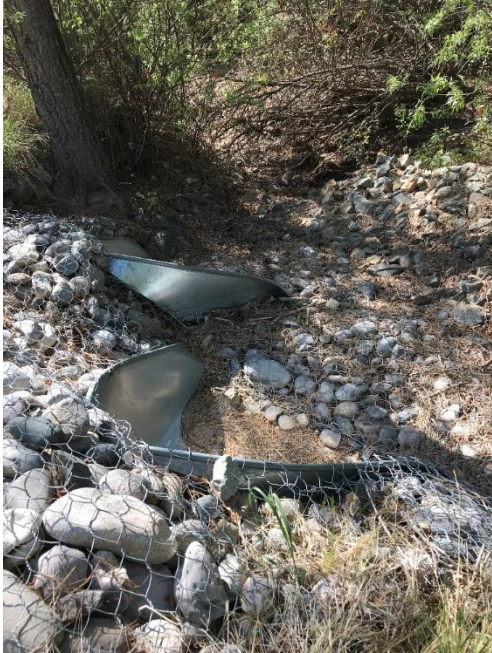
Photo C-3.4-19 May 2021—Discharge culvert outlets and bank protection
