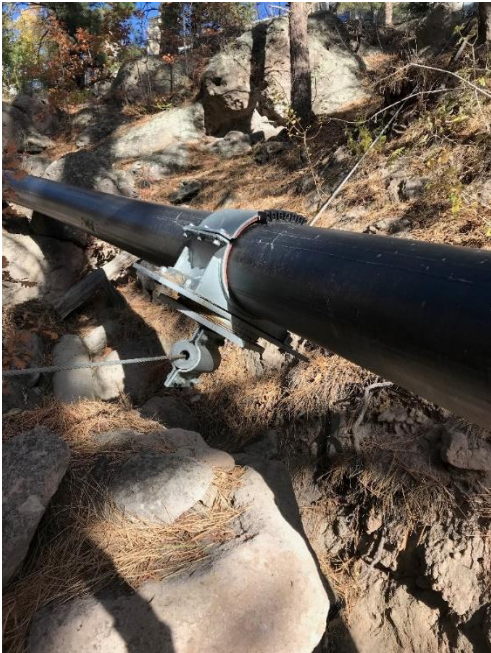
Photo C-3.4-4 October 2021—Pipeline cable support
