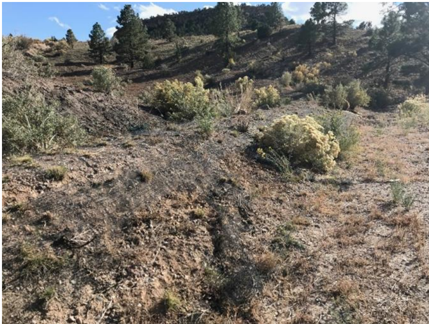
Photo C-4.6-4 October 2021—Borrow pit runoff retention berm. Berm has been impacted by recent Los Alamos County well construction activities. Berm is still functioning and stable, no action recommended. Continue to monitor.
