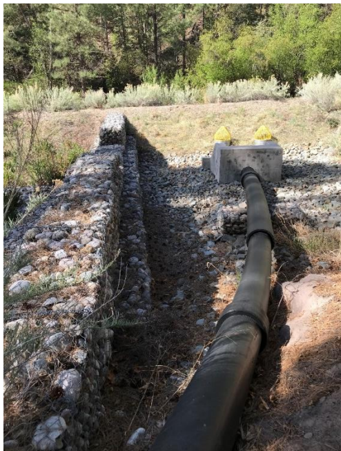
Photo C-3.4-13 May 2021—Pipeline outlet, energy dissipater, and gabion overflow structure
