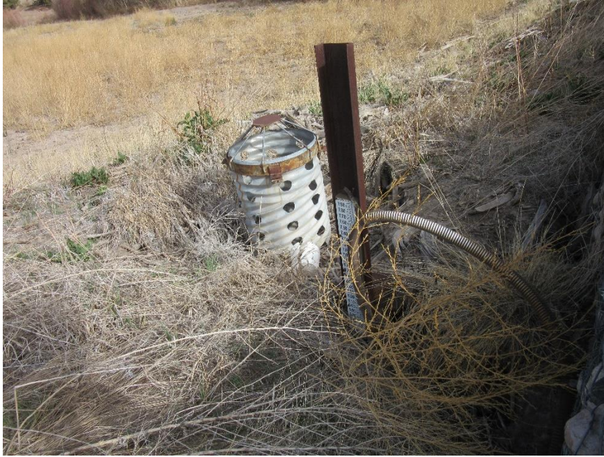
Photo C-4.4-1 May 2021—Standpipe. Debris and sediment is at staff plate height 5.4 ft. No significant change since last inspection.
