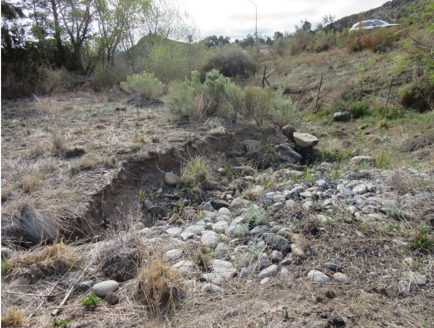
Photo C-4.5-3 October 2021—Headcut at edge of gabion mattress, downstream of weir outlet, looking east/downstream. Continue to monitor.
