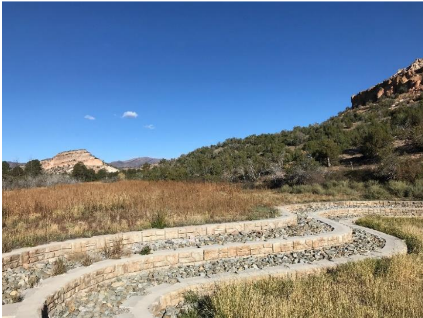
Photo C-6.1-2 October 2021—Redi-Rock block structure, looking west/upstream
