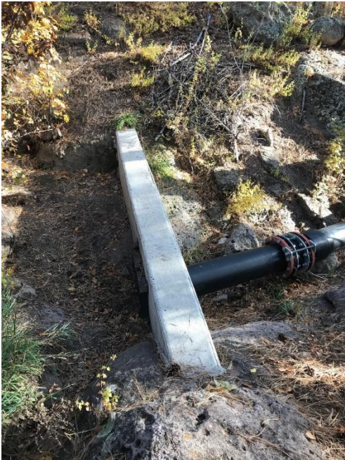
Photo C-3.4-2 October 2021—Pipeline headwall
