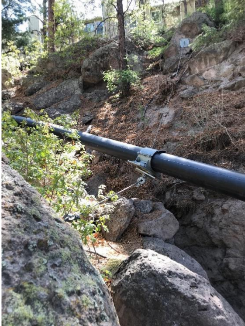
Photo C-3.4-3 May 2021—Pipeline cable support
