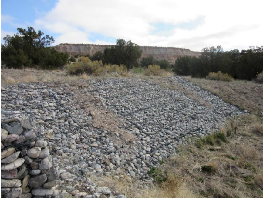
Photo C-4.1-5 May 2021—Downstream northern embankment, looking east/downstream. Sediment deposited from runoff coming from dirt roads upgradient of the embankment. No action recommended.
