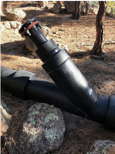
Photo C-3.4-8 October 2021— Pipeline cleanout
