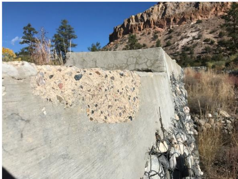
Photo C-5.2-6 October 2021—Spalling on concrete weir spillway. No action recommended, continue to monitor.
