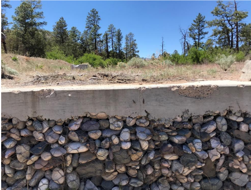
Photo C-5.2-5 May 2021—Spalling on concrete weir spillway. No action recommended, continue to monitor.
