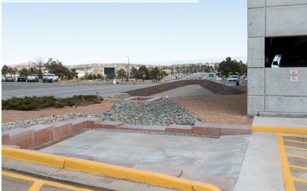
Sediment trap and detention basin to collect parking lot flow at TA-03
