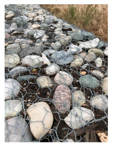
Photo C-4.7-4 September 2020—broken gabion wires on south end of weir crest. Recommend repair.
