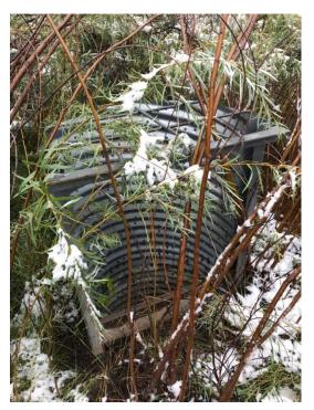
Photo C-2.5-1 September 2020—standpipe. Sediment level is approximately 1 ft below wood board stop. No significant change since last inspection. Will continue to monitor.
