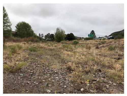
Photo C-4.5-1 September 2020—Los Alamos Pond 2 (middle) looking downstream. Pond has been breached and has no sediment capacity. No action recommended.
