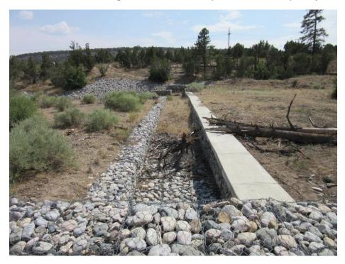
Photo C-5.4-2 August 2020—weir crest and flow-way, looking south. Tree has fallen over overflow weir structure. Recommend removal of tree.
