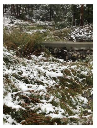
Photo C-2.2-1 September 2020—upslope face of weir, looking east. Weir is functioning; no deteriorating joints or bulging gabion baskets.
