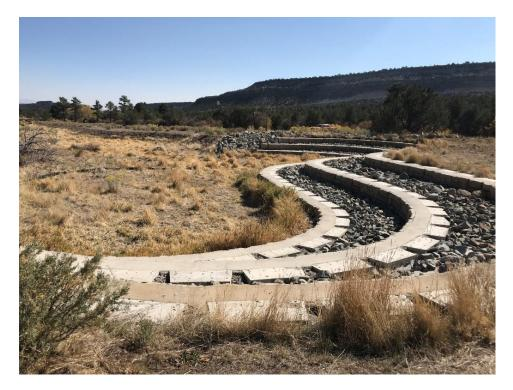
Photo C-6.1-5 October 2020—Redi-Rock block structure, looking southeast. No deficiency found.
