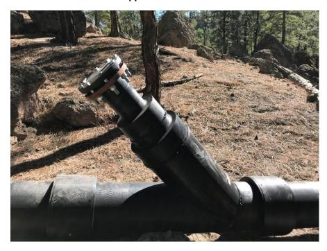
Photo C-3.7-2 October 2020—pipeline vacuum breaker. Control is operating as designed with no apparent issues to structure.
