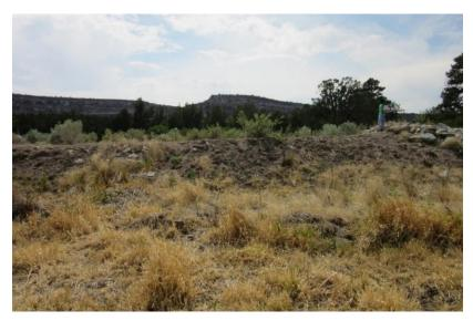
Photo C-6.3-1 August 2020—south bank, looking south. Riprap (Class B) has fallen down to toe of steep slope on south bank. South bank is susceptible to erosion. Loose soil in voids where riprap was placed. Recommend placement of jute erosion-control matting, wire-enclosed riprap using on-site riprap, or brush barriers using on-site fallen trees to stabilize soil on steep slopes downstream of grade-control structure. Continue to monitor.
