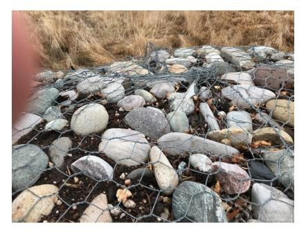
Photo C-4.7-3 September 2020—broken gabions on north end of crest. Recommend repair of holes in gabion basket.
