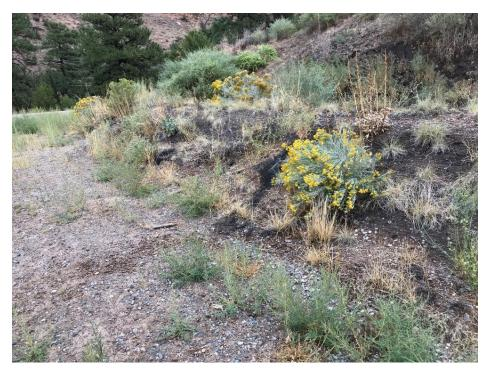
Photo C-4.11-2 September 2020—vegetation on earthen berm. Vegetation is not well established. Continue to monitor. Damage to north end of berm that occurred during county construction remains. No action recommended.
