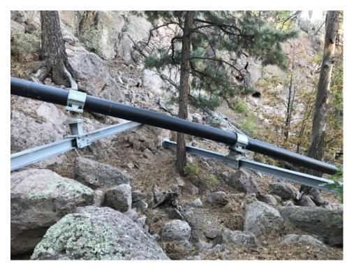
Photo C-3.6-5 October 2020—pipeline cable support. No significant change since last inspection.
