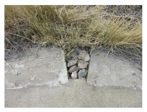
Photo C-6.1-3 August 2020—Redi-Rock block structure. Noted void between block 13 and 14 (as counted from north end of structure). Filled void with on-site rocks based on recommendation from 2019 Q4 inspection.
