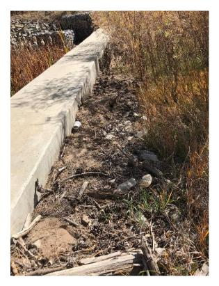
Photo C-2.2-3 October 2020—upslope face of weir, looking south. Recommend trash pickup.
