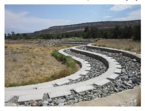
Photo C-6.1-2 August 2020—Redi-Rock block structure, looking southeast. Redi-Rock structure shows no evidence of displacement or settling. Vegetation well established.
