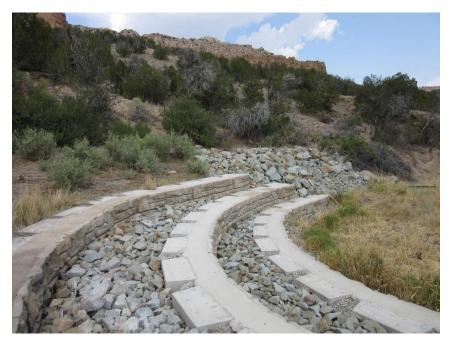
Photo C-6.2-1 August 2020—wetland north bank, looking northeast. Slope is stable with no evidence of erosion where riprap is located. Structure is functioning as designed with established vegetation.
