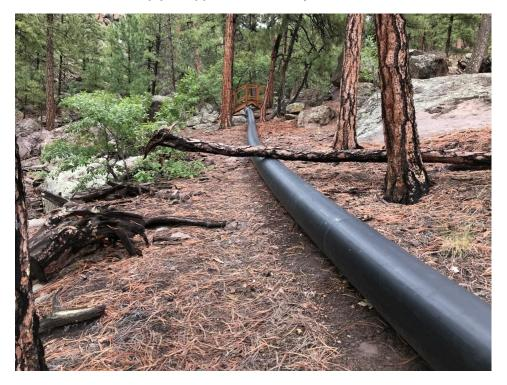
Photo C-3.6-8 September 2020—fallen tree on pipeline. Recommend relocation of fallen tree and repair of bridge.
