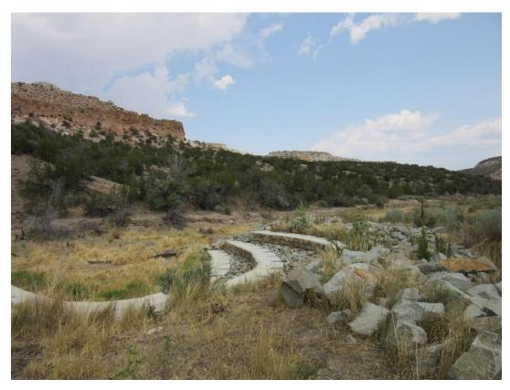
Photo C-6.4-1 August 2020—south bank berm, looking northeast. Berm is stable. No noted erosion or breaching, slides, or cracks in berm.
