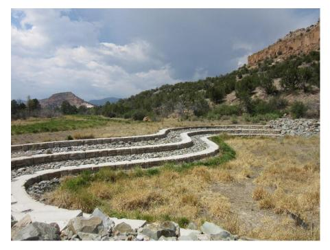
Photo C-6.1-1 August 2020—Redi-Rock block structure, looking north. Redi-Rock structure shows no evidence of displacement or settling. Vegetation well established.
