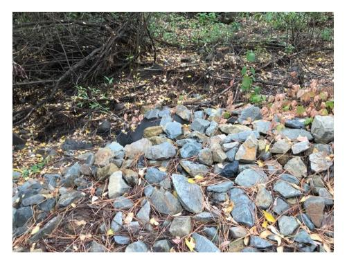
Photo C-3.9-5 September 2020—discharge culvert north of Los Alamos Canyon Road. Riprap area is steep and any size riprap presents a falling hazard. Area should stabilize naturally. No action recommended.
