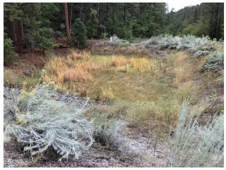
Photo C-3.1-1 September 2020—lower basin. No breaching/slides/cracks/sloughs present on embankment or pond. No erosion occurring on slope. No trash or debris present in control. Rodent burrows not encountered. Recommend removal of vegetation on the maintenance access path on the pond bank north of the Canyon Road.
