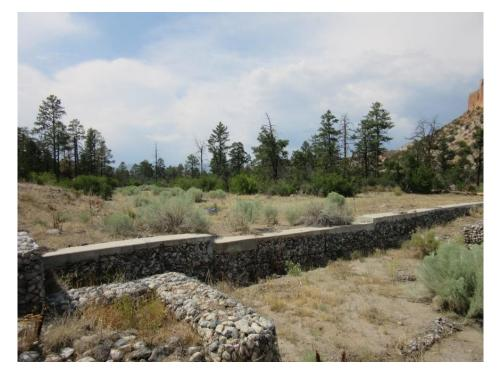
Photo C-5.1-1 August 2020—south embankment, looking west. Well established vegetation on embankment. No signs of erosion or undermining.
