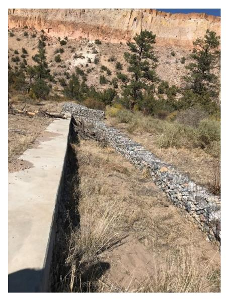
Photo C-5.4-4 October 2020—weir crest and flow-way, looking north. Recommend removal of fallen tree.
