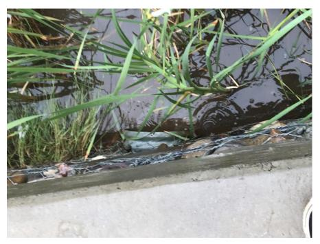
Photo C-2.7-1 September 2020—outlet. Evidence of corrosion noted in 2018. Pond level was at approximately 6 in. above the bottom of the outlet culvert at time of inspection. Will continue to monitor.
