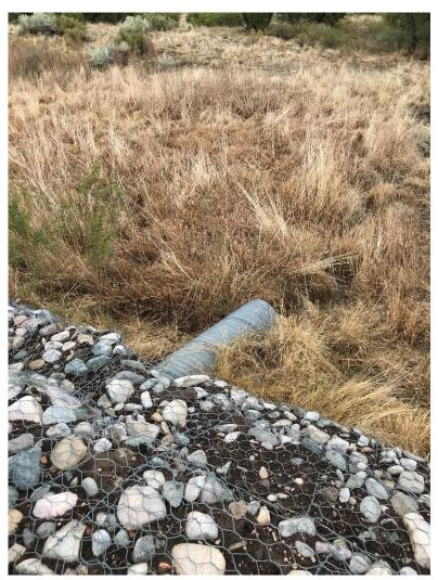
Photo C-4.10-1 September 2020—weir outlet. Erosion occurring in sediments deposited on top of gabion mattress apron. Rilling does not extend beyond the end of the gabion mattress apron. Sediment deposits on top of gabion mattress are approximately 1 in. below the bottom of the outlet invert. No action recommended.
