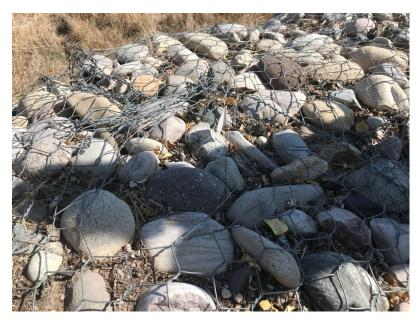
Photo C-4.7-6 October 2020—broken gabions on north end of crest. Recommend repair of holes in gabion basket.
