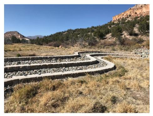
Photo C-6.1-4 October 2020—Redi-Rock block structure, looking north. No deficiency found.
