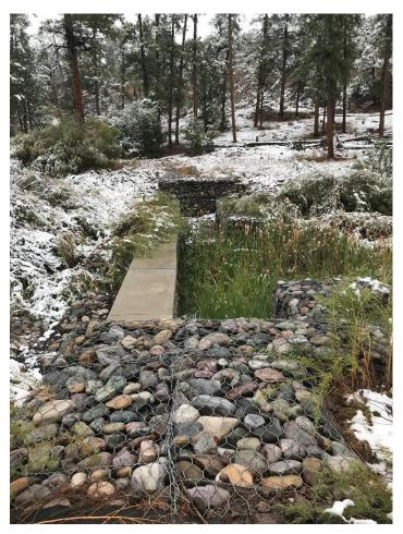
Photo C-2.6-1 September 2020—spillway alignment. Spillway operating as designed. No sign of improper alignment or deterioration. No trash encountered.
