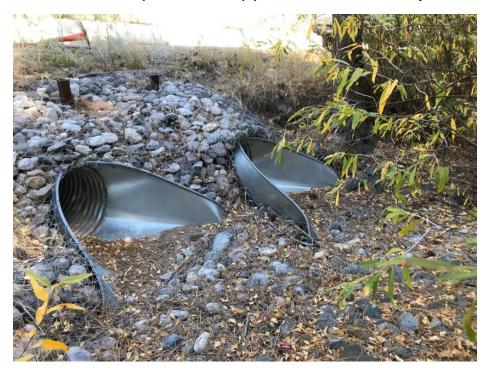
Photo C-3.9-4 October 2020—pipeline outlet. No deficiency found.
