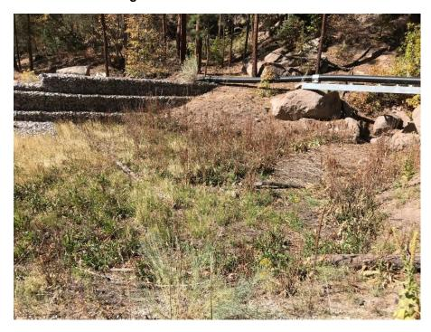
Photo C-3.2-2 October 2020—upper basin. Basin dry. Sloughing on south side of basin above where TRM was installed. Sides are retained by concrete jersey barrier at north road edge. Continue to monitor.
