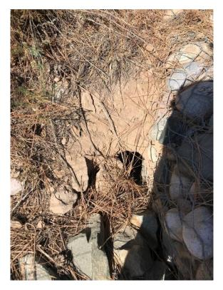
Photo C-2.2-4 October 2020—piping occurring at upslope face of weir. Recommend placing rock from nearby and on-site round riprap pile within the two voids upslope of weir near the north abutment.
