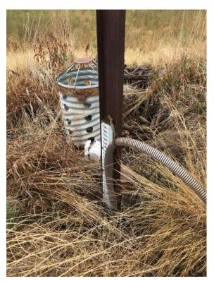
Photo C-4.9-1 September 2020—standpipe. Sediment and debris level at 4.6 ft on staff gage upstream of the weir.
