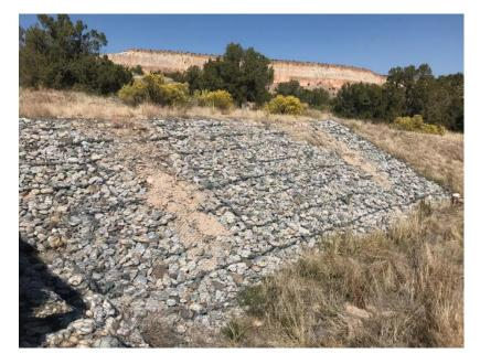
Photo C-4.3-4 October 2020—downstream northern embankment slope. Sediment deposited from runoff coming from dirt roads upgradient of the north side gabion embankment. Recommend placement of gravel bags at top of gabion on north bank downstream of the Los Alamos Canyon Weir.
