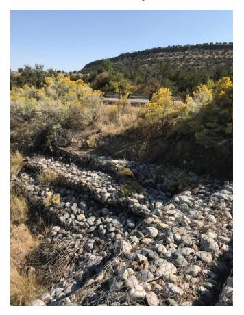
Photo C-4.3-2 October 2020—downstream southern embankment slope. No deficiency found.
