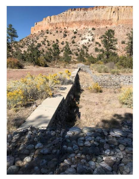
Photo C-5.4-3 October 2020—weir spillway and flow-way, looking north. Recommend removal of tall vegetation located on upstream side of spillway.
