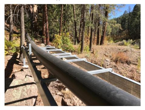
Photo C-3.8-2 October 2020—pipeline bridge structure. Control is operating as designed with no apparent issues to structure.
