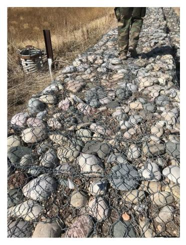
Photo C-4.7-7 October 2020—broken gabion wires on south end of weir crest. Recommend repair.
