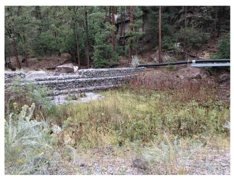
Photo C-3.2-1 September 2020—upper basin. Sloughing on south bank of the Upper Pond above where TRM was installed. Sides are retained by concrete jersey barrier at edge of road. Continue to monitor.
