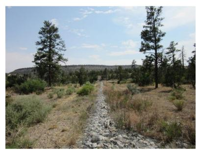
Photo C-5.2-1 August 2020—embankment abutment from north side of channel, looking south. Well established vegetation surrounding control. No presence of trash or debris.
