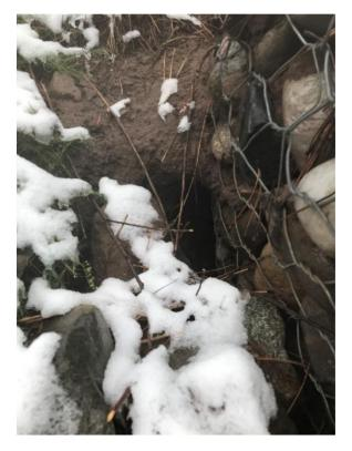
Photo C-2.2-2 September 2020—piping occurring at upslope face of weir. Continue to monitor.
