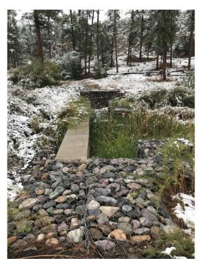
Photo C-2.3-1 September 2020—crest of weir structure looking upslope. No deteriorated joints present on upslope side of weir. Gabion basket is structurally intact and in stable condition.
