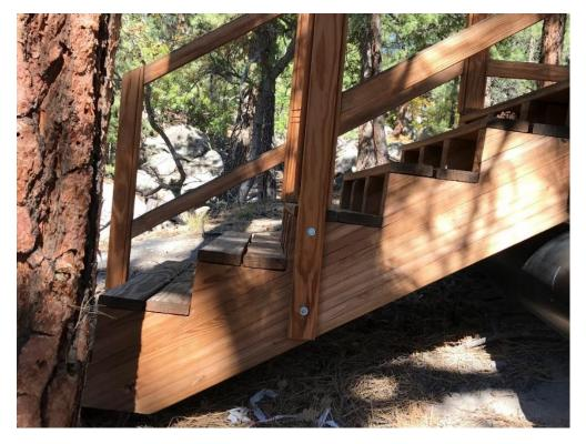
Photo C-3.6-10 October 2020—bridge. Recommend repair of bridge.
