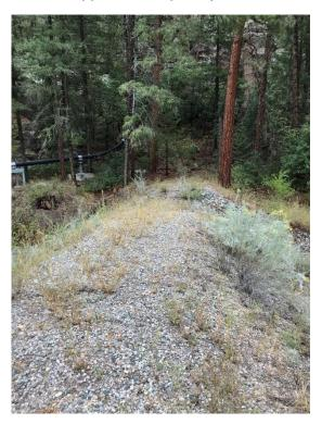
Photo C-3.4-1 September 2020—upper basin spillway. No signs of erosion occurring on or near spillway. Spillway is maintaining alignment and stability.
