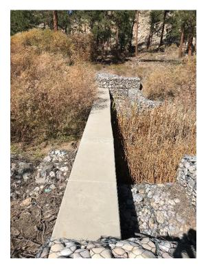
Photo C-2.3-2 October 2020—weir structure looking upslope. No significant change since last inspection.
