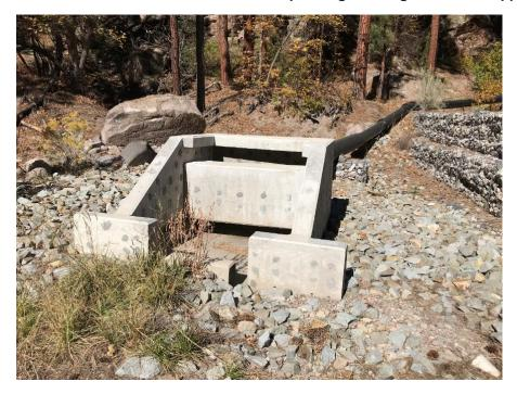
Photo C-3.9-2 October 2020—pipeline outlet, energy dissipater, and gabion overflow structure. Control is operating as designed with no apparent issues to structure.
