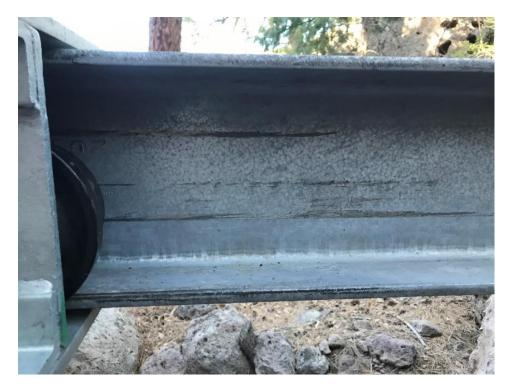
Photo C-3.6-7 October 2020—beam trolley support. Caster gouging and degradation of coating due to skewed support on beam trolley support 15. Continue to monitor gouging on pipe support beam trolleys.
