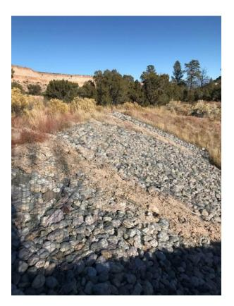
Photo C-4.3-3 September 2020—downstream northern embankment slope. Sediment deposited from runoff coming from dirt roads upgradient of the north side gabion embankment. Recommend placement of gravel bags at top of gabion on north bank downstream of the Los Alamos Canyon Weir.
