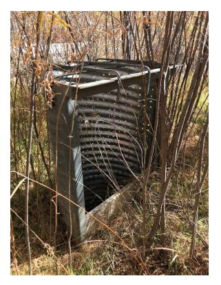
Photo C-2.5-3 October 2020—standpipe. No significant change since last inspection.
