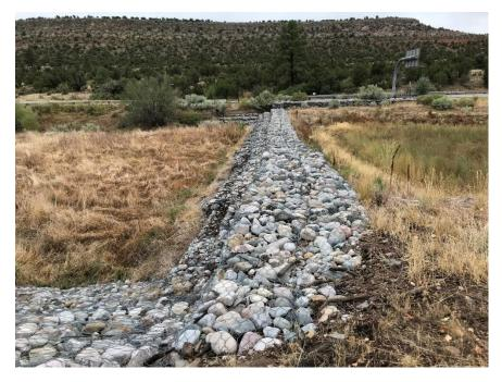
Photo C-4.7-2 September 2020—weir crest. Recommend repair of holes in gabion basket.
