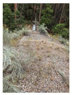
Photo C-3.3-1 September 2020—lower basin spillway. No signs of erosion occurring on or near spillway. Spillway is maintaining alignment and stability.
