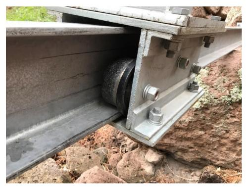
Photo C-3.6-6 September 2020—beam trolley support. Caster gouging and degradation of coating due to skewed support on beam trolley support 15. Continue to monitor gouging on pipe support beam trolleys.
