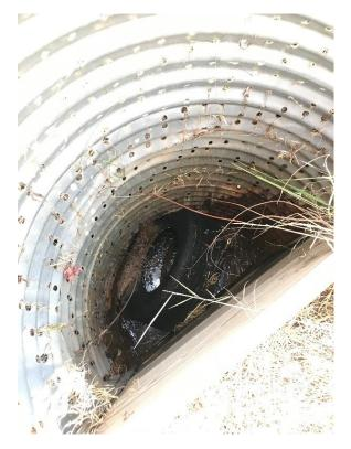
Photo C-2.5-4 September 2020—standpipe. Recommend removal of tire.
