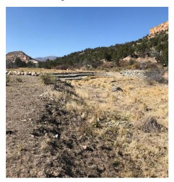
Photo C-6.3-2 October 2020—south bank, looking west. South bank is susceptible to erosion. Loose soil in voids where fallen riprap was placed. Recommend placement of jute erosion-control matting, wire-enclosed riprap, or brush barriers at toe of slope on south bank downstream of Pueblo Canyon Wetland grade-control structure. C-6.4 Downstream South Bank
