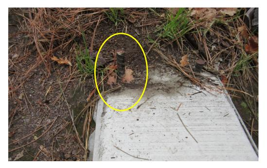
Photo C-3.6-3 September 2020—pipeline headwall. Rebar sticking up on headwall is a tripping hazard. Recommend removal.
