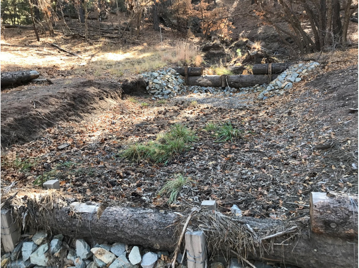
Photo B-2.0-2 November 4, 2020 – upper log check dam
