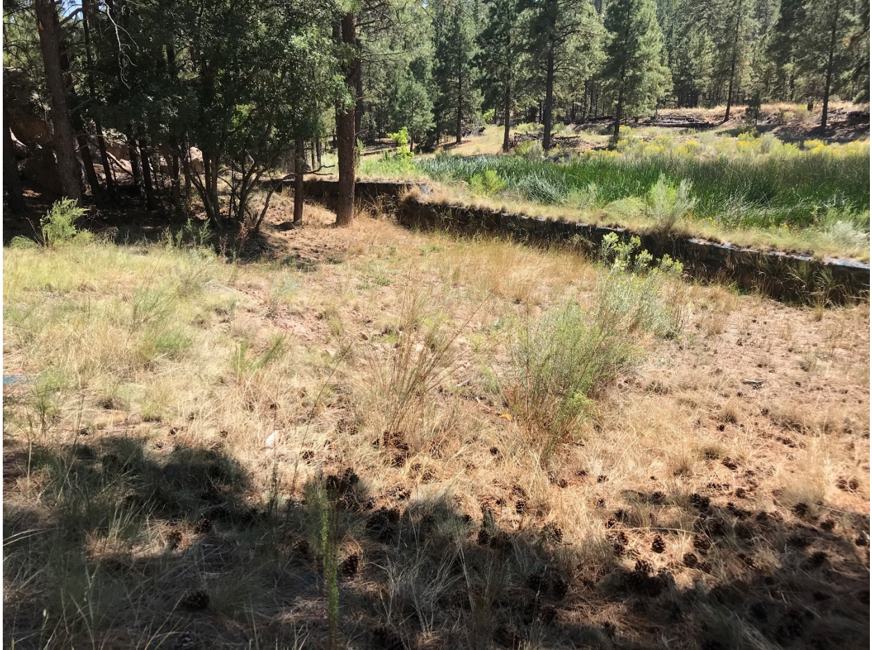
Photo B-3.8-2 September 4, 2020—lower run-on cell barrier, looking southwest, sediment level 4–5 ft below top of spillway
