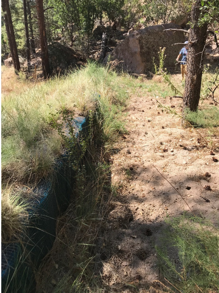
Photo B-3.7-1 September 4, 2020—Upper run-on cell barrier looking east. Sediment level at 1 ft below top of spillway.
