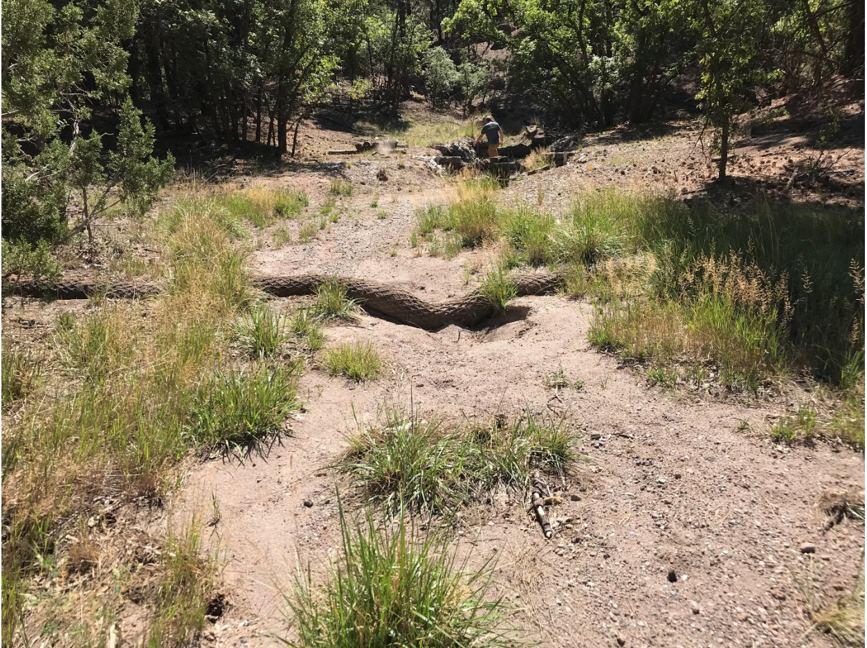
Photo B-2.0-4 September 4, 2020 – coir log, view looking south, recommend removal to address local scour
