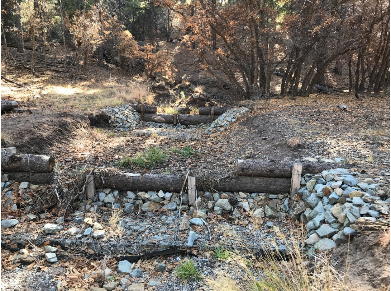
Photo B-2.0-3 November 4, 2020 – lower log check dam, log check dam 2, view looking south
