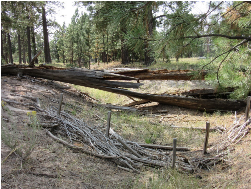
Figure 12 Juniper bale check dam located in drainage channel to 90s Line Pond, September 2020. Note vegetation in channel.
