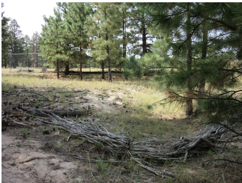
Figure 10 Juniper bale check dam located in drainage channel to 90s Line Pond, September 2020. Note vegetation in channel.
