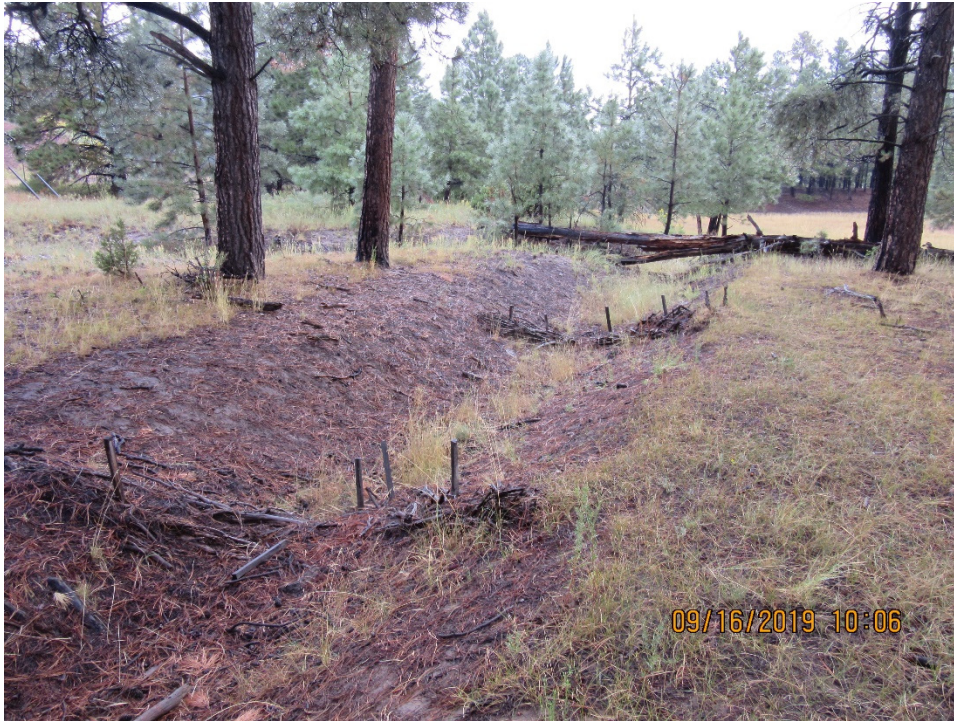
Figure 5 Juniper bale check dams located in drainage channel to 90s Line Pond, September 2019. Note vegetation in channel.
