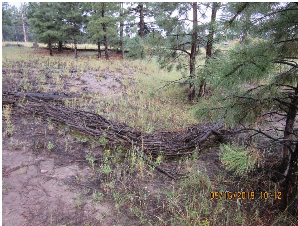
Figure 9 Juniper bale check dam located in drainage channel to 90s Line Pond, September 2019. Note vegetation in channel.
