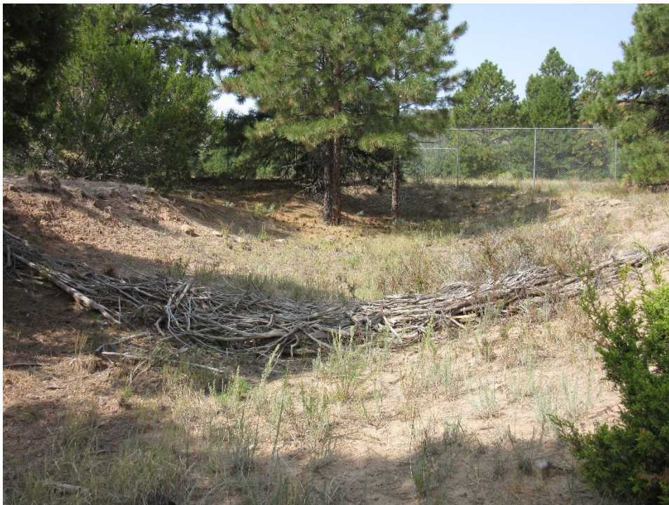
Figure 8 Juniper bale check dam located in drainage channel to 90s Line Pond, September 2020. Note vegetation in channel.
