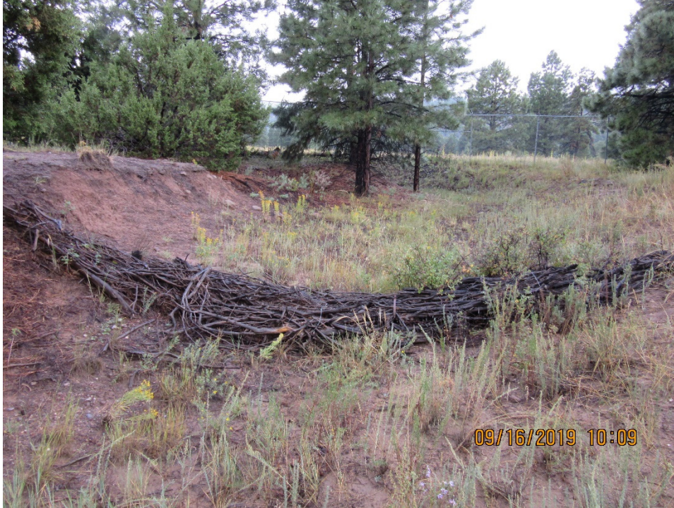
Figure 7 Juniper bale check dam located in drainage channel to 90s Line Pond, September 2019. Note vegetation in channel.
