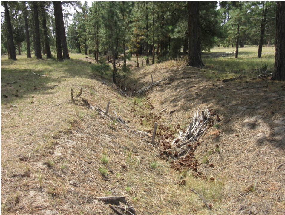
Figure 6 Juniper bale check dams located in drainage channel to 90s Line Pond, September 2020. Note vegetation in channel.
