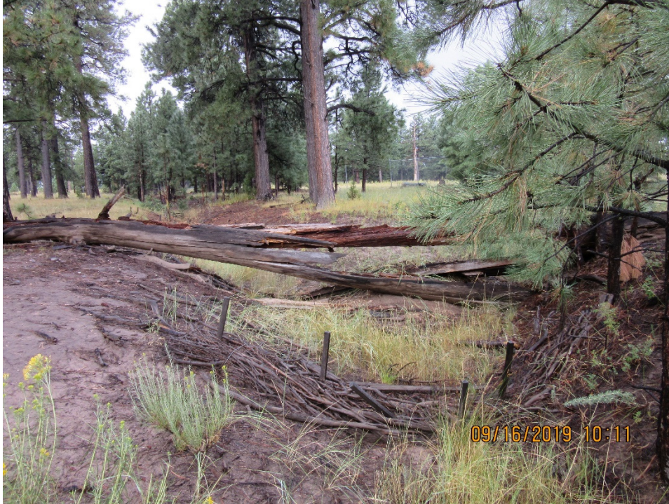
Figure 11 Juniper bale check dam located in drainage channel to 90s Line Pond, September 2019. Note vegetation in channel.
