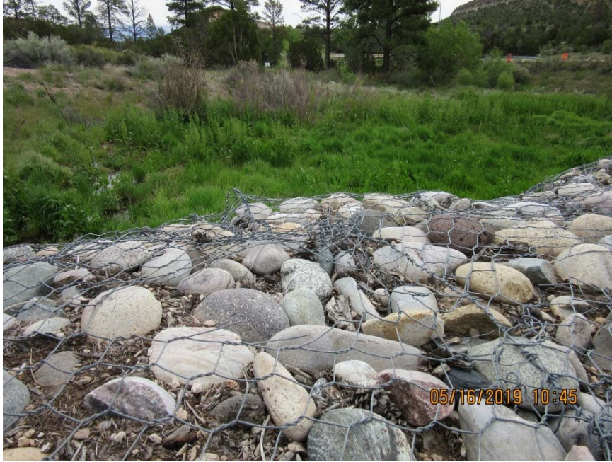
Photo C-4.7-2 May 2019—broken gabion wires on north end of weir crest. Recommend repair of holes in gabion basket.
