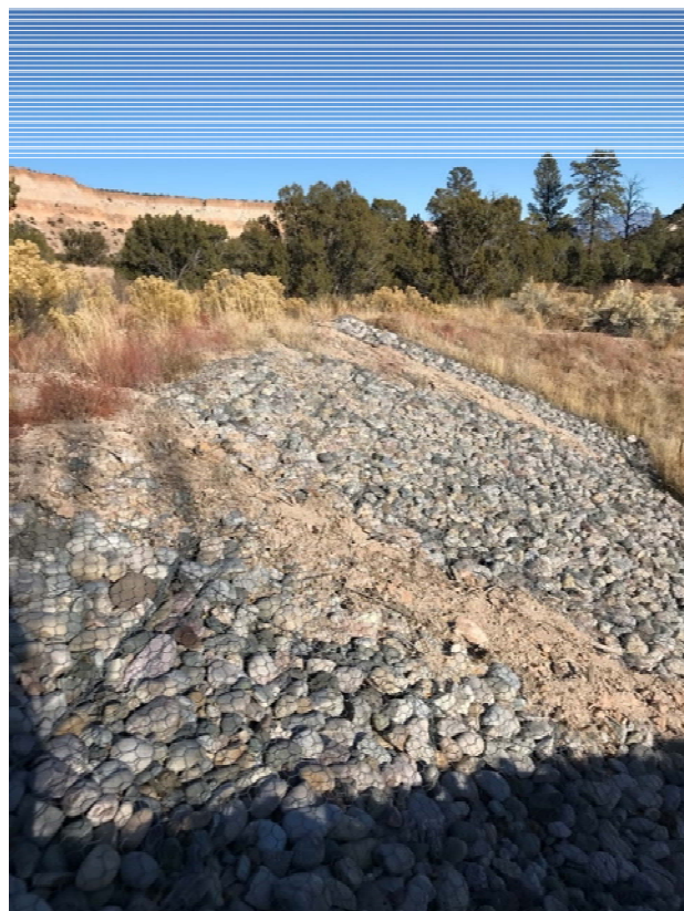
Photo C-4.3-5 November 2019—downstream northern embankment slope. Recommend wattle or gravel bag placement on top of gabion baskets.
