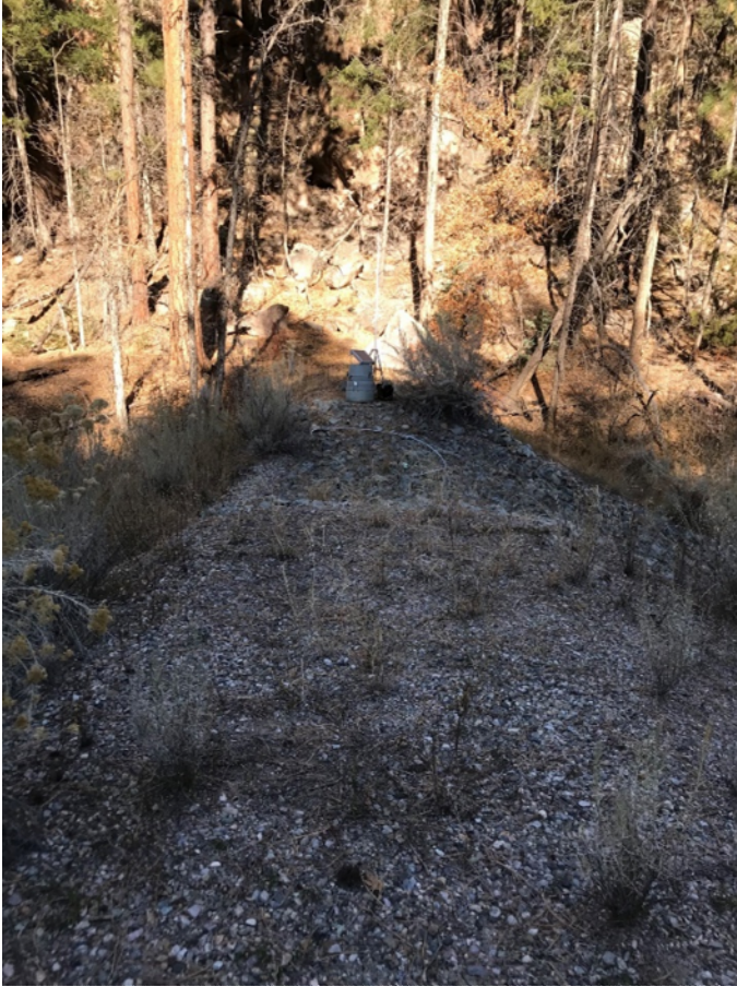
Photo C-3.3-3 November 2019—lower basin spillway. No signs of erosion occurring on or near spillway. Spillway is maintaining alignment and stability. Rodent burrows encountered. Will continue to monitor.
