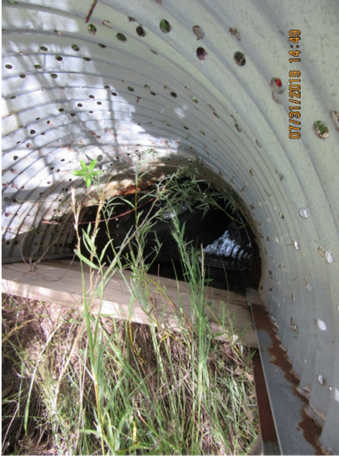
Photo C-2.5-3 Flow event inspection for July 25, 2019, storm event—standpipe. No change in sediment level since last inspection.
