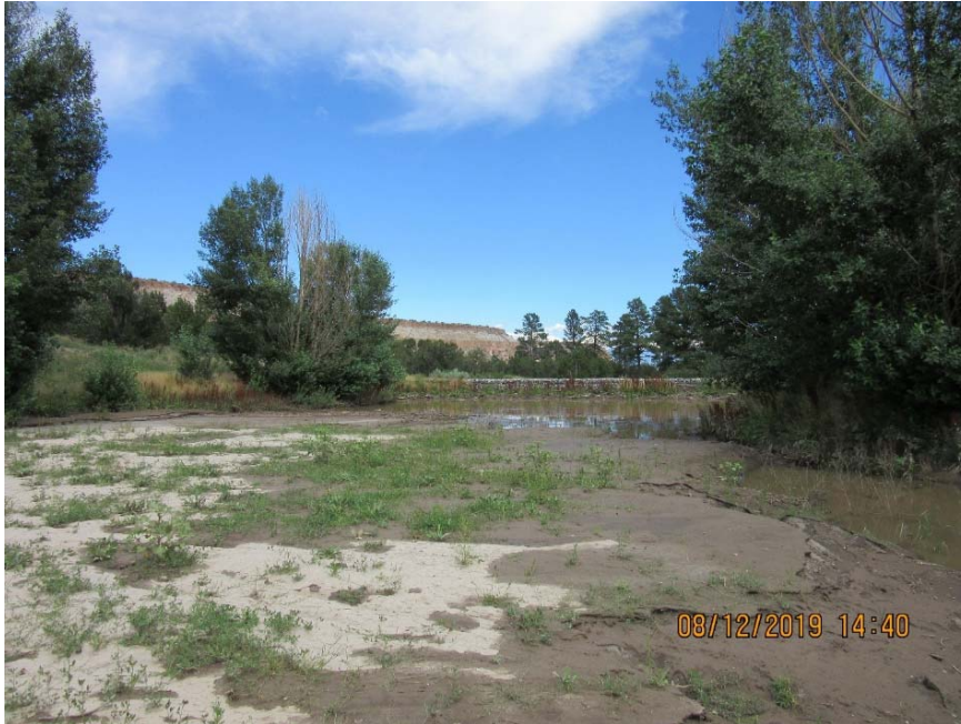
Photo C-4.6-3 Flow event inspection for August 7, 2019, storm event—Los Alamos Pond 3 (lower). Sediment deposition area extended approximately 3 ft to the east (downstream).
