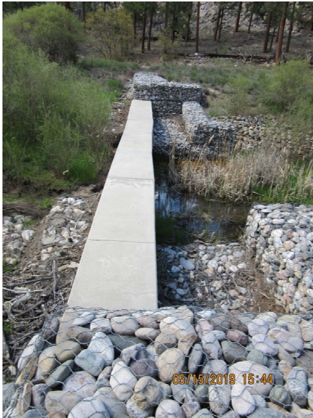
Photo C-2.6-1 May 2019—spillway alignment. Spillway operating as designed. No sign of improper alignment or deterioration. Recommend removal of trash encountered.
