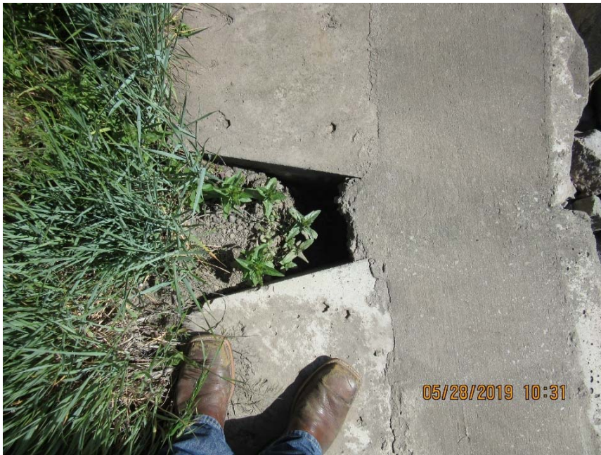
Photo C-6.1-3 May 2019—Redi-Rock block structure. Preferential flow path located mid-upper level. The crushed stone placed in the void space between block 13 and 14 (as counted from north end of structure) washed out. Will continue to monitor.
