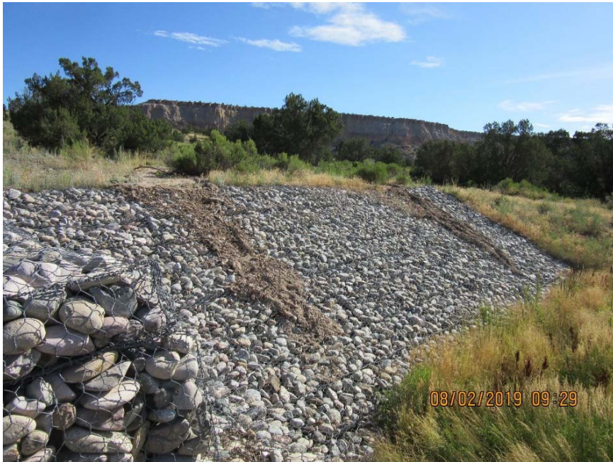
Photo C-4.3-3 Flow event inspection for July 26, 2019, storm event—downstream northern embankment slope. Recommend wattle or gravel bag placement at top of gabion baskets.
