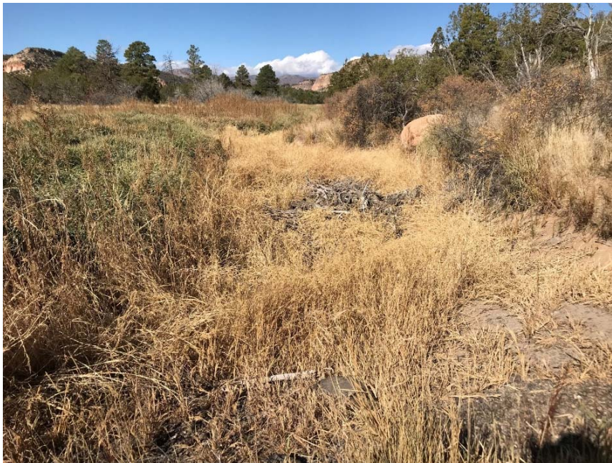
Photo C-6.5-2 October 2019—upstream pond, looking upstream. Pond is dry. TRM is covered with sediment. Pond has approximately 1-ft depth for accumulation of sediment.
