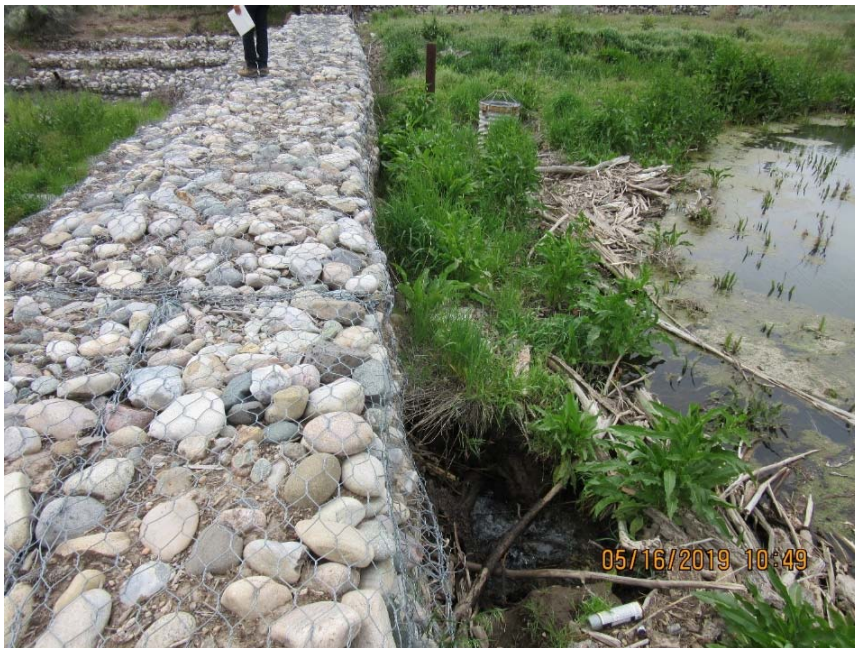
Photo C-4.2-1 May 2019—abutment looking south. Sinkholes still present. Four to five areas of preferential flow. Will continue to monitor. Lower pond filled with approximately 2-3 ft water. Actively flowing. Minor amount of trash on upstream side against the abutment. Recommend collection and disposal of trash.
