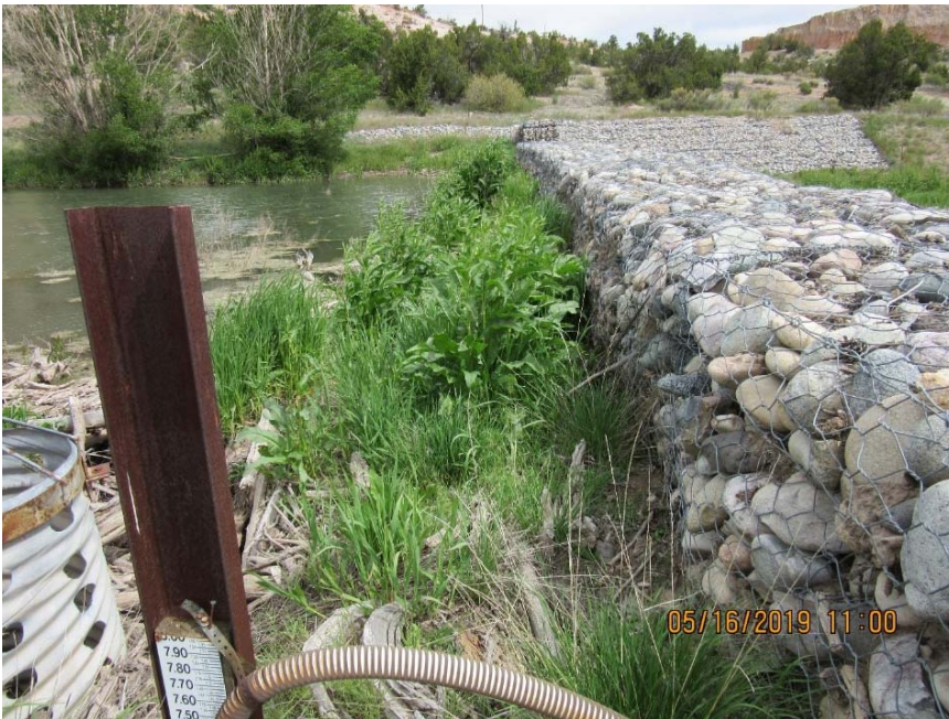
Photo C-4.7-1 May 2019—upstream weir face. Continue to monitor bulging gabion baskets.
