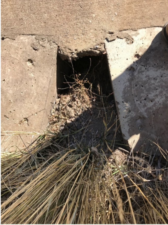
Photo C-6.1-6 October 2019—Redi-Rock block structure. Note preferential flow path. Recommend fill of void with a large gradation gravel.
