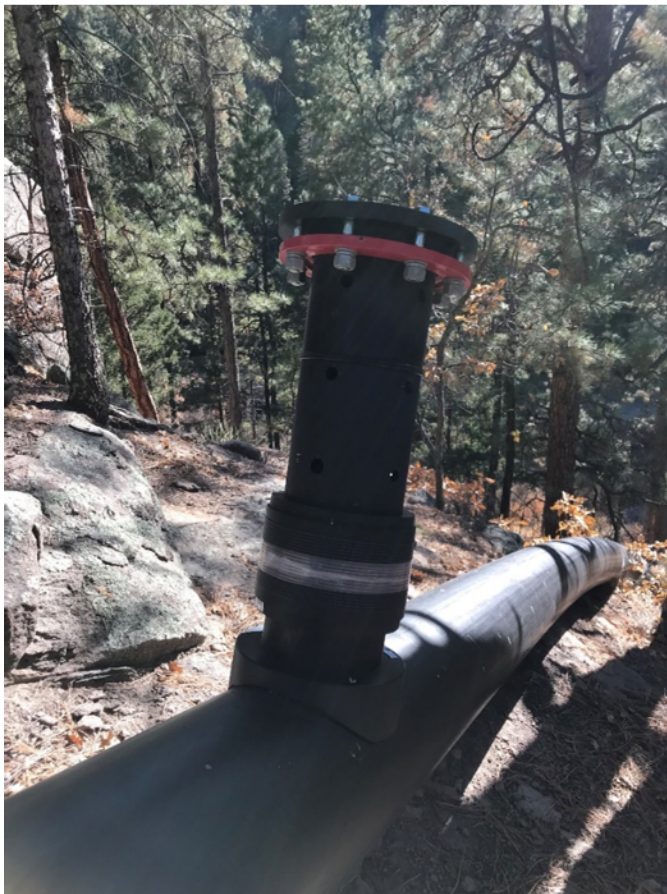
Photo C-3.7-3 November 2019—pipeline vacuum breaker. Control is operating as designed with no apparent issues to structure.
