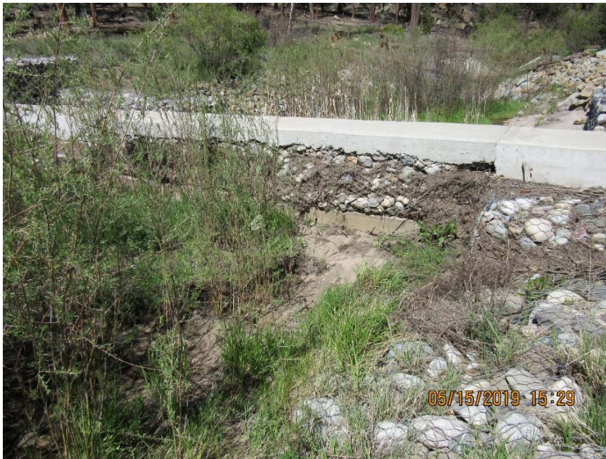
Photo C-2.2-1 May 2019—upslope face of weir, looking east. Weir is functioning; no deteriorating joints or bulging gabion baskets.
