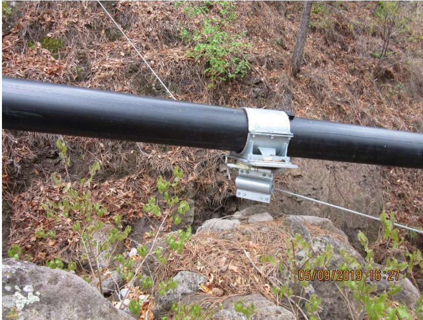
Photo C-3.6-5 May 2019—Pipeline cable support is no longer skewed.
