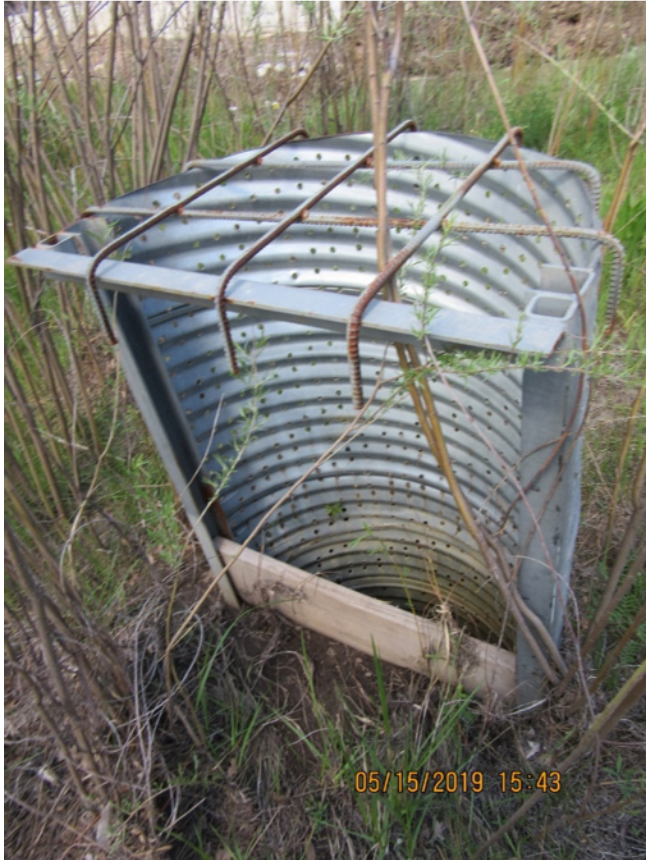
Photo C-2.5-1 May 2019—standpipe. Sediment level is approximately 1 ft below wood board stop. No significant change since last inspection. Will continue to monitor.
