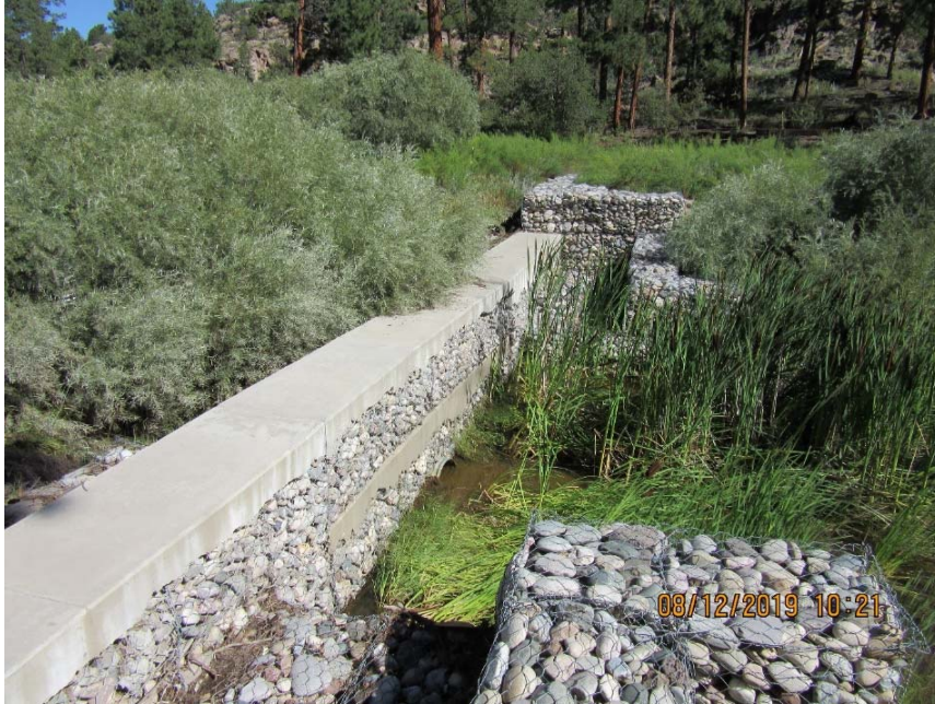
Photo C-2.7-3 Flow event inspection for August 7, 2019, storm event—outlet. Pond level was at approximately 6 in. above the bottom of the outlet culvert at time of inspection.
