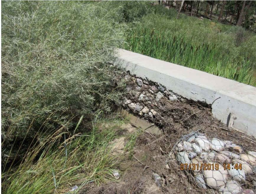
Photo C-2.2-2 Flow event inspection for July 25, 2019, storm event—upslope face of weir, looking east. Some trash/debris present.
