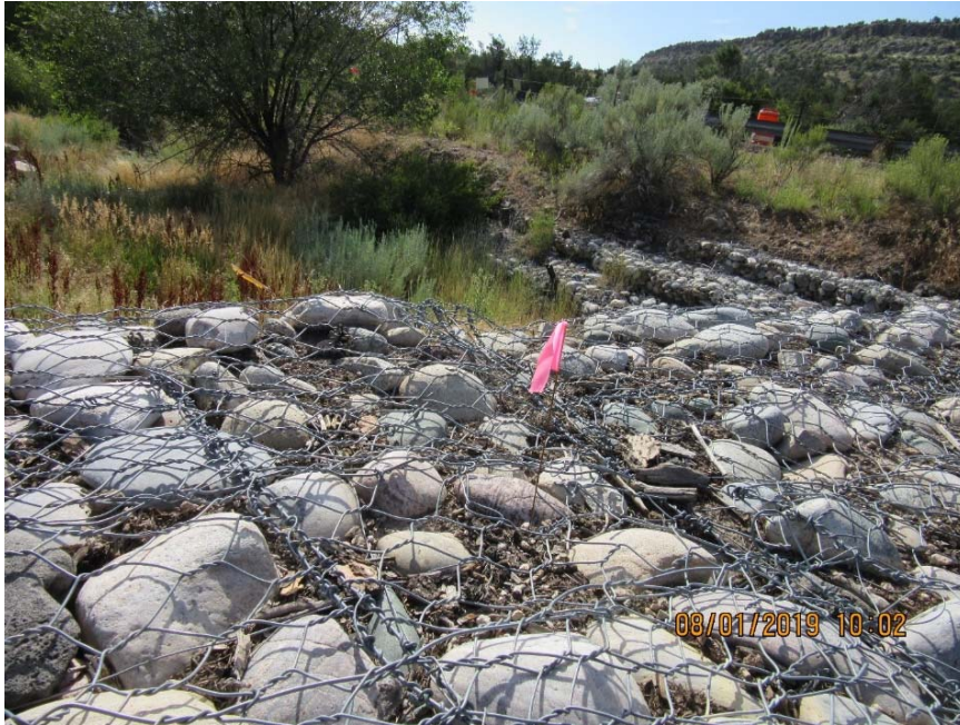
Photo C-4.7-4 Flow event inspection for July 26, 2019, storm event—broken gabion wires on north end of weir crest. Recommend repair.
