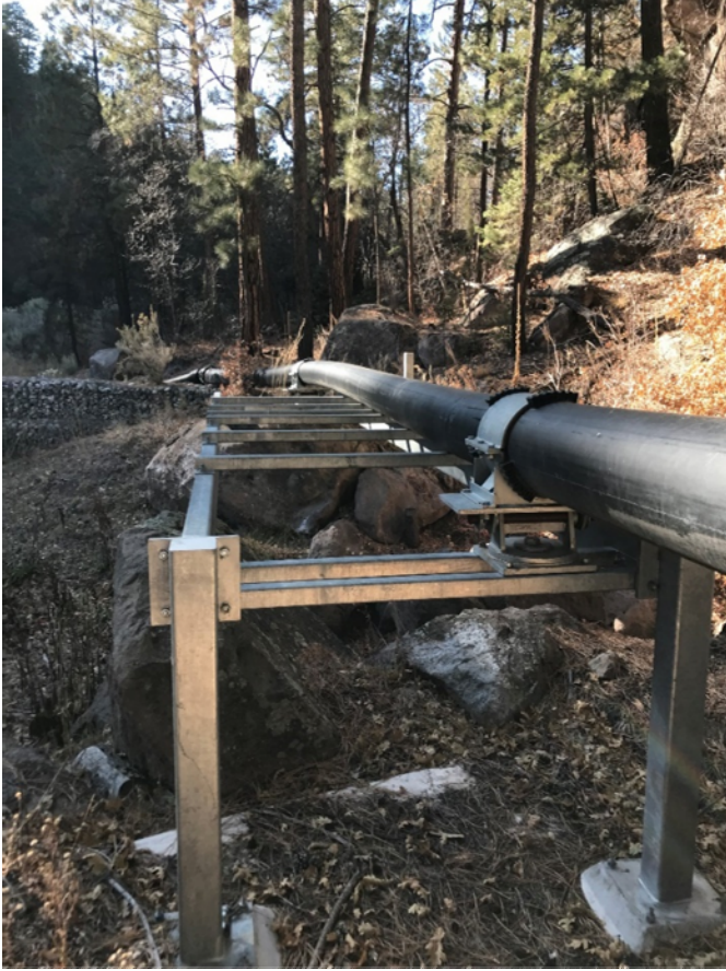
Photo C-3.8-3 November 2019—pipeline bridge structure. Control is operating as designed with no apparent issues to structure.
