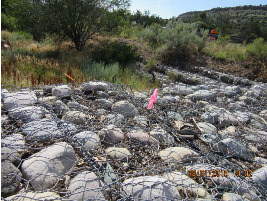
Photo C-4.3-2 Flow event inspection for July 26, 2019, storm event—downstream southern embankment slope. Sediment deposited from runoff coming from dirt roads upgradient of the northside gabion embankment. Will continue to monitor.
