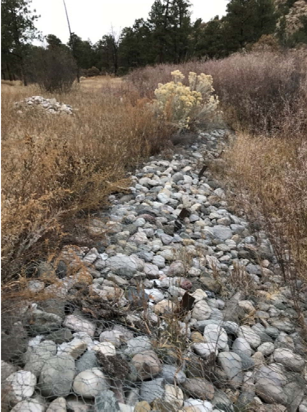
Photo C-2.1-3 November 2019—Embankment is stable and operating as designed. Well-established vegetation with no erosion occurring from hillslope. One rodent hole encountered. Recommend continued monitoring.
