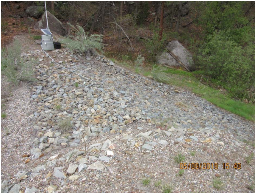
Photo C-3.3-1 May 2019—lower basin spillway. No signs of erosion occurring on or near spillway. Spillway is maintaining alignment and stability.
