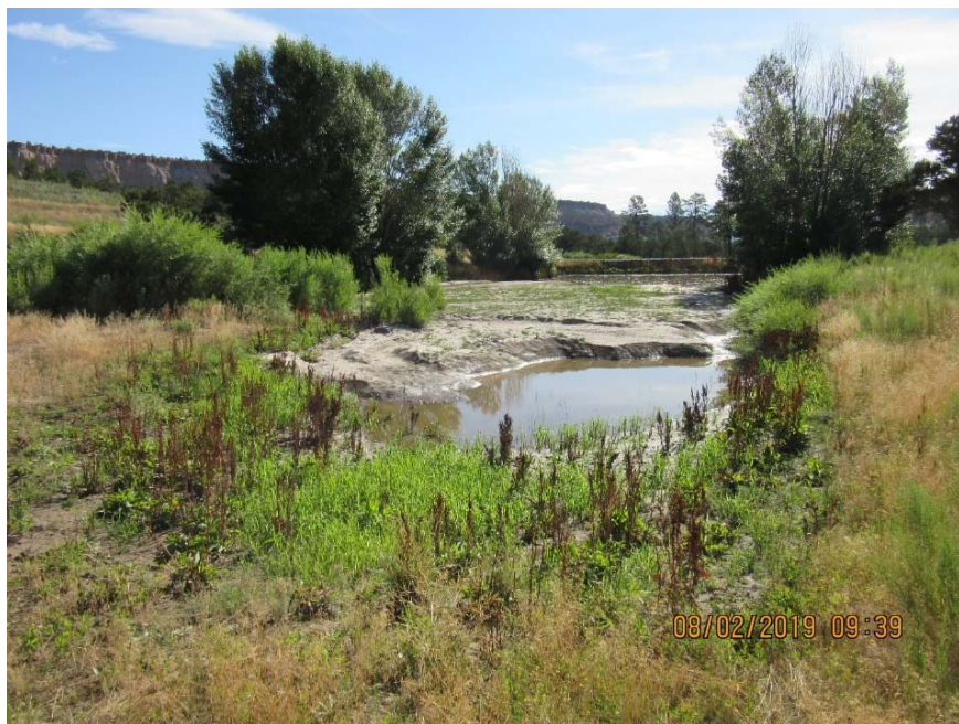
Photo C-4.5-2 Flow event inspection for July 26, 2019, storm event—Los Alamos Pond 2 (middle) looking downstream. Pond has been breached. No sediment capacity at flow line. Deposition of medium gradation (approximately 0.25-in.-diameter) size sediments noted at flow line.
