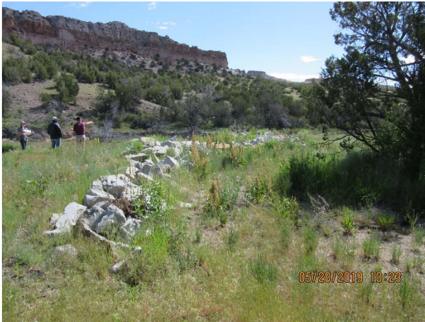
Photo C-6.4-1 May 2019—south-bank berm, looking northeast. Berm is stable; no noted erosion or breaching/slides/cracks to berm.
