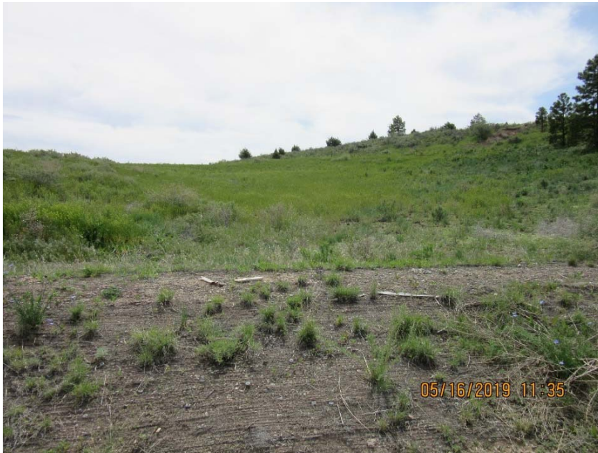
Photo C-4.11-1 May 2019—borrow pit and berm. Minor erosion on upper end of borrow pit. Vegetation well established.
