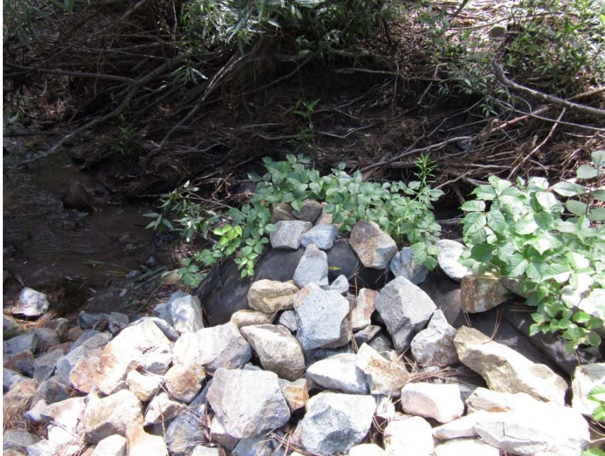
Photo C-3.6-11 Flow event inspection for August 7, 2019, storm event—discharge culvert north of Los Alamos Canyon road. Geotextile exposed. Recommend placement of riprap to cover geotextile.
