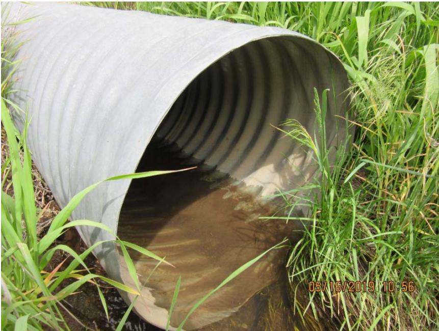
Photo C-4.10-1 May 2019—weir outlet. Water flowing/seeping through gabions at various locations. Pipe has some flow. Continue to monitor erosion occurring 50–60 ft downstream of the weir. No sediment present. Highly vegetated.
