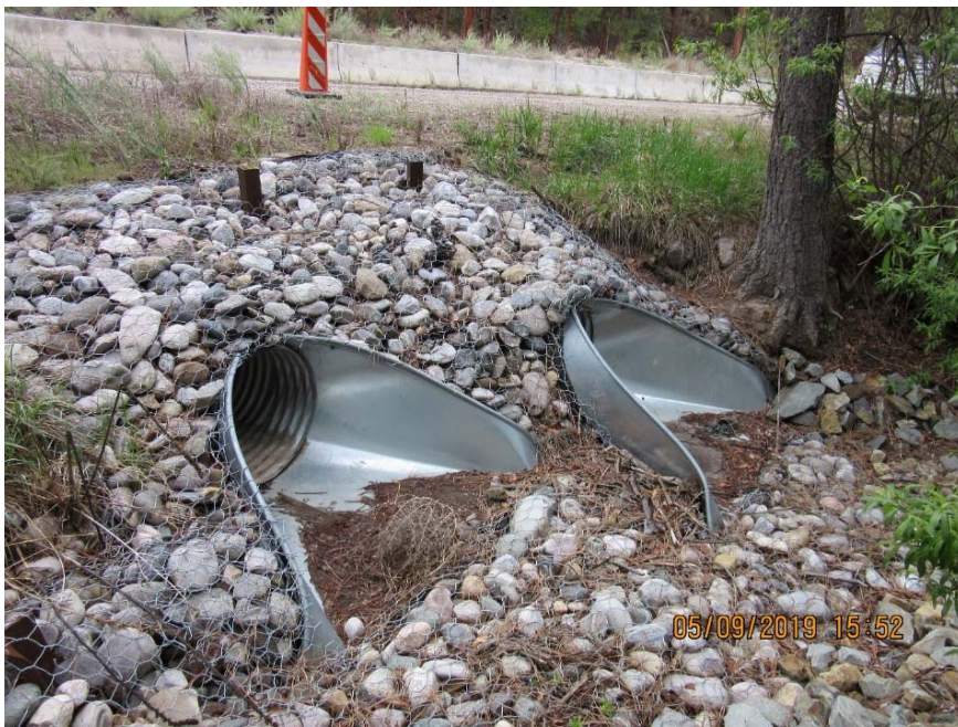
Photo C-3.6-8 May 2019—pipeline outlet downstream of Los Alamos Canyon road
