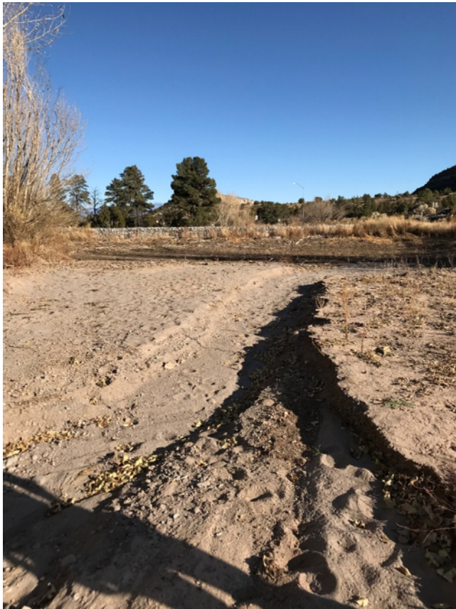
Photo C-4.4-2 November 2019—Los Alamos Pond 1 (upper) looking downstream. Pond has been breached and has no sediment capacity.
