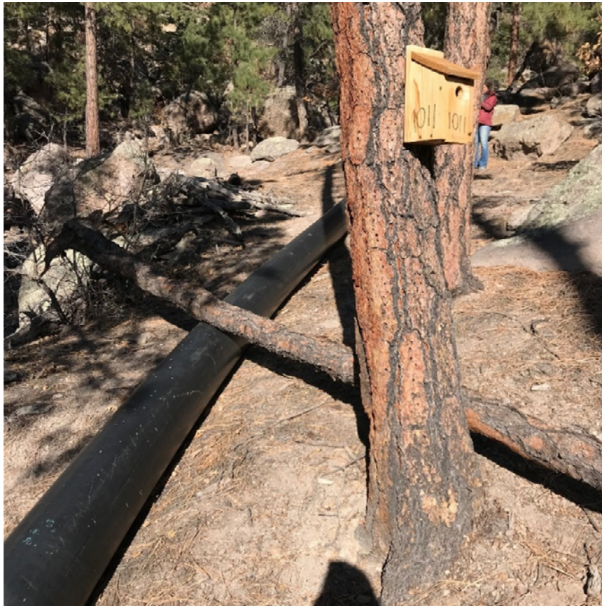
Photo C-3.6-12 November 2019—Tree fell on pipeline. Removal recommended.
