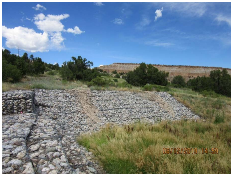
Photo C-4.3-4 Flow event inspection for August 7, 2019, storm event—downstream northern embankment slope. Surface water collecting on the paths downstream of the weir causing deposition of coarse sediments on the north gabion embankment. Recommend placement of gravel bags or wattles at the top of the gabions and relocating sediments deposited to north of the gravel bags or wattles.
