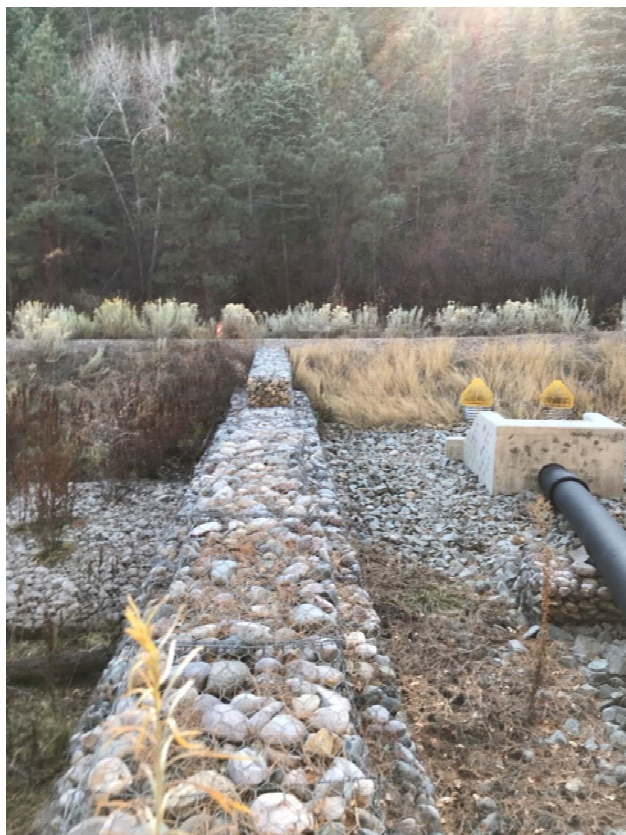
Photo C-3.6-13 November 2019—discharge culvert inlet and riser pipe. Evidence of water level found at top of spillway (needlecast deposition).
