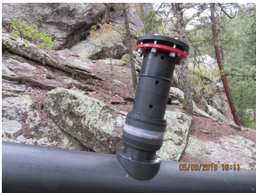
Photo C-3.7-1 May 2019—pipeline vacuum breaker. Control is operating as designed with no apparent issues to structure.
