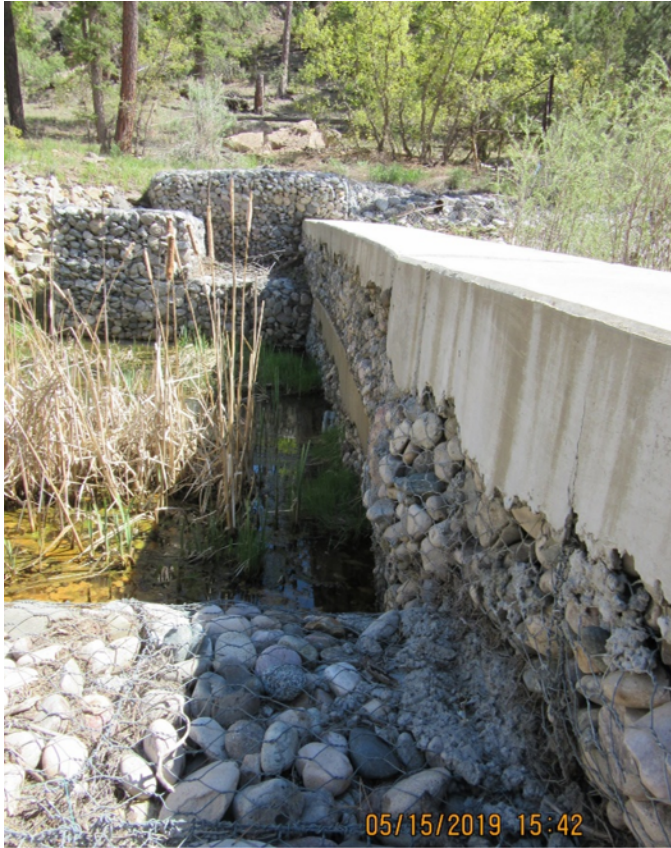
Photo C-2.4-1 May 2019—downstream face of weir. Continue to monitor bulging gabion baskets. No evidence of cracking/spalling; area is clear of debris.
