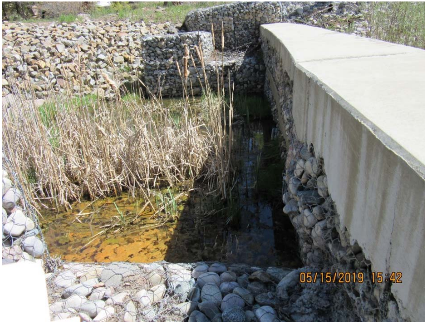
Photo C-2.7-1 May 2019—outlet. Evidence of corrosion noted in 2018. Pond level was at approximately 6 in. above the bottom of the outlet culvert at time of inspection. No evidence of undercutting, erosion, or excessive sediment deposition. Fallen trees are present downstream of GCS—one upstream of flow gage and one downstream of flow gage. Recommend removal of fallen trees. Sediment level to 6 in. above outlet culvert invert elevation. Will continue to monitor.
