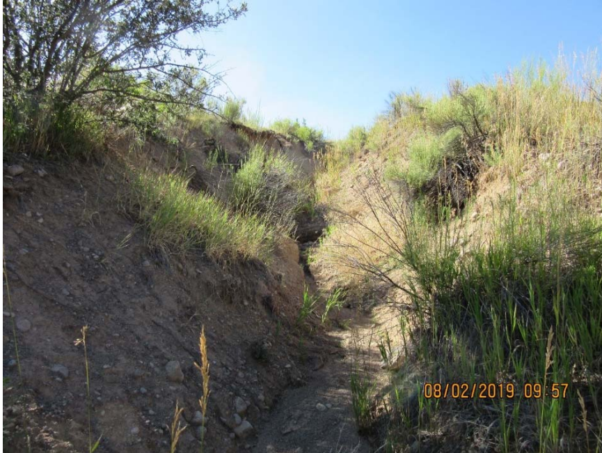
Photo C-4.11-5 Flow event inspection for July 26, 2019, storm event—borrow pit. Channelization is stabilized upstream of a log in the large undercut area. Will continue to monitor. Berm and TRM damage noted at north end of the berm. Damage occurred during nearby Los Alamos County well construction. Recommend discussion with Los Alamos County to repair berm and TRM damage. Filter fabric exposed and detached downstream of the berm on the south end. Recommend filter fabric restapling and then covering with base course.
