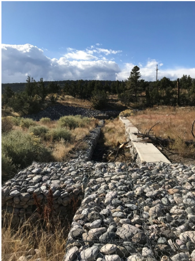
Photo C-5.4-4 October 2019—weir crest and flow-way, looking south. Recommend relocation of fallen tree.
