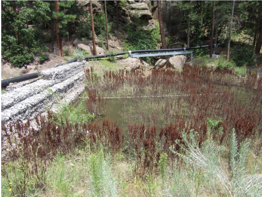
Photo C-3.2-2 Flow event inspection for August 7, 2019, storm event—upper basin. Sloughs due to wildlife tracts upgradient of turf-reinforcement mat (TRM). Fallen tree in pond. Vegetation growth noted on basin maintenance access. Recommend to clean up vegetation growth on the maintenance access paths.
