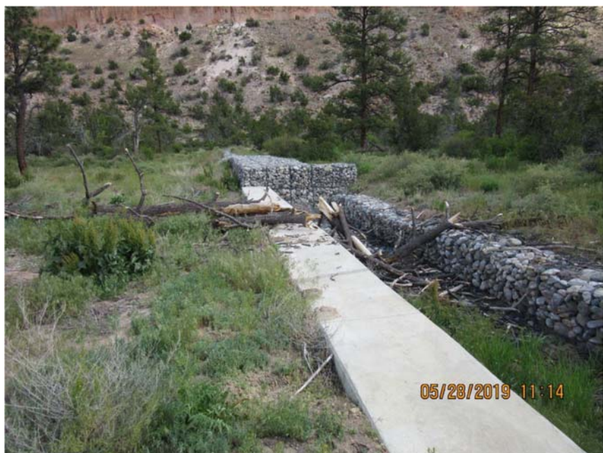
Photo C-5.4-2 May 2019—weir crest and flow-way, looking north. A tree has fallen over the overflow weir structure. Recommend removal of the tree. Bulging gabions and minor cracks present. Gabion wiring has failed in one location and created a hole approximately 1 ft in diameter. Recommend repair.
