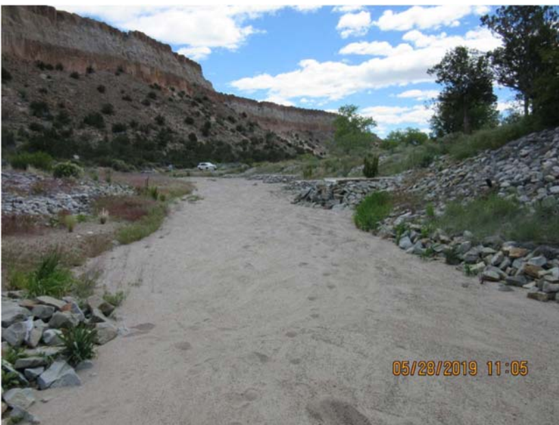
Photo C-5.5-1 May 2019—Redi-Rock spurs, looking east. Well-established vegetation along all hillslopes. No erosion apparent along slopes or near TRM. All structures functioning as designed.
