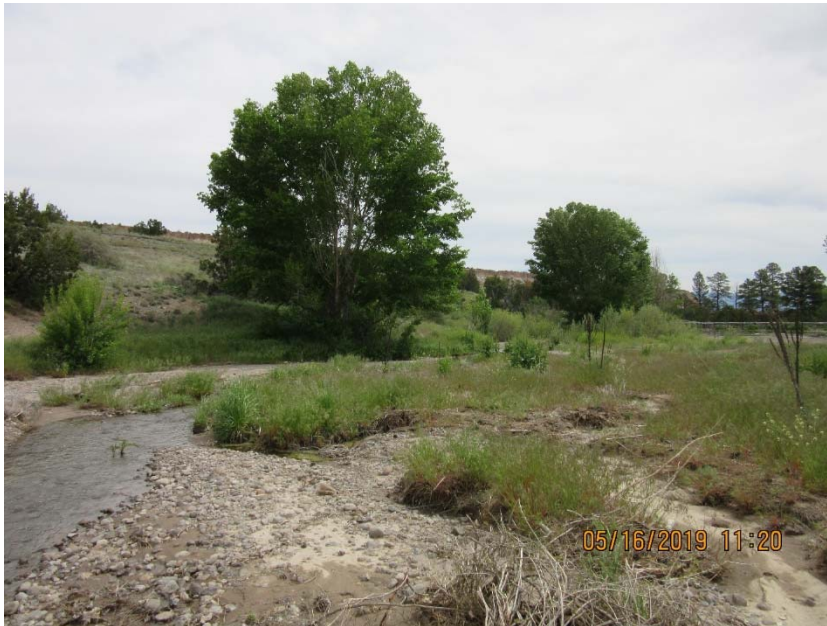
Photo C-4.4-1 May 2019—Los Alamos Pond 1 (upper) looking downstream. Pond appears to have been breached. Pond has no capacity to retain sediment.
