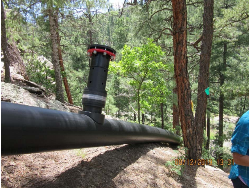
Photo C-3.7-2 Flow event inspection for August 7, 2019, storm event—pipeline vacuum breaker. Control is operating as designed with no apparent issues to structure.
