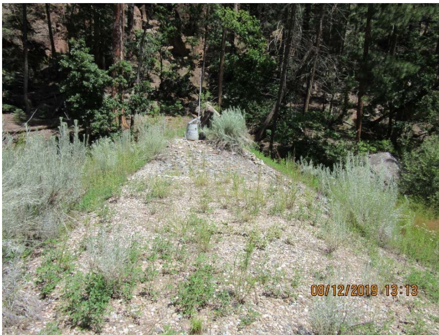
Photo C-3.3-2 Flow event inspection for August 7, 2019, storm event—lower basin spillway. Needlecast and taller vegetation noted. Recommend cleanup of vegetation growth on the spillway.
