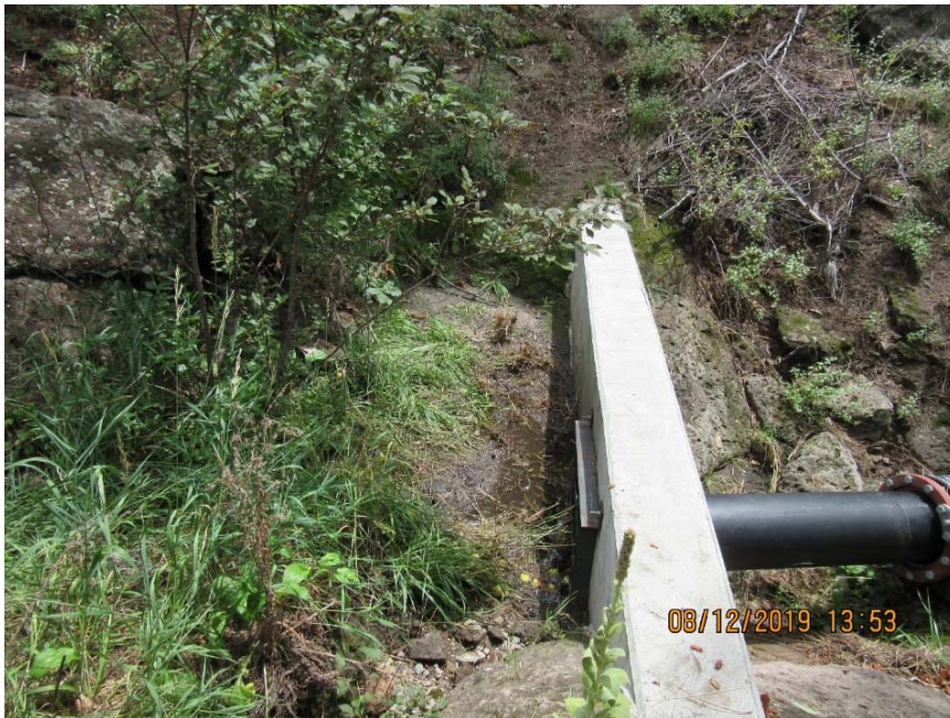
Photo C-3.6-2 Flow event inspection for August 7, 2019, storm event—pipeline headwall. Needlecast debris was removed.
