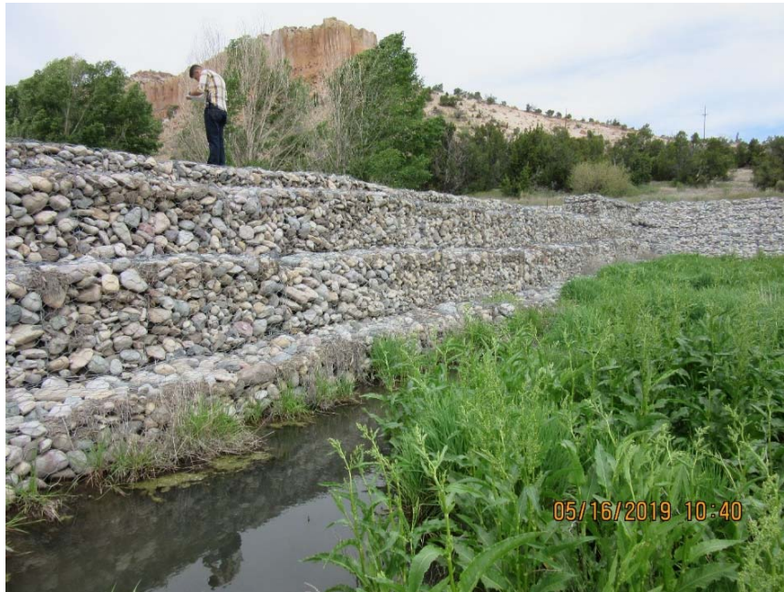
Photo C-4.8-1 May 2019—downstream weir face. Continue to monitor bulging baskets and joints.
