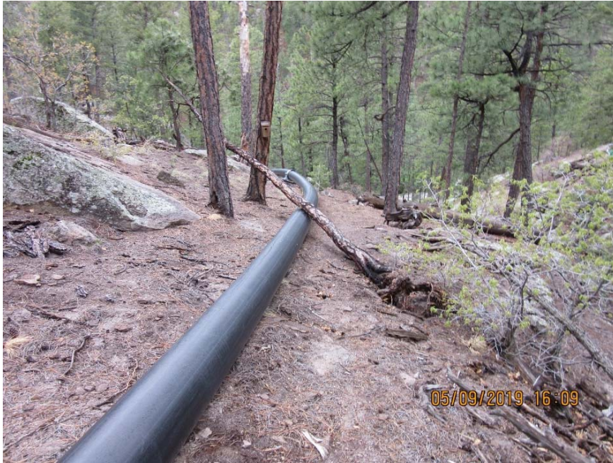
Photo C-3.6-7 May 2019—fallen tree on pipeline. Recommend relocation of fallen tree.
