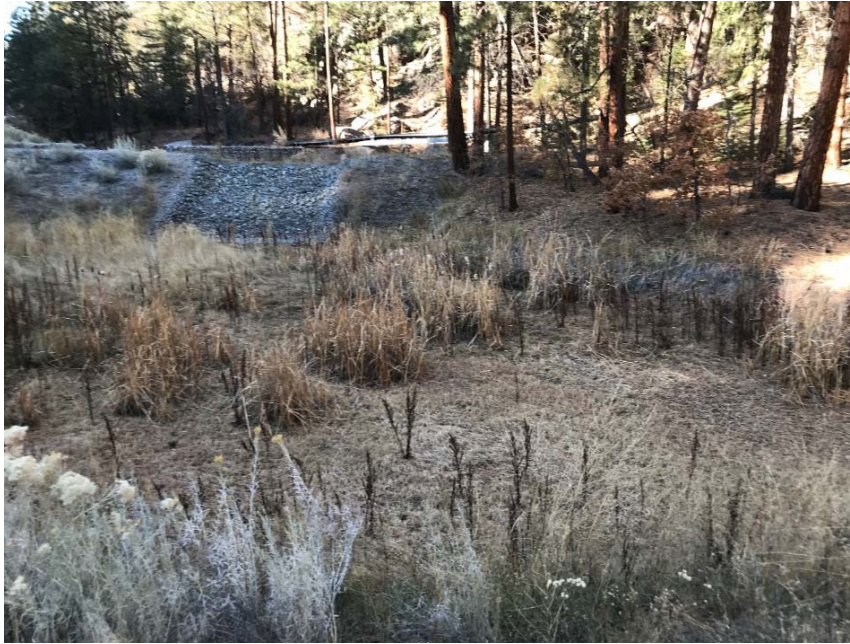
Photo C-3.1-3 November 2019—lower basin. Basin dry. Rodent burrows encountered on south side of basin. Will continue to monitor.
