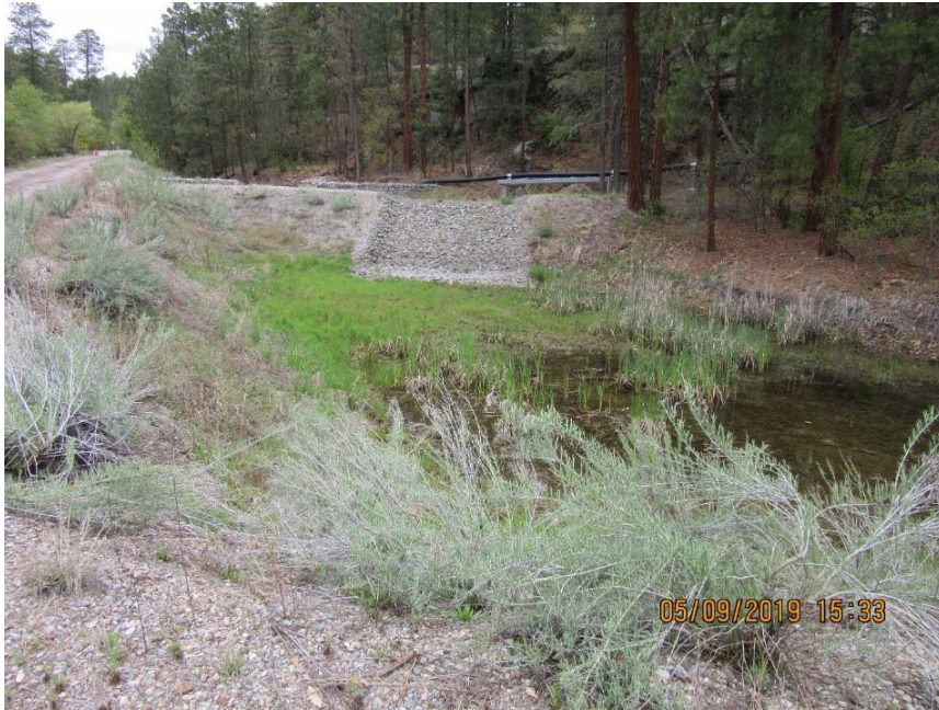
Photo C-3.1-1 May 2019—lower basin. No breaching/slides/cracks/sloughs present on embankment and pond. No erosion occurring on slope. No trash or debris present in control. Recommend pest control along south side of ponds for several rodent burrows.
