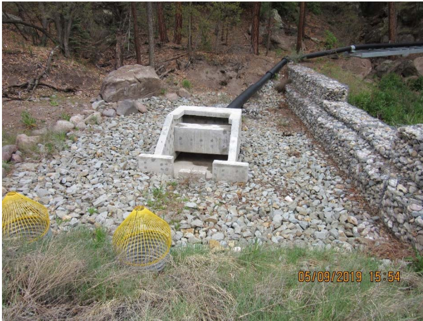
Photo C-3.9-1 May 2019—pipeline outlet, energy dissipater, and gabion overflow structure. Control is operating as designed with no apparent issues to structure.
