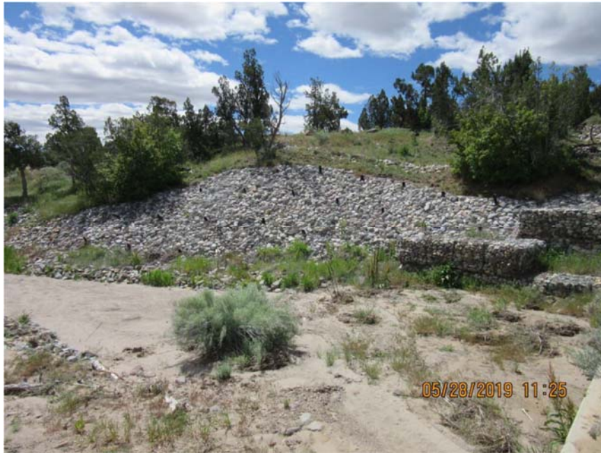
Photo C-5.3-1 May 2019—downstream south embankment and scour-stop, looking south. Control is operating as designed. No buckling of embankment occurring. Riprap functioning as designed. Vegetation established and no evidence of erosion. Minor rodent burrows. Will continue to monitor.
