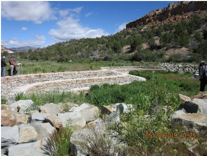
Photo C-6.1-1 May 2019—Redi-Rock block structure, looking north. Redi-Rock structure shows no evidence of displacement or settling. Vegetation well established.
