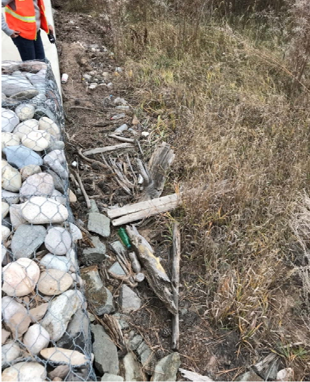
Photo C-2.2-4 November 2019—upstream face of weir. Floatable debris present. Recommend removal of debris.
