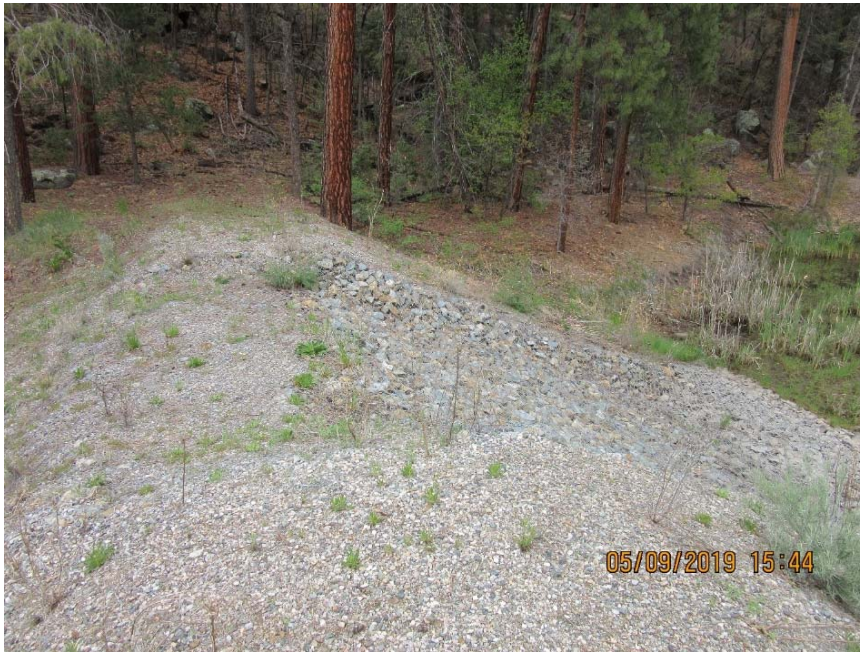
Photo C-3.4-1 May 2019—upper basin spillway. No signs of erosion occurring on or near spillway. Spillway is maintaining alignment and stability.
