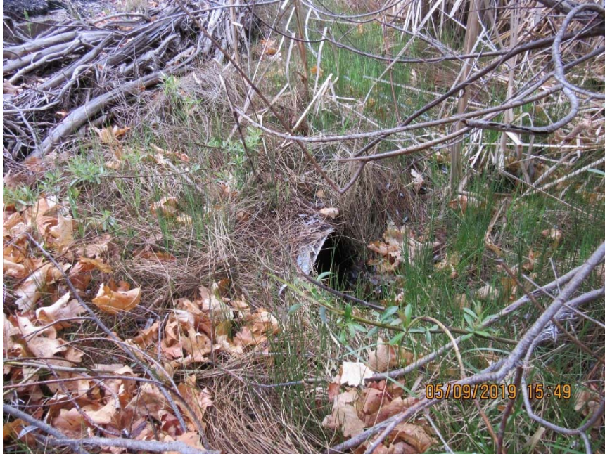
Photo C-3.5-2 May 2019—culvert inlet. Willows and wetland vegetation well established, stable, and clear of trash/debris. No seepage or piping occurring.
