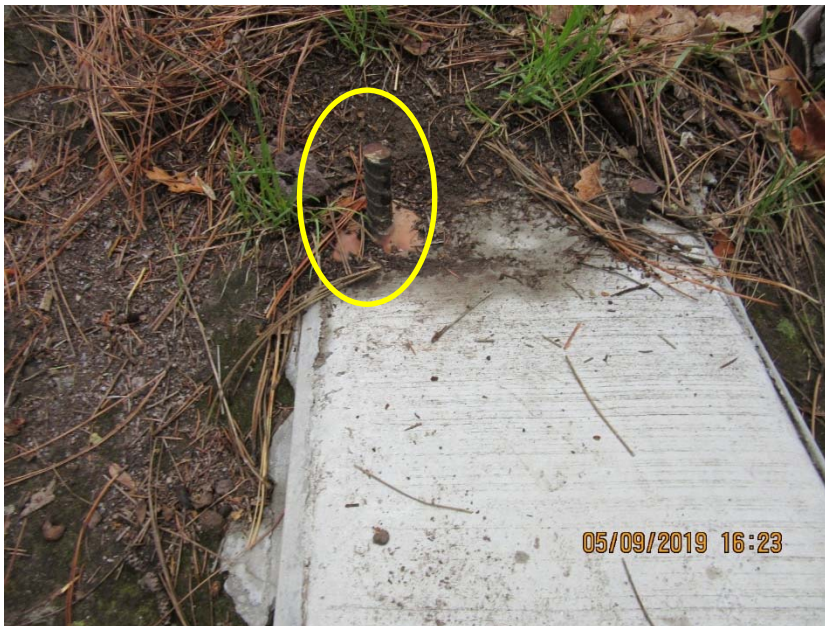
Photo C-3.6-4 May 2019—pipeline headwall. Rebar sticking up on headwall is a tripping hazard. Recommend removal.
