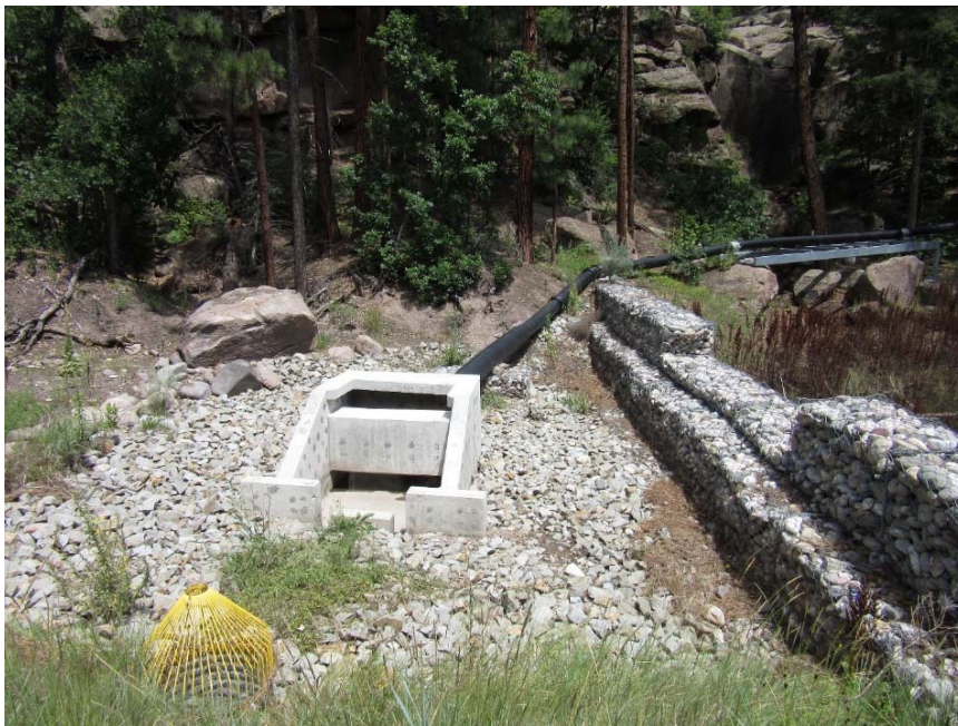
Photo C-3.9-2 Flow event inspection for August 7, 2019, storm event—pipeline outlet, energy dissipater, and gabion overflow structure. Control is operating as designed with no apparent issues to structure.
