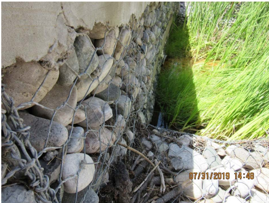
Photo C-2.7-2 Flow event inspection for July 25, 2019, storm event—outlet. Evidence of corrosion noted in 2018. Pond level was at approximately 6 in. above the bottom of the outlet culvert at time of inspection.
