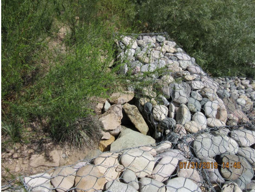
Photo C-2.1-5 Flow event inspection for July 25, 2019, storm event—Erosion occurring at northeast corner of weir was addressed. Area filled with on-site round riprap.
