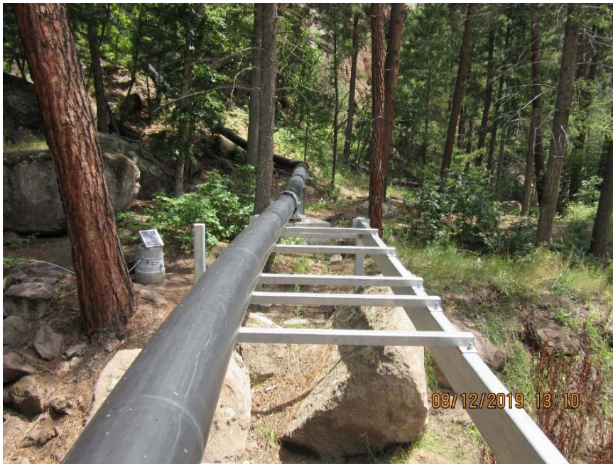
Photo C-3.8-2 Flow event inspection for August 7, 2019, storm event—pipeline bridge structure. Control is operating as designed with no apparent issues to structure.
