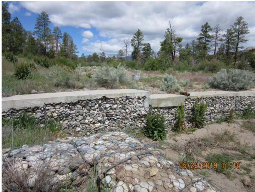
Photo C-5.1-1 May 2019—south embankment, looking west. Well-established vegetation on embankment. No signs of erosion or undermining.
