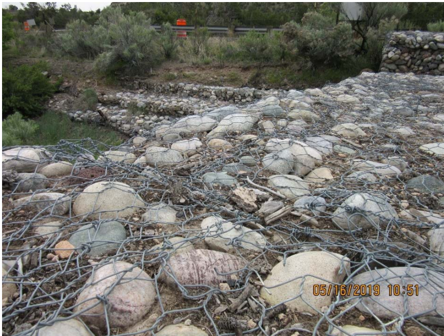
Photo C-4.7-3 May 2019—broken gabions on south end of crest. Recommend repair of holes in gabion basket.
