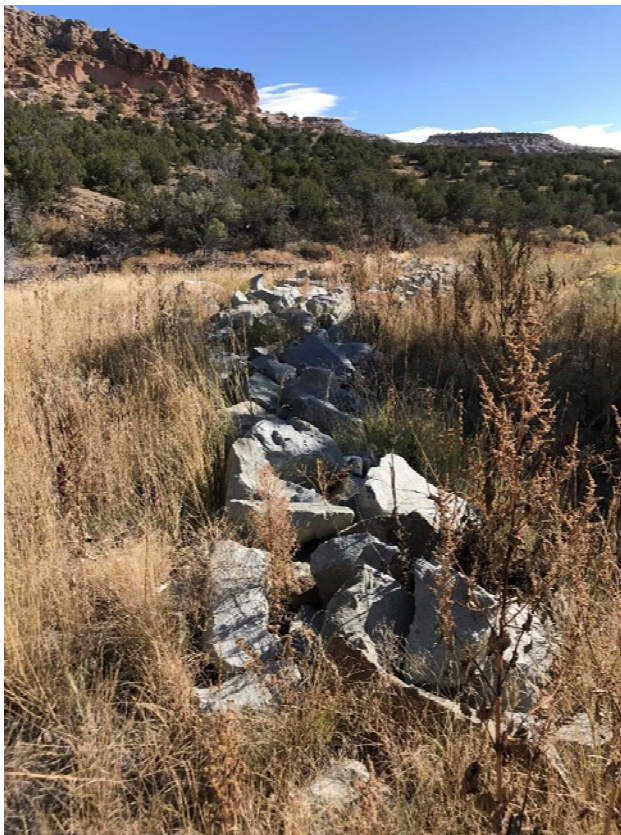
Photo C-6.4-2 October 2019—south-bank berm, looking northeast. Berm is stable; no noted erosion or breaching/slides/cracks to berm.
