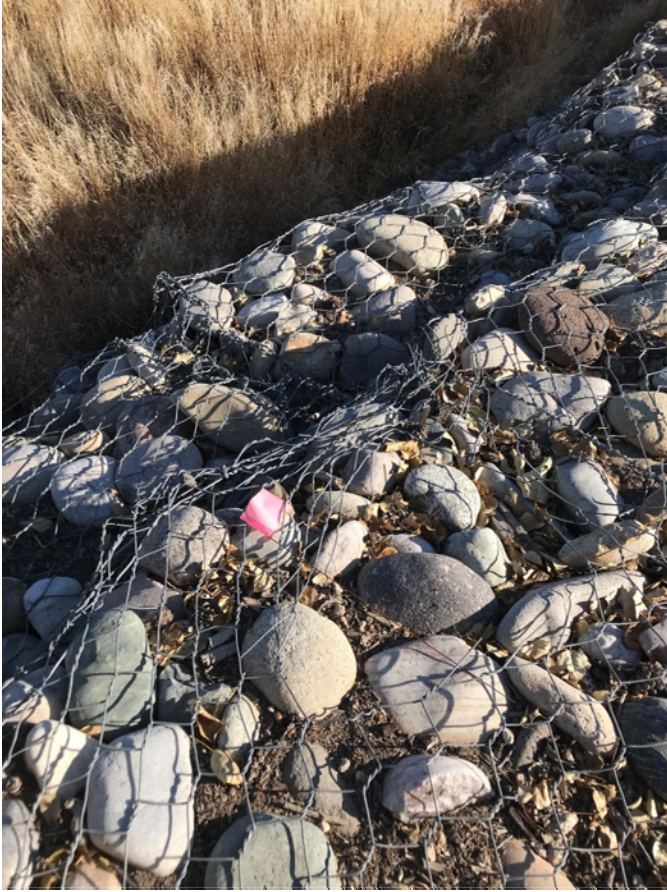
Photo C-4.7-8 November 2019—broken gabion wires on north end of weir crest. Recommend repair.
