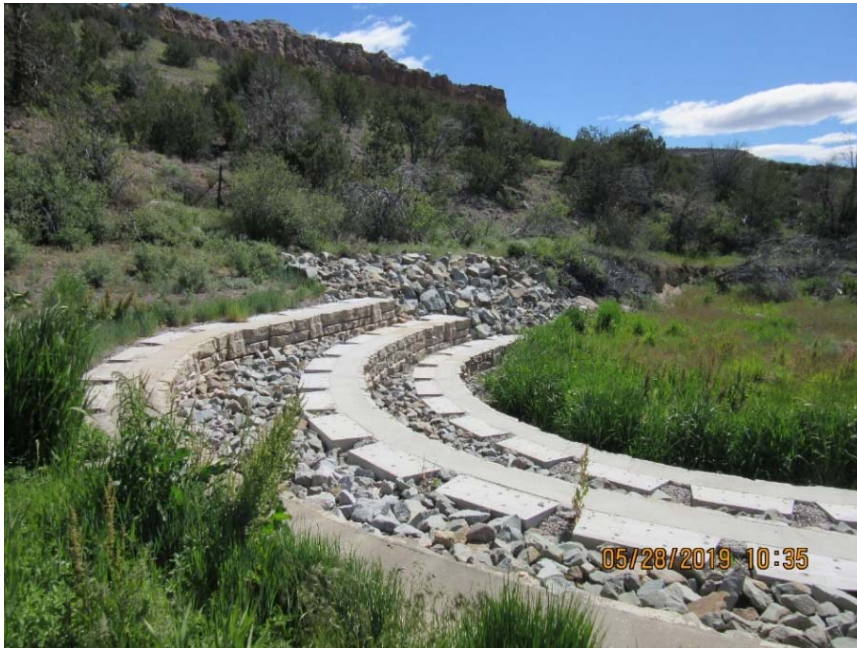
Photo C-6.2-1 May 2019—wetland north bank, looking northeast. Slope is stable with no evidence of erosion where riprap is located. Structure is functioning as designed with established vegetation.
