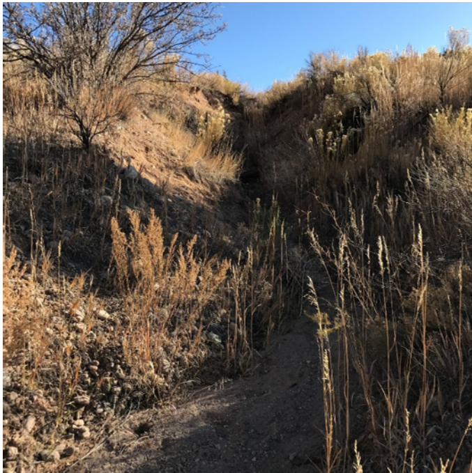
Photo C-4.11-10 November 2019—borrow pit. Damage on north end is not resolved by Los Alamos County. Recommend notification to Los Alamos County to have berm and TRM damage repaired.
