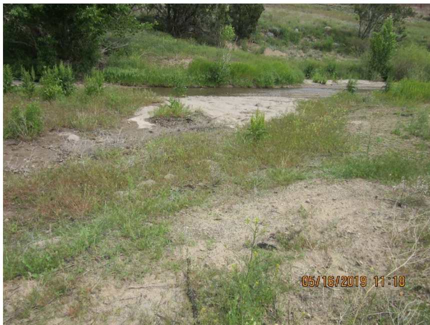
Photo C-4.5-1 May 2019—Los Alamos Pond 2 (middle) looking downstream. Pond appears to have been breached. Minor ponding on the south side of channel. Pond has no capacity to retain sediment.
