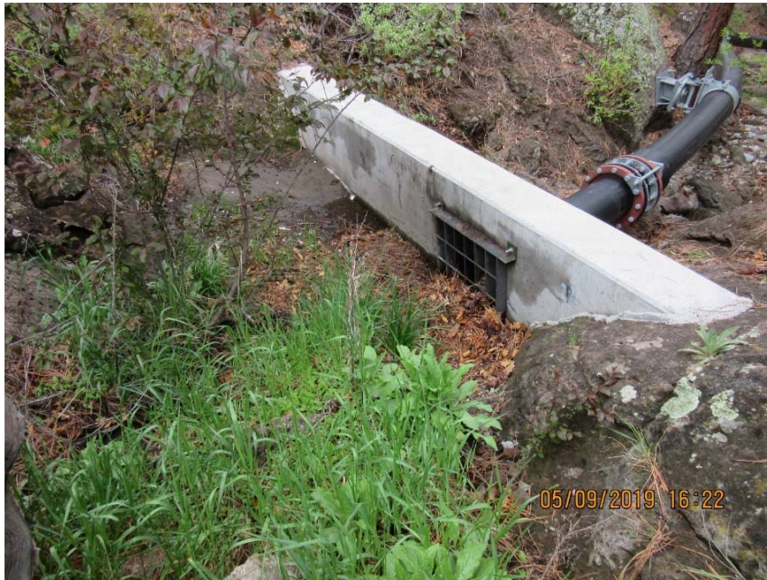
Photo C-3.6-1 May 2019—pipeline headwall. Headwall functioning as designed. Needlecast is blocking portion of pipe inlet grate. Recommend maintenance to remove needlecast.
