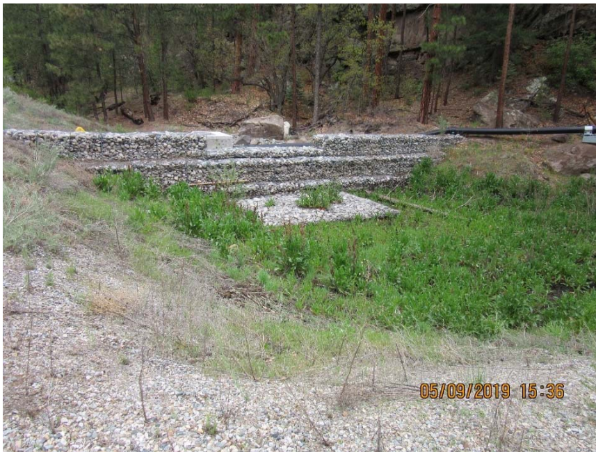
Photo C-3.2-1 May 2019—upper basin. No breaching, slides, cracks, or sloughs present on embankment and pond. No erosion occurring on slope. No trash or debris present in control. Recommend pest control along south side of ponds for several rodent burrows. Recommend removal of fallen tree in pond.
