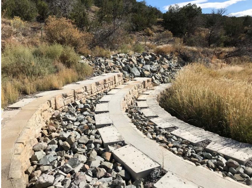
Photo C-6.2-2 October 2019—wetland north bank, looking northeast. Slope is stable with no evidence of erosion where riprap is located. Structure is functioning as designed with established vegetation.
