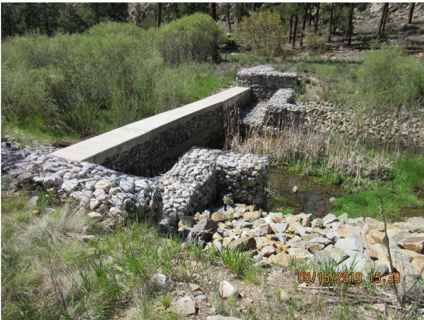
Photo C-2.3-1 May 2019—weir structure looking upstream. No deteriorated joints present on upslope side of weir. Gabion basket is structurally intact and in stable condition.
