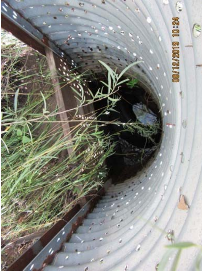
Photo C-2.5-4 Flow event inspection for August 7, 2019, storm event—standpipe. Sediment level at approximately 6 in. below top of wood board stop.
