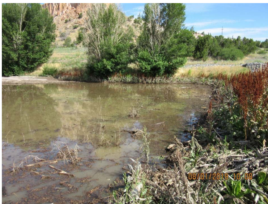
Photo C-4.6-2 Flow event inspection for July 26, 2019, storm event—Los Alamos Pond 3 (lower). Pond level approximately 0.5-ft deep in lower pond. Tadpoles noted. Approximately 0.5 ft sediment deposition upstream of pond. High flows on north side of pond; low flows at south side of pond. Will continue to monitor.
