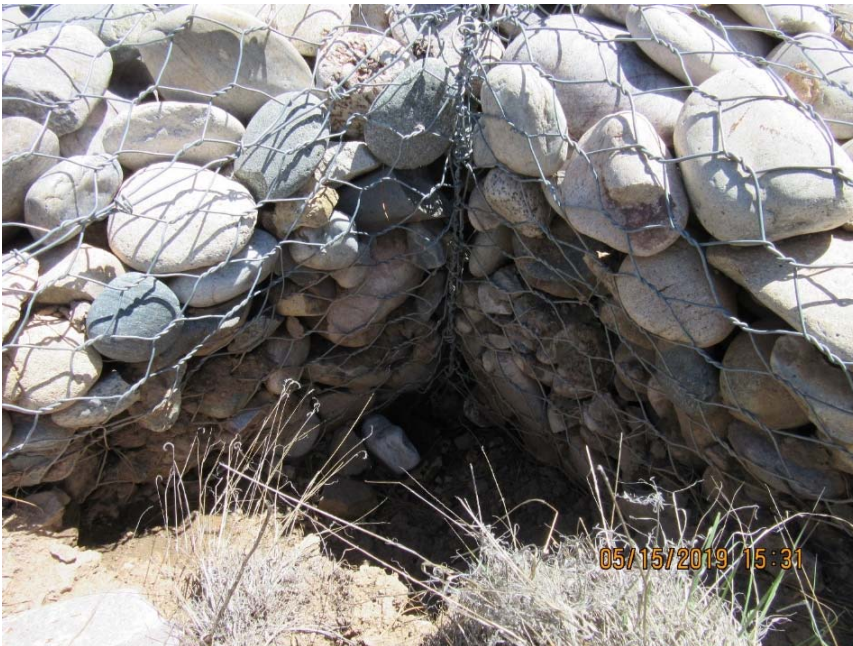
Photo C-2.1-4 May 2019—Erosion occurring at northeast corner of weir. Recommend filling hole with on-site round riprap.
