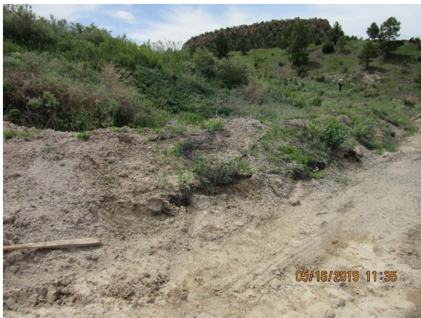
Photo C-4.11-3 May 2019—Berm and TRM damage (north end) occurred during nearby Los Alamos County well construction. If additional sediment is brought in, the recommendation is to increase the entire berm height.
