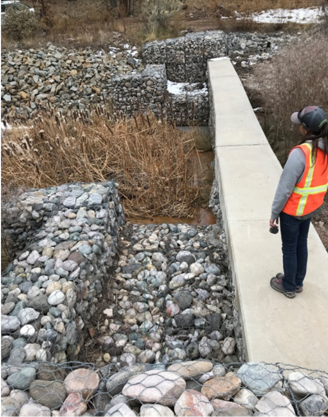
Photo C-2.4-2 November 2019—downstream face of weir. No significant change since last inspection.
