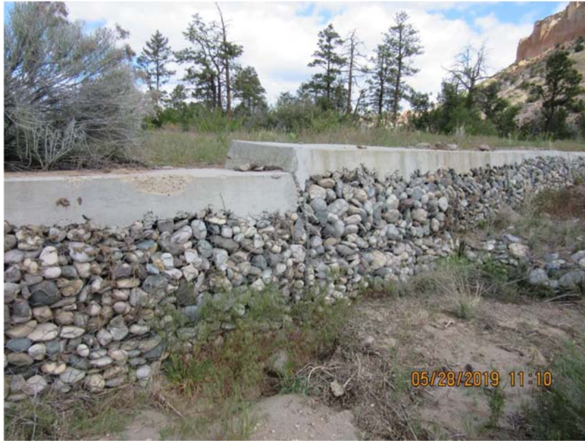
Photo C-5.4-3 May 2019—weir spillway and flow-way, looking west. Minor spalling/chipping of concrete on downstream side of the spillway. Will continue to monitor.
