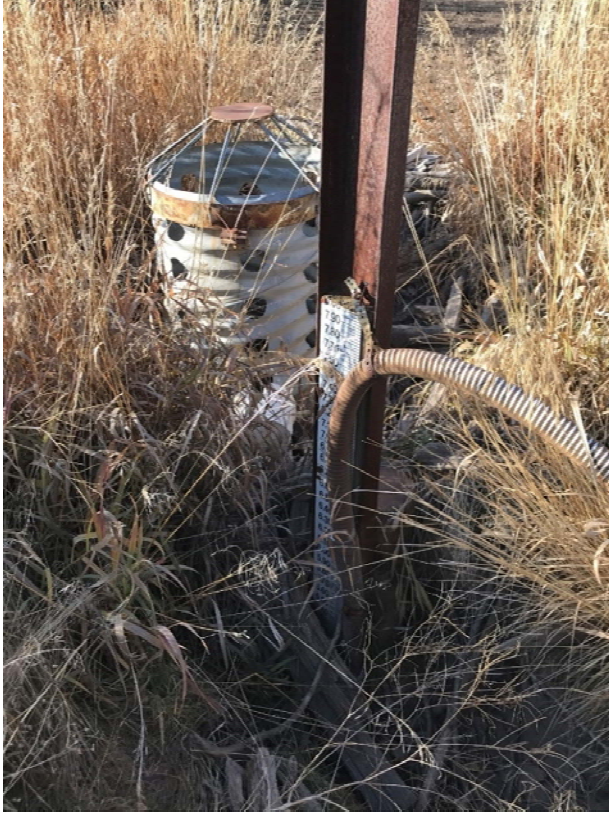
Photo C-4.9-4 November 2019—standpipe. Sediment and debris level at 4.6 ft on gage.
