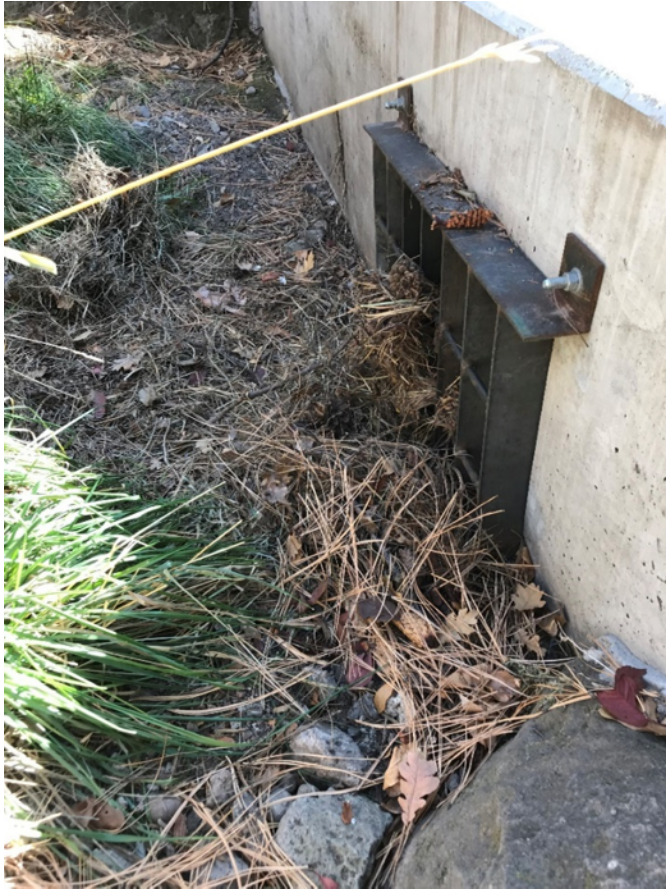
Photo C-3.6-3 November 2019—pipeline headwall. Needlecast debris at trash rack blocking inlet. Blockage removed. Recommend replacement of trash rack with one that is not in line with the pipe inlet.
