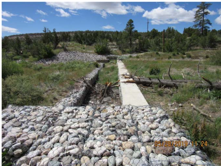
Photo C-5.4-1 May 2019—weir crest and flow-way, looking south. Cracks in concrete are apparent where overflow weir intersects the spillway (both corners of the spillway). Alignment is fine. There appears to be a twisting of the overflow concrete weir and spillway crests as a result of gabion movement/settling. Will continue to monitor.
