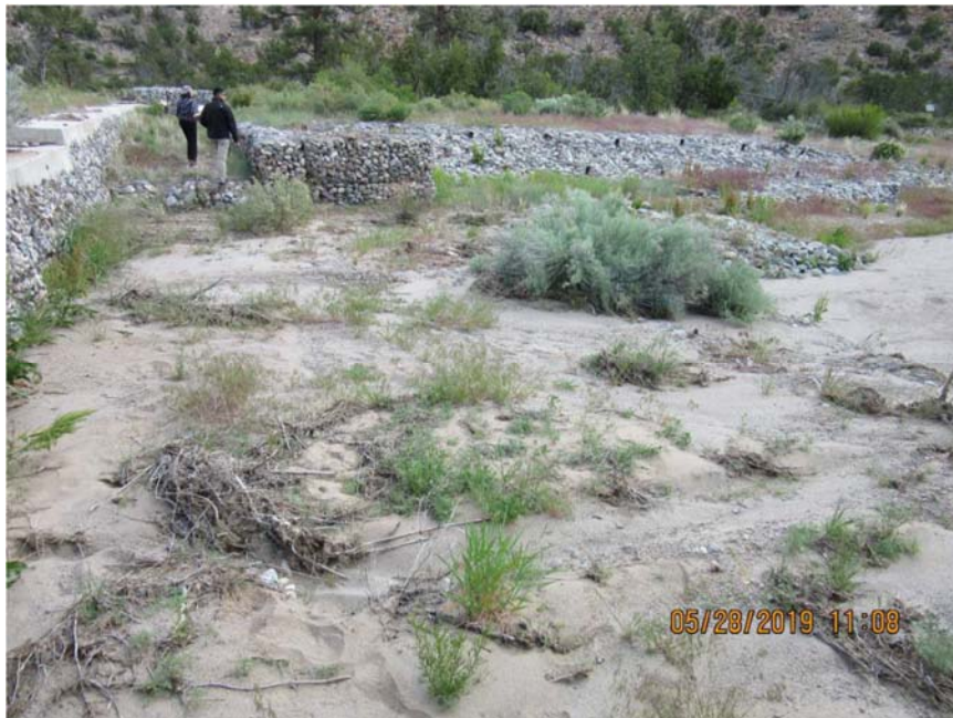
Photo C-5.3-2 May 2019—downstream north embankment and scour-stop, looking north. Control is operating as designed. No buckling of embankment occurring. Riprap functioning as designed. Vegetation established and no evidence of erosion. Minor rodent burrows. Will continue to monitor.
