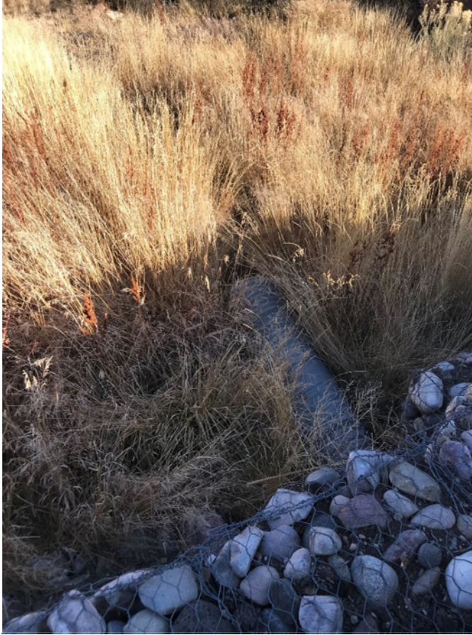
Photo C-4.10-3 November 2019—weir outlet. Erosion occurring in sediments deposited on top of gabion mattress. Erosion is resolved before end of gabion mattress apron. Sediment deposits on top of gabion mattress apron are approximately 1 in. below bottom of outlet invert.
