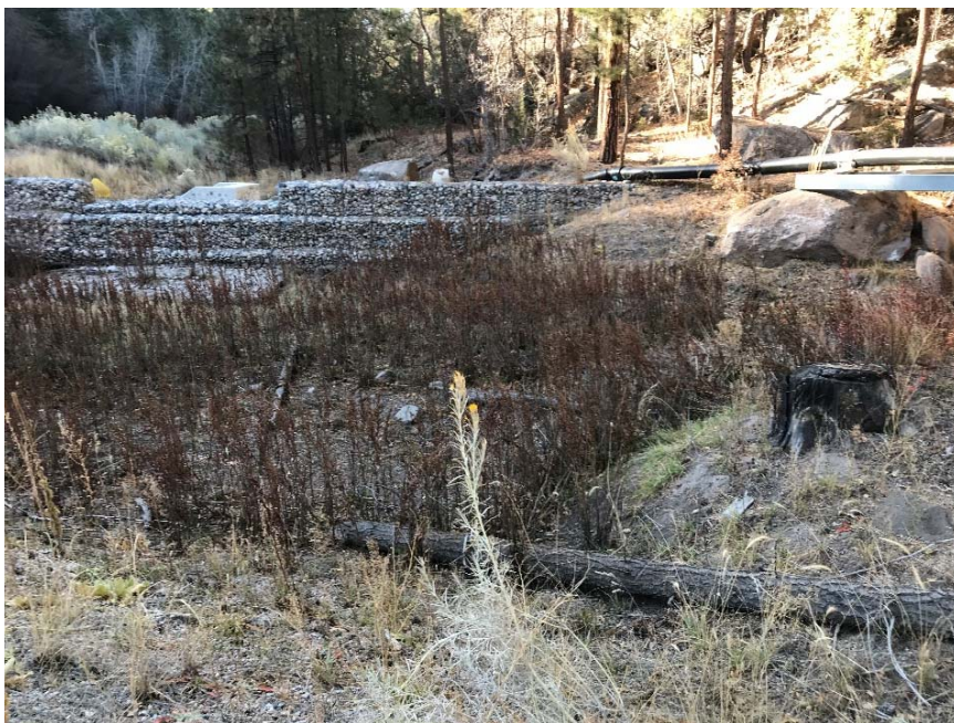
Photo C-3.2-3 November 2019—upper basin. Basin dry. No erosion occurring on slope. Sloughing on south side of basin, above where TRM was installed. Sides are retained by concrete jersey barrier at edge of road. Rodent burrows encountered on south side of basin, above where TRM was installed. Fallen tree in basin. Will continue to monitor.
