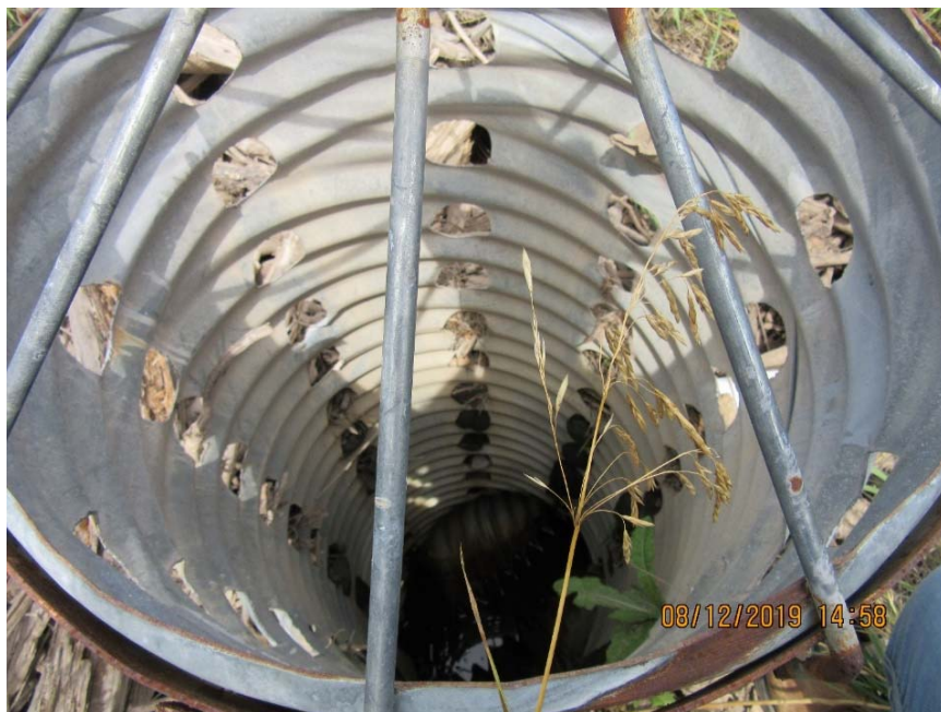
Photo C-4.9-3 Flow event inspection for August 7, 2019, storm event—standpipe. Sediment upstream of weir at 4.7-ft depth and debris at 6-ft depth. Approximately 3 ft of standpipe exposed. No significant change since last inspection.
