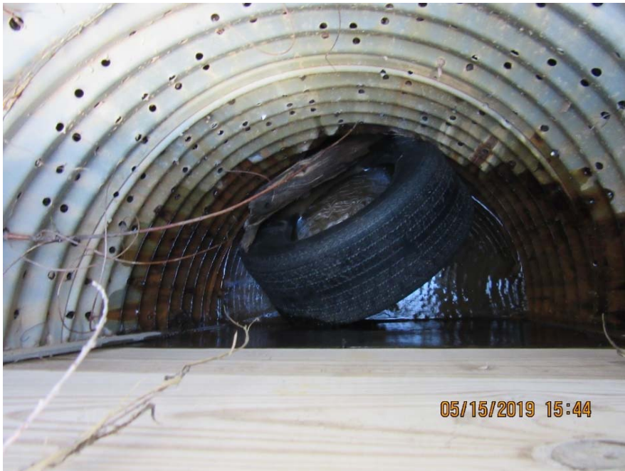
Photo C-2.5-2 May 2019—standpipe. Tire is present within standpipe. No action recommended.
