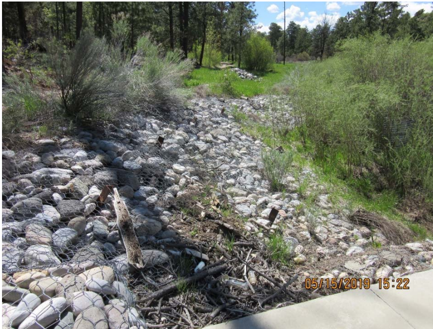
Photo C-2.1-1 May 2019—Embankment is stable and operating as designed. Well-established vegetation with no erosion occurring from hillslope. Some trash and debris present.
