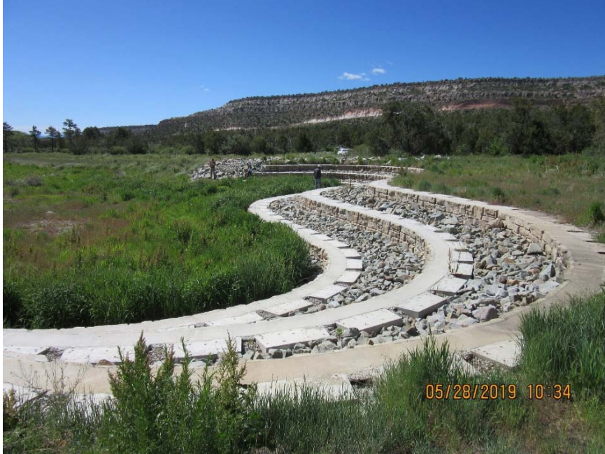
Photo C-6.1-2 May 2019—Redi-Rock block structure, looking southeast. Redi-Rock structure shows no evidence of displacement or settling. Vegetation well established.
