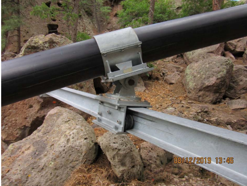
Photo C-3.6-9 Flow event inspection for August 7, 2019, storm event—Castor gouging due to skewed support on beam trolley support 15, south side. Continue to monitor.
