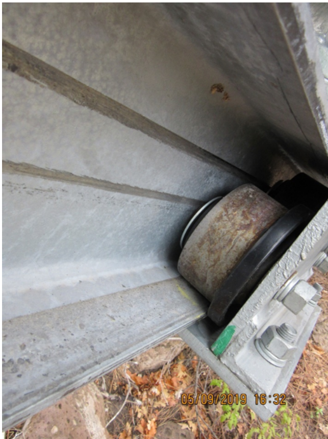
Photo C-3.6-6 May 2019—Trolley flanged wheels on beam trolley supports are gouging the I-beam supports. Noted deterioration of coating on trolley flanged wheels. Recommend further investigation.
