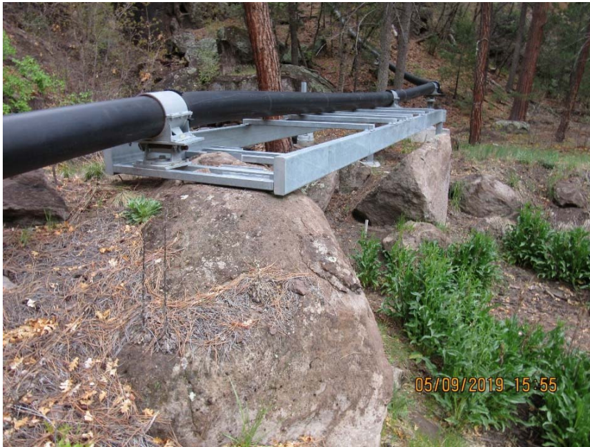
Photo C-3.8-1 May 2019—pipeline bridge structure. Control is operating as designed with no apparent issues to structure.
