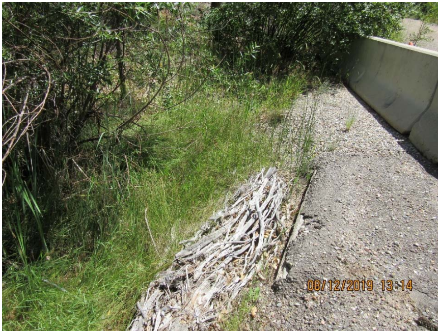
Photo C-3.5-3 Flow event inspection for August 7, 2019, storm event—Culvert inlet is covered with branches.
