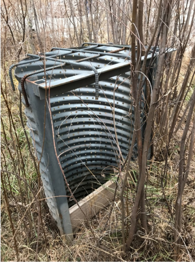
Photo C-2.5-5 November 2019—standpipe. Sediment level is approximately 1 ft below wood board stop. Tire is present within standpipe. No action recommended.
