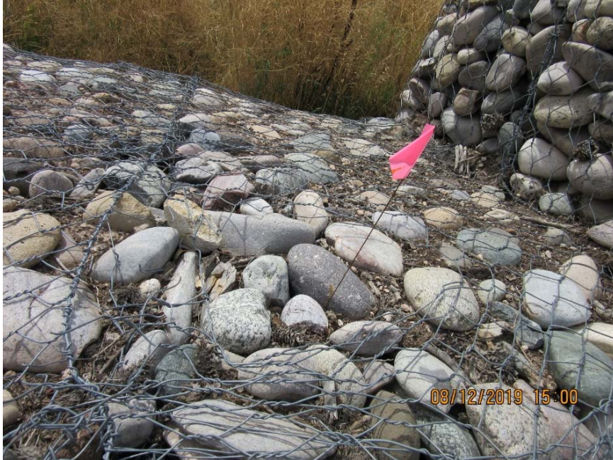
Photo C-4.7-6 Flow event inspection for August 7, 2019, storm event—broken gabion wires on north end of weir crest. Recommend repair.
