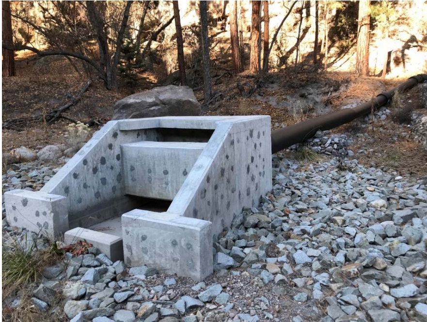
Photo C-3.9-3 November 2019—pipeline outlet, energy dissipater, and gabion overflow structure. Control is operating as designed with no apparent issues to structure.
