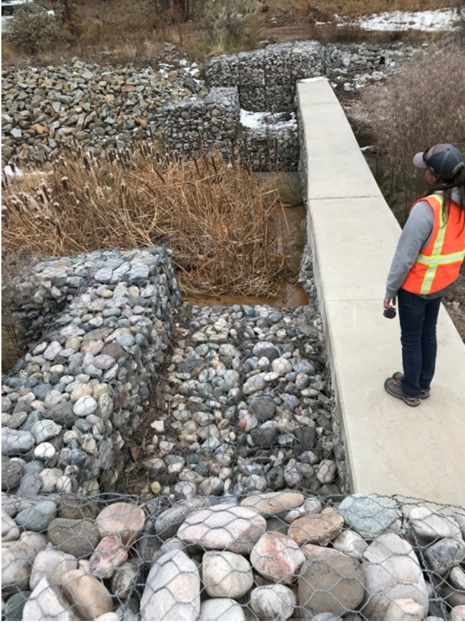
Photo C-2.6-3 November 2019—spillway alignment. Spillway operating as designed. No sign of improper alignment, deterioration, or trash/debris.
