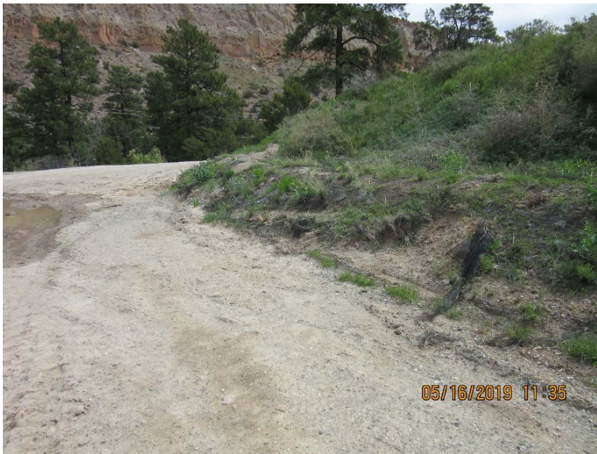
Photo C-4.11-2 May 2019—Berm and TRM damage (north end) occurred during nearby Los Alamos County well construction. If additional sediment is brought in, the recommendation is to increase the entire berm height.
