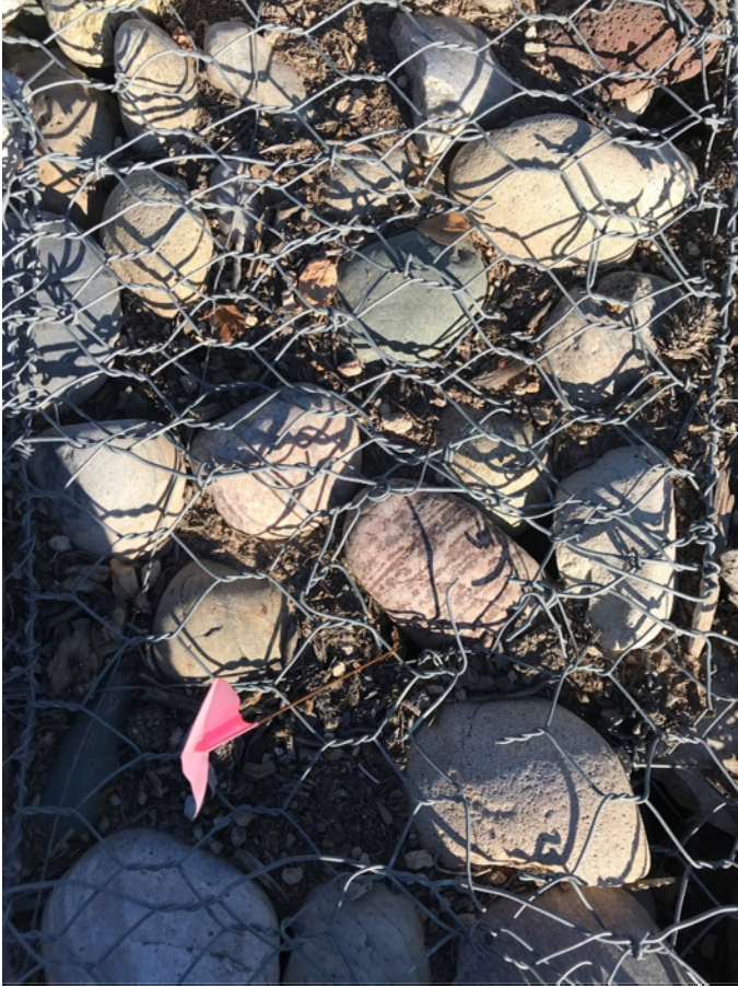
Photo C-4.7-9 November 2019—broken gabion wires on south end of weir crest. Recommend repair.
