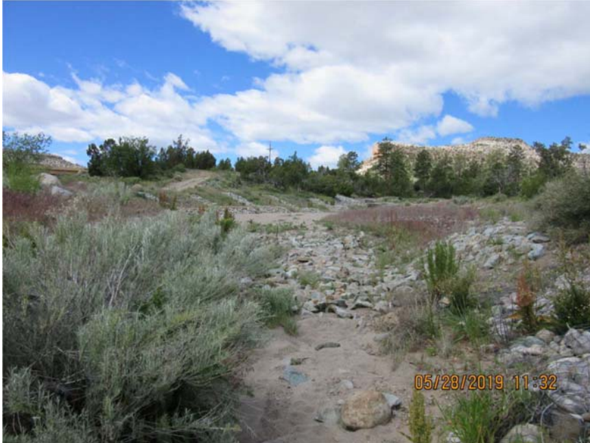
Photo C-5.5-2 May 2019—Redi-Rock spurs, looking west. Medium size (12-in. nominal diameter) rocks deposited upstream of flow gage. Will continue to monitor.
