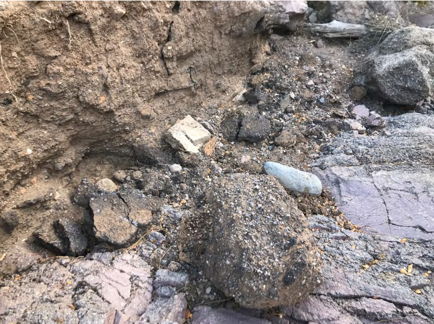
Figure 4.2-4 Example of asphalt in the soil in the drainage channel before removal. Asphalt pieces ranged in size from 0.5 ft to several feet in diameter.
