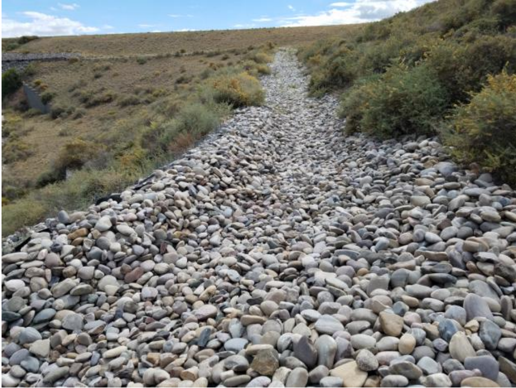
Picture 18. Eastern Berm on Sideslope East of Landfill
