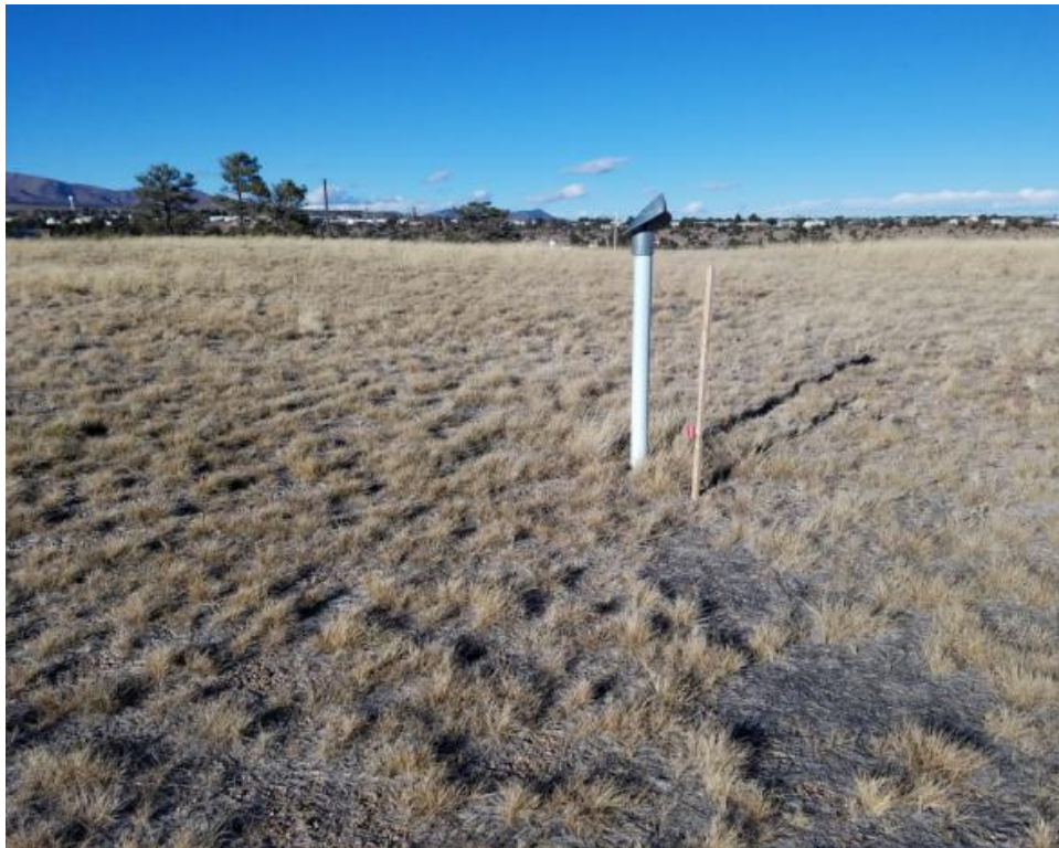
Picture 4. Methane Monitoring Port - North Slope of Landfill
