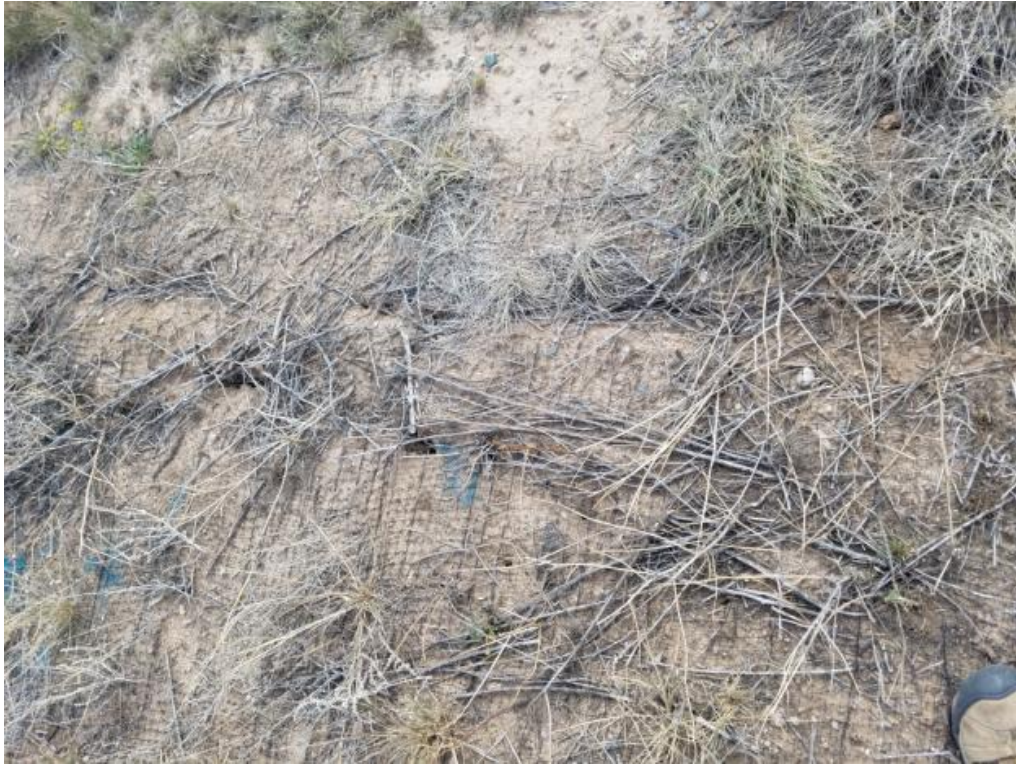
Picture 28. Tension Cracking near Top of Side Slope of Older Landfill Cover, North of ET Cover
