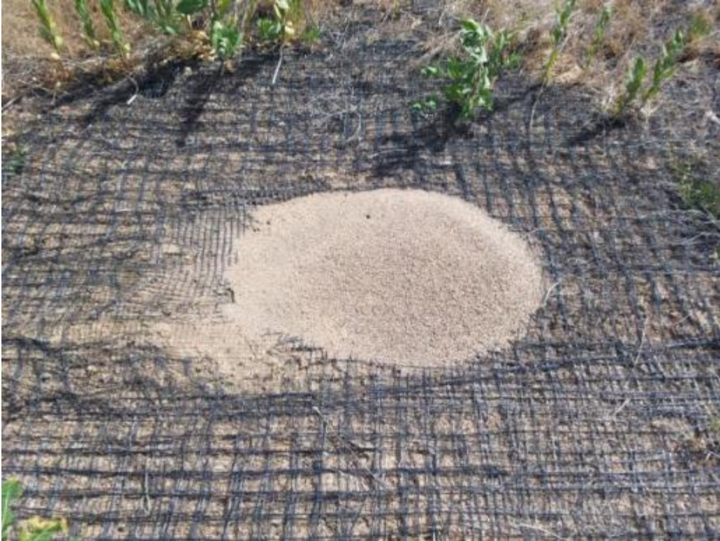
Picture 19. Biointrusion (Ant Hill) in Older Landfill Side Slope, North of ET Cover
