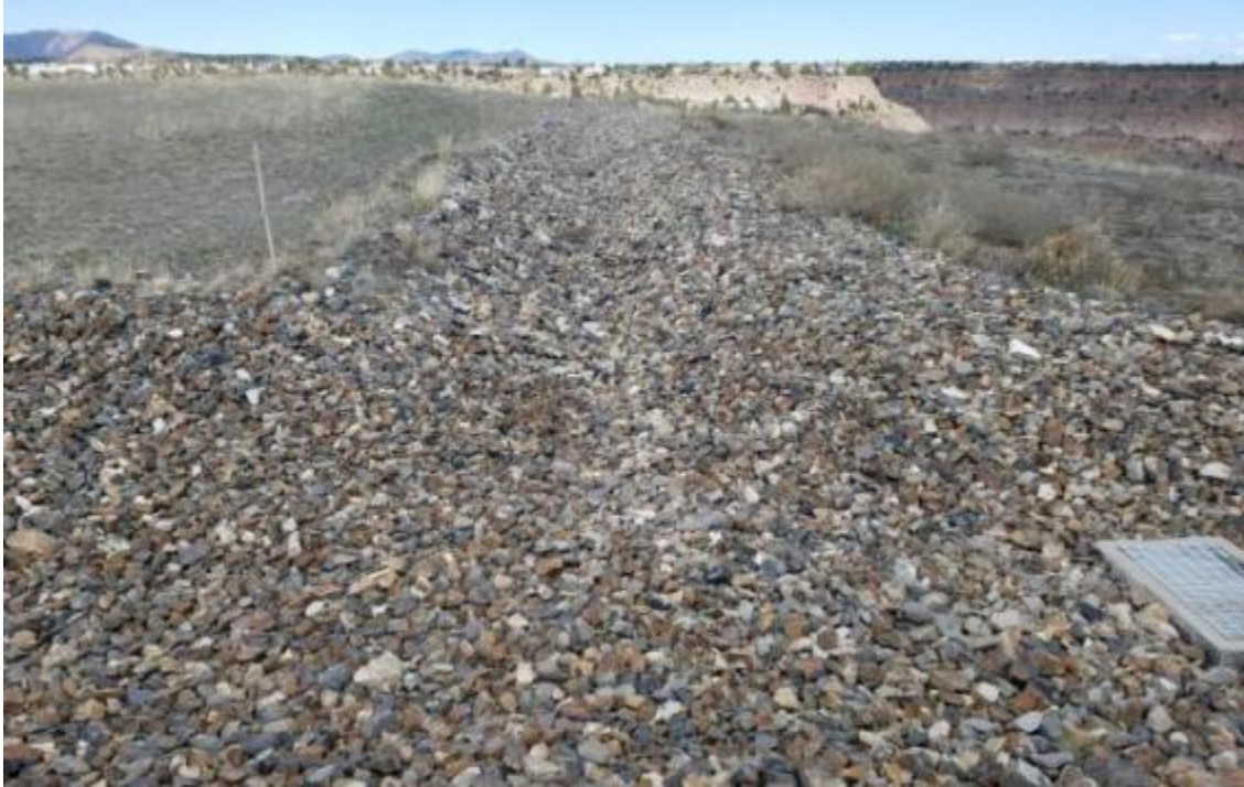
Picture 11. Drainage Channel - East Perimeter of ET Cover
