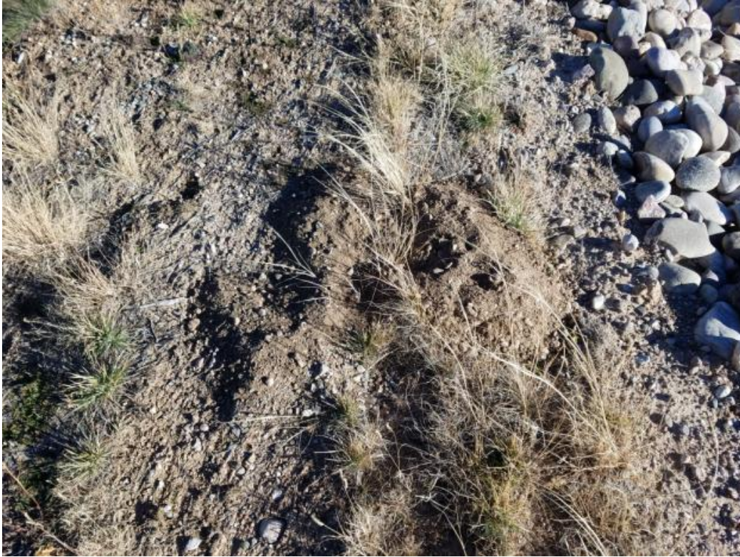
Picture 19. Biointrusion in Older Landfill Side Slope, North of ET Cover
