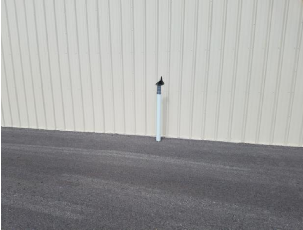
Picture 2. Methane Monitoring Port - West of Landfill, South of New Hangar
