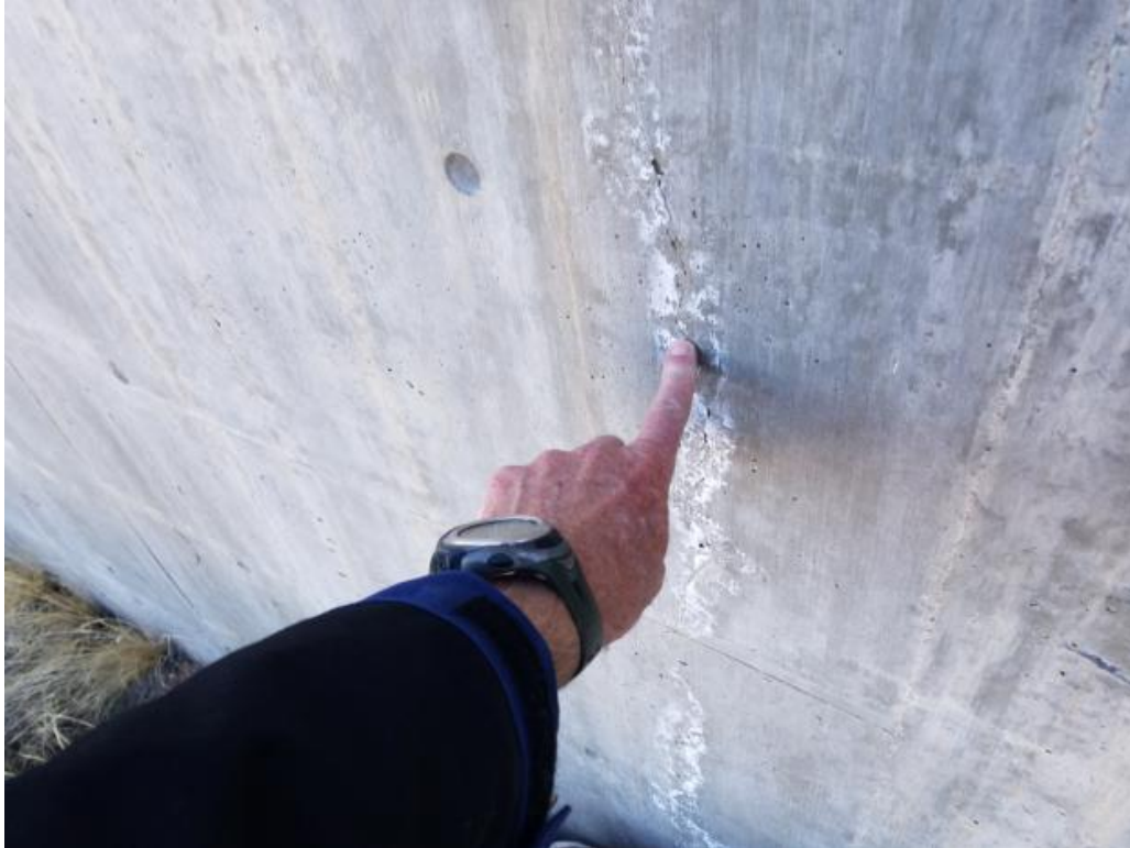
Picture 24. Small Crack in Concrete Retaining Wall - East End of Landfill
