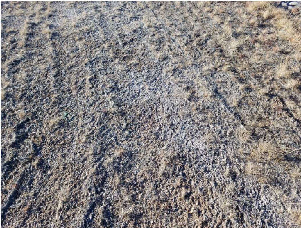
Picture 28. Light Colored Precipitate on Cover Surface (NE Corner)
