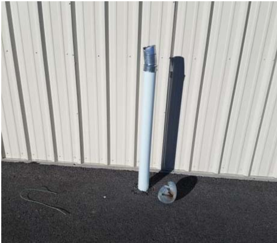
Picture 2. Methane Monitoring Port - West of Landfill, South of New Hangar
