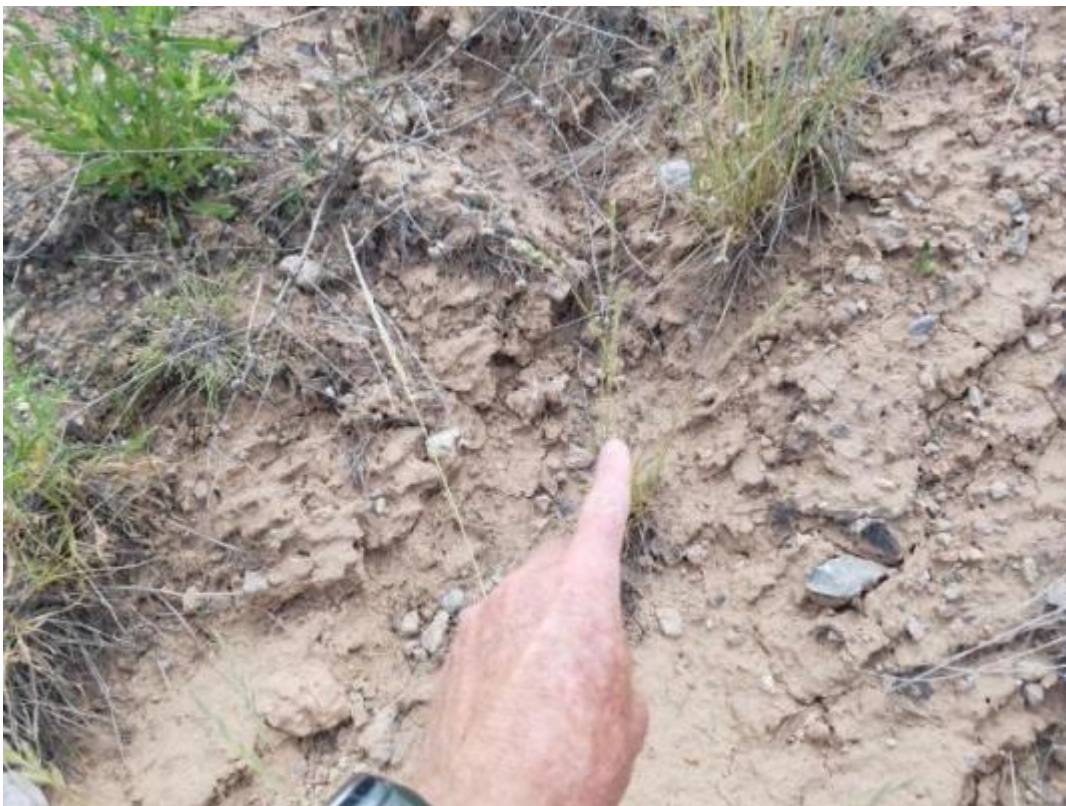
Picture 26. Rill Erosion, Base of East Slope @ End of Landfill
