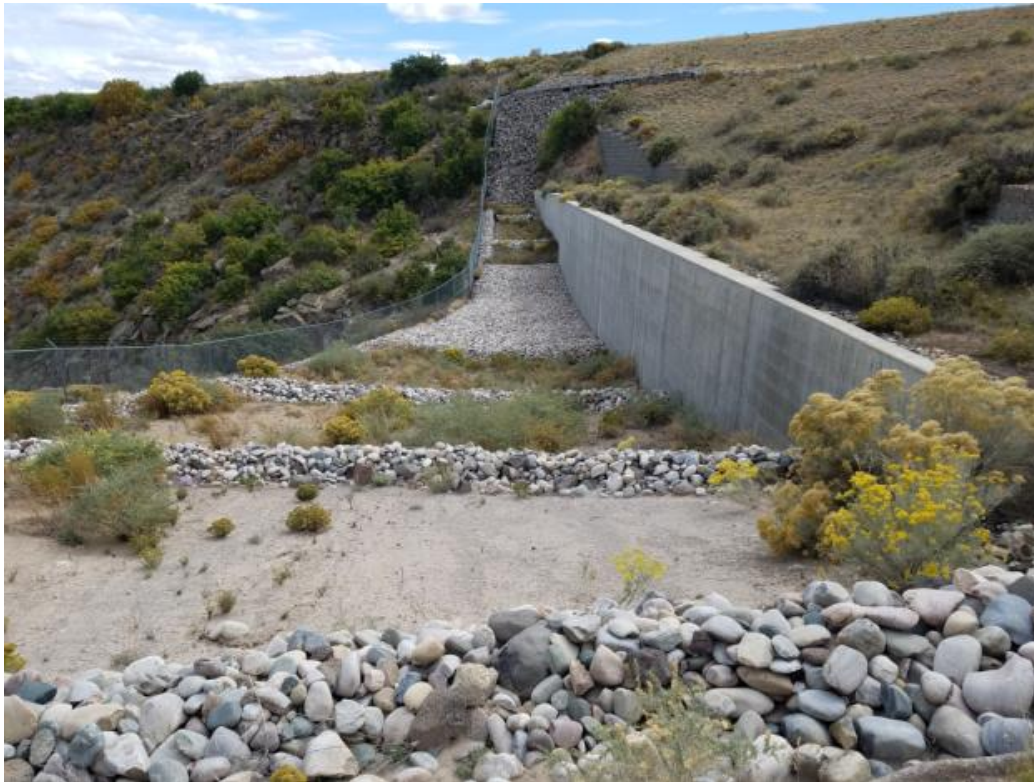
Picture 25. Erosion Control below Concrete Retaining Wall - NE End of Landfill
