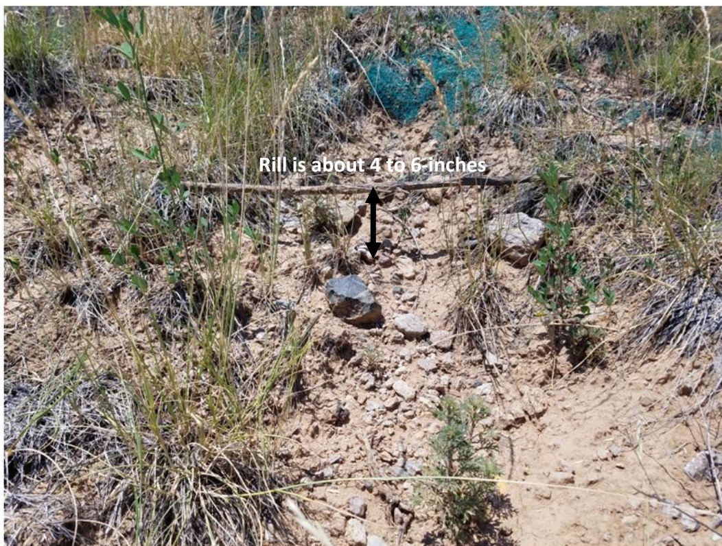
Picture 1. New Rill Erosion noted at Base of Eastern Landfill Slope
