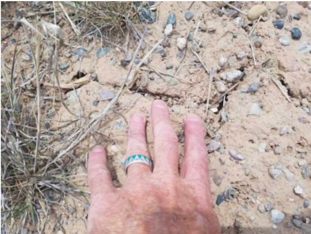
Picture 28. Tension Cracking in Surface of ET Cover
