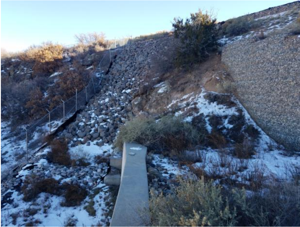
Picture 23. Large Rip Rap Slope and Gabion Retainment Wall - East End of Landfill Site
