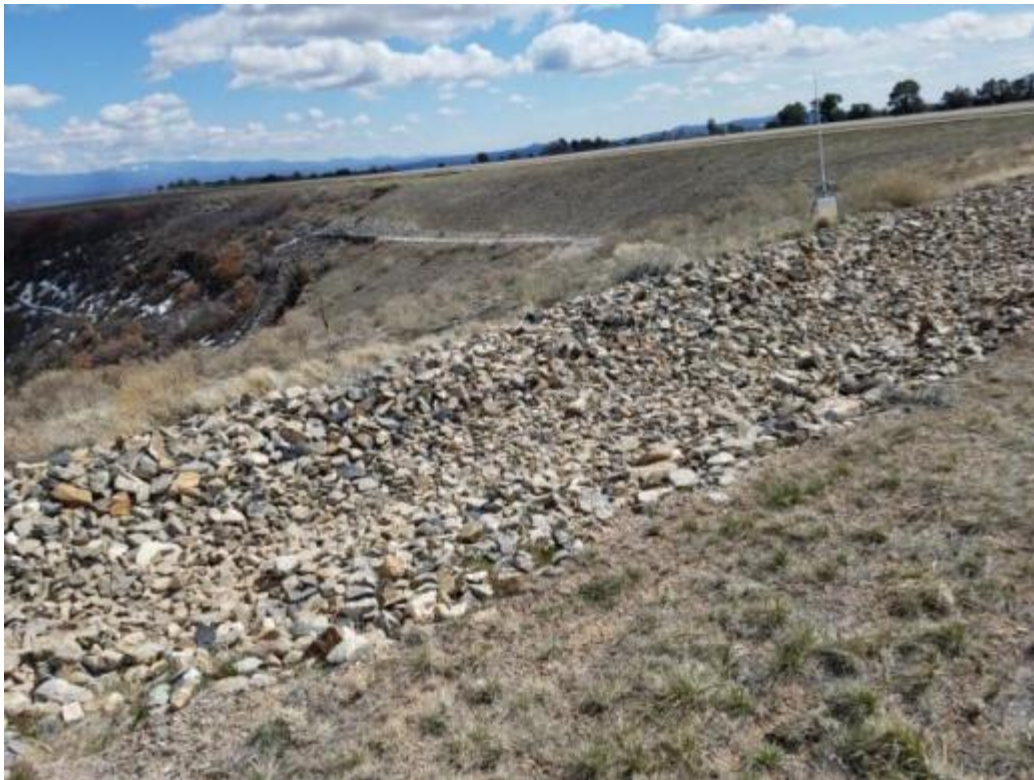
Picture 26. Side Slopes and Erosion Control, East End of Landfill
