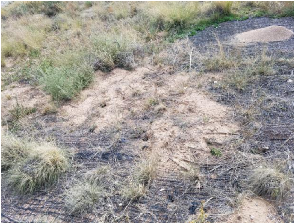
Picture 19. Biointrusion in Older Landfill Side Slope, East of ET Cover
