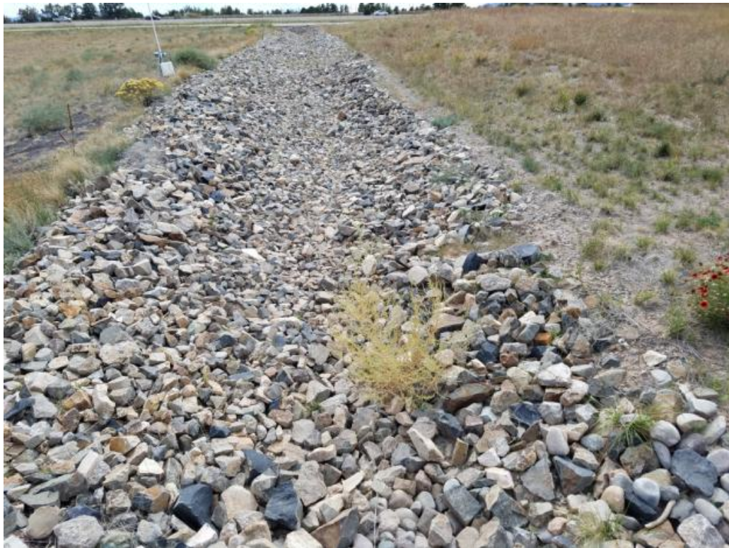
Picture 11. Drainage Channel - East Perimeter of ET Cover
