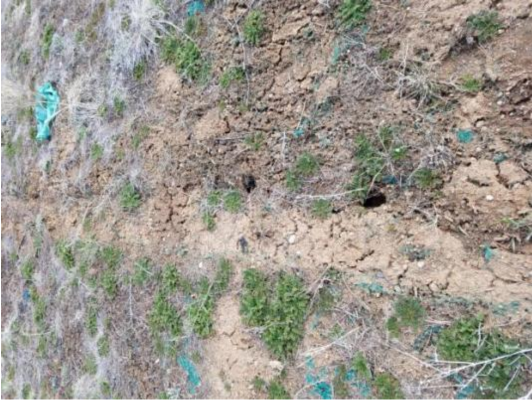
Picture 29. Crack near Top of Side Slope of Older Landfill Cover, North of ET Cover
