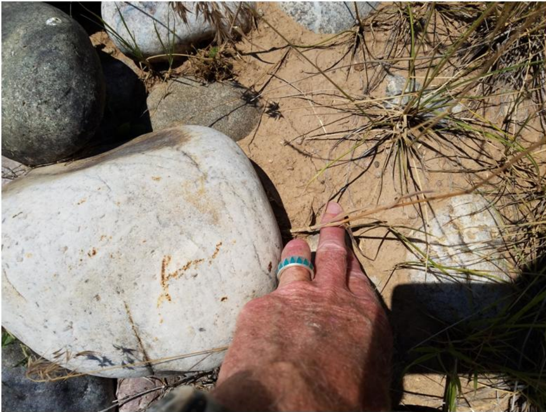
Picture 3. Sediment in Riprap at Base of Slope
