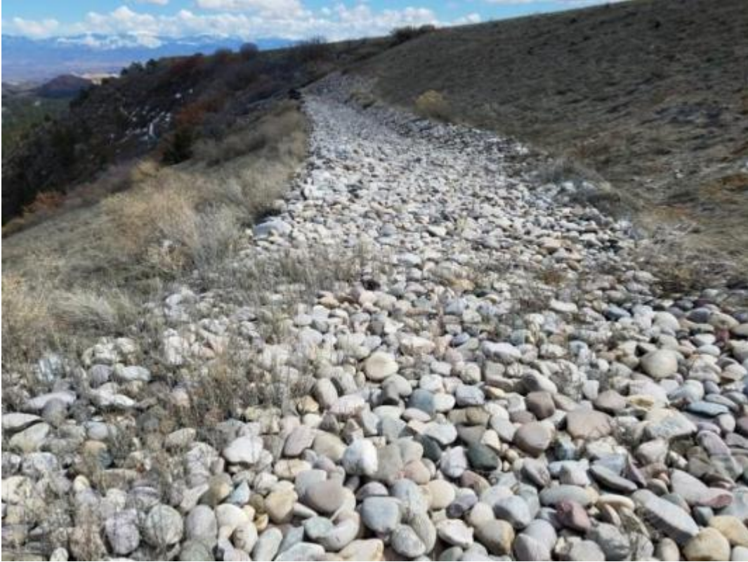
Picture 21. Sideslope Berm East of Landfill
