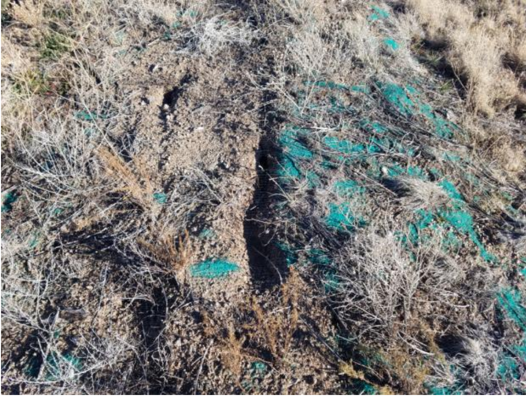
Picture 29. Tension Cracking near Top of Side Slope of Older Landfill Cover, North of ET Cover
