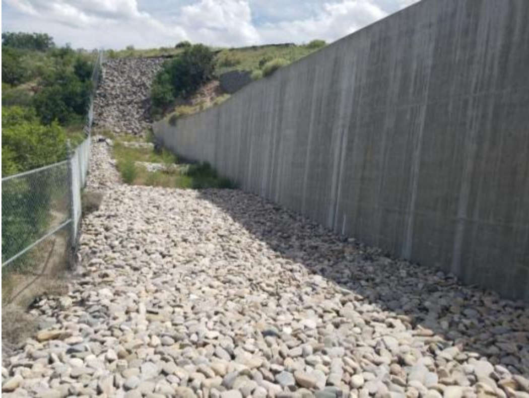
Picture 23. Large Rip Rap Slope and Concrete Retainment Wall - East End of Landfill Site
