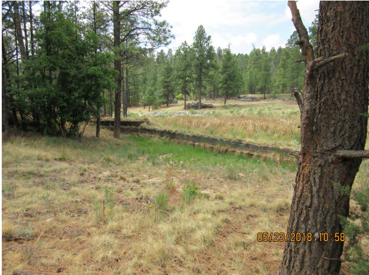
Figure E-3.8-2 May 2018: Lower defense cell barrier with approximately 3.5 ft of capacity available from bottom of pond to spillway
