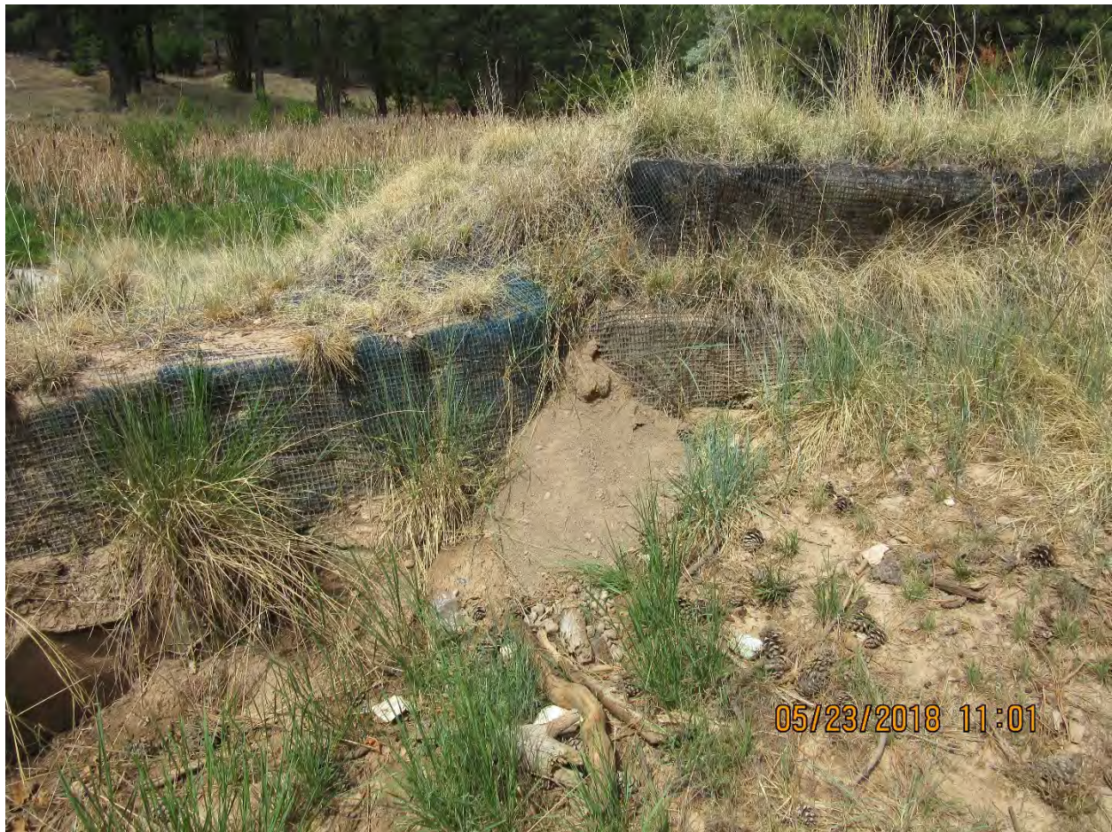
Figure E-3.8-1 May 2018: Lower defense cell. Need to monitor erosion occurring at the west end of the spillway. Investigate need for possible maintenance to address erosion occurring under the turf-reinforcement mat on spillway rundowns.
