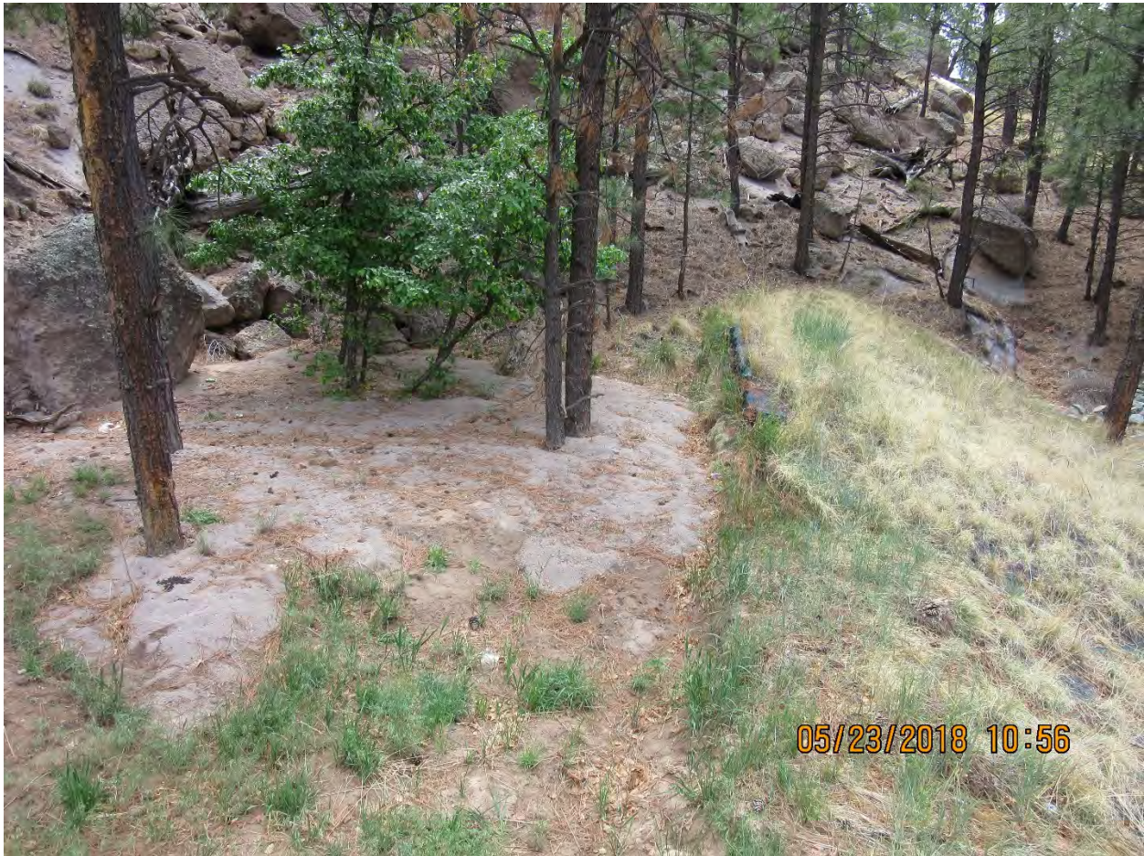
Figure E-3.7-1 May 2018: Upper defense cell sediment migration has recently occurred. There is approximately 1 ft of capacity from the bottom of the pond to the spillway.
