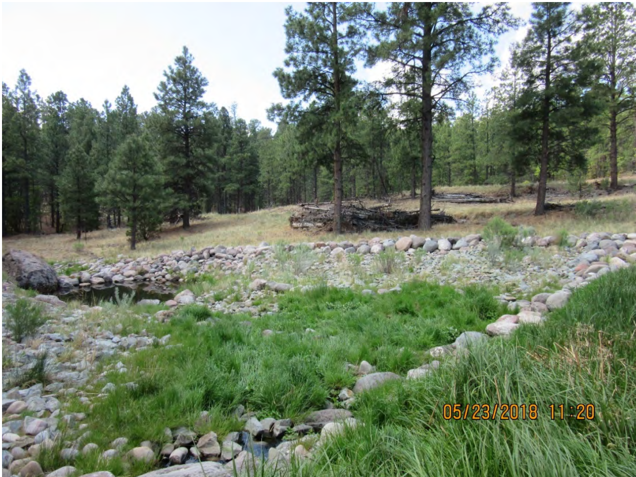
Figure E-3.5-1 May 2018: Lower wetland looking downstream. There is slight vegetation establishment in riprap. The structure is working as designed with no evidence of channelization.
