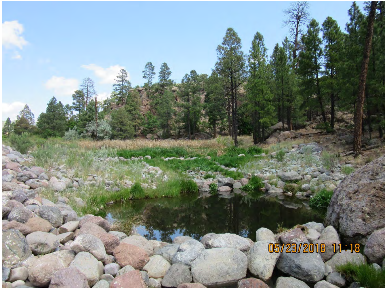
Figure E-3.6-1 May 2018: Cascade structure (looking downstream) working as designed. There is no evidence of rock displacement. There is no evidence of erosion in/near cascade pool.
