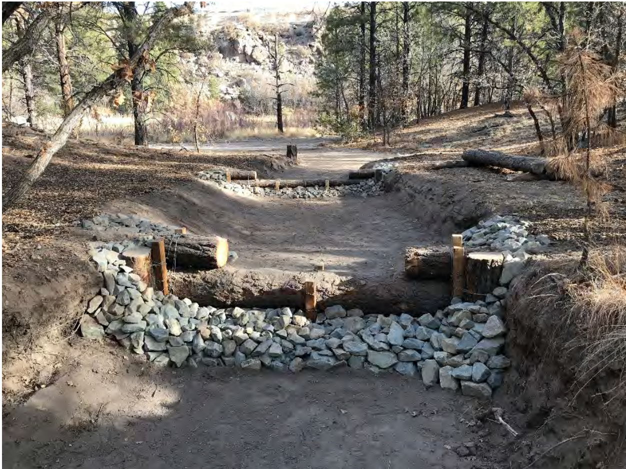
Figure E-2.1-1 January 2018: View of repaired log check dams with additional riprap erosion protection (looking downstream)
