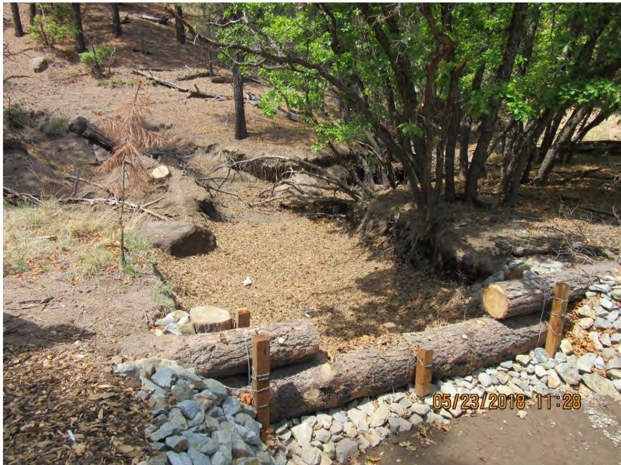
Figure E 3.9-1 May 2018: Upper log check dam
