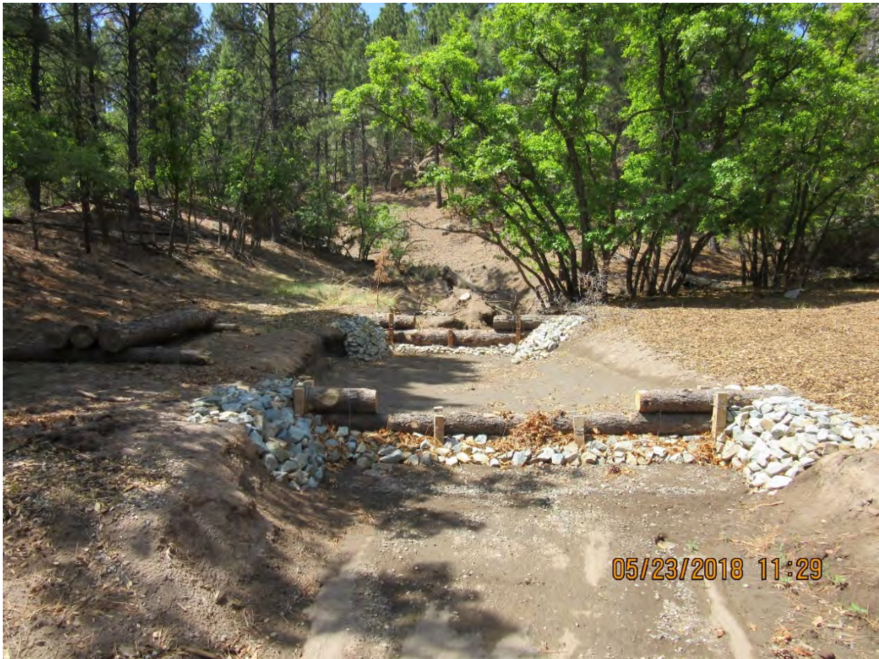
Figure E 3.10-1 May 2018: Lower log check dam
