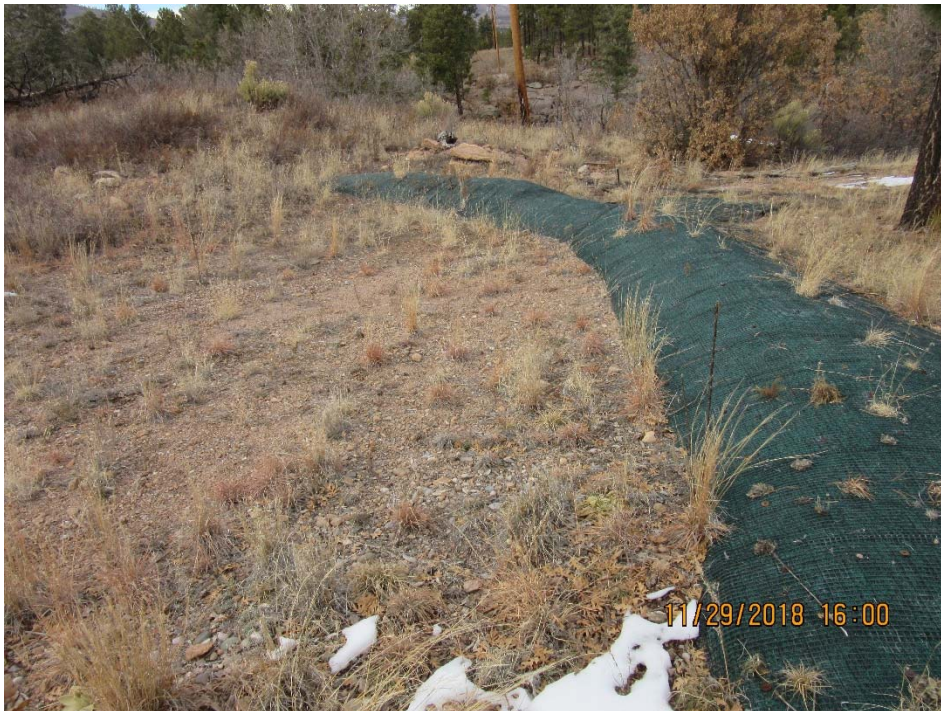
Figure 3 Earthen berm (V00703010027, center of photo) at the top of drainage leading into Fishladder Canyon (December 2018). Note established vegetation. Condition of control: excellent.
