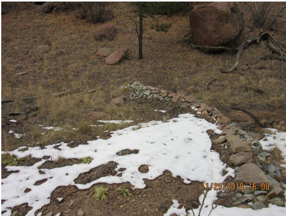
Figure 7 Rock check dam (V00706010024, center of photo) in Fishladder Canyon primary drainage (December 2018). Condition of control: very good.
