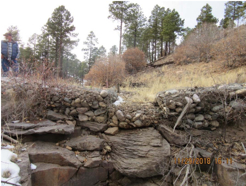
Figure 9 Gabion (V00707010002, center of photo) at access road crossing in Fishladder Canyon (December 2018). Note vegetation in channel upstream of control. Condition of control: good.
