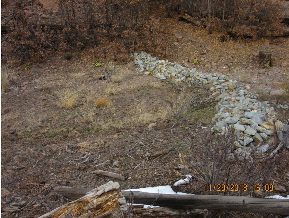
Figure 8 Rock check dam (V00706010025, center of photo) in primary drainage (December 2018). Note established vegetation in channel. Condition of control: excellent.
