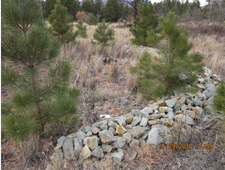
Figure 2 Rock berm (V00703120026, center of photo) at the top of drainage leading into Fishladder Canyon (December 2018). Note established vegetation. Condition of control: excellent.
