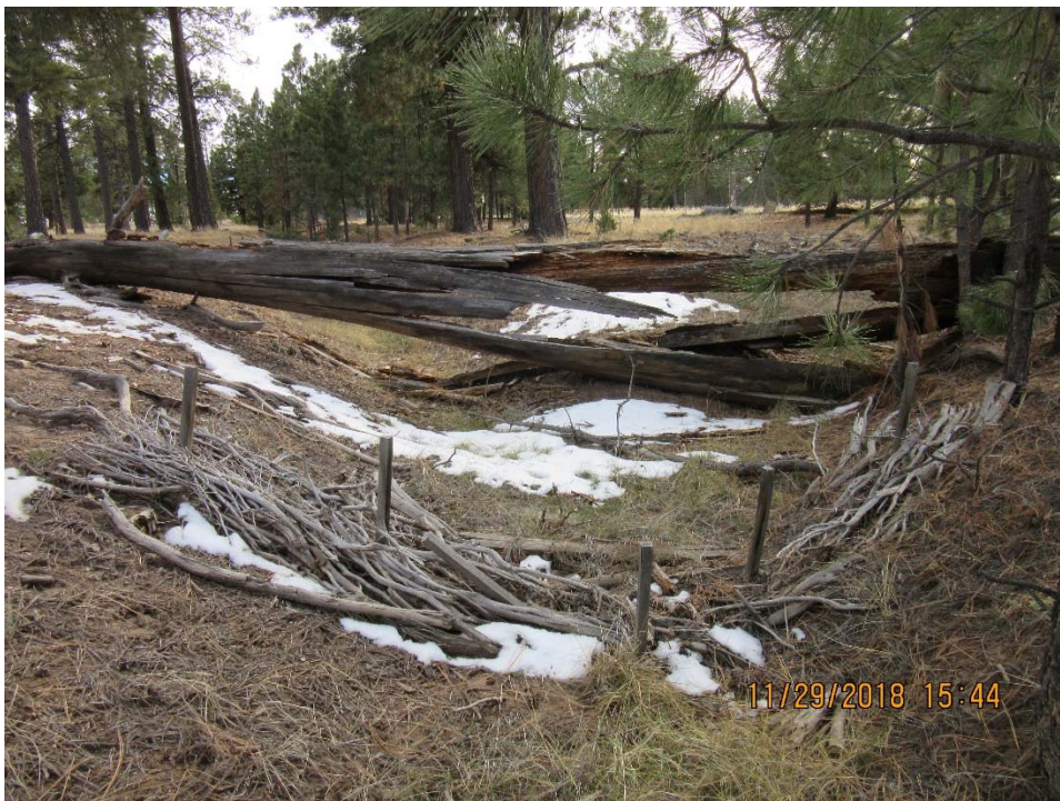
Figure 6 Juniper bale check dam located in drainage channel to 90s Line Pond, November 2018. Note vegetation in channel.
