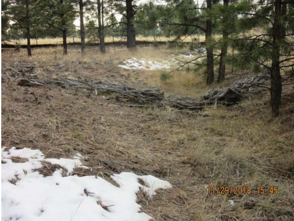
Figure 5 Juniper bale check dam located in drainage channel to 90s Line Pond, November 2018. Note vegetation in channel.
