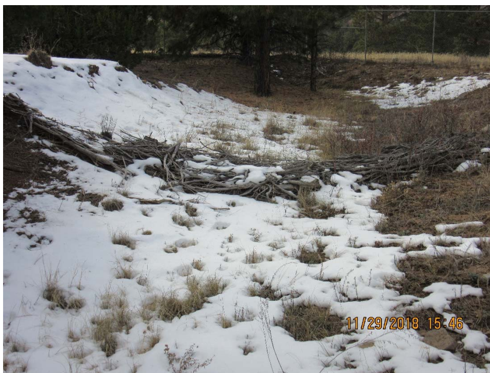
Figure 4 Juniper bale check dam located in drainage channel to 90s Line Pond, November 2018. Note vegetation in channel.
