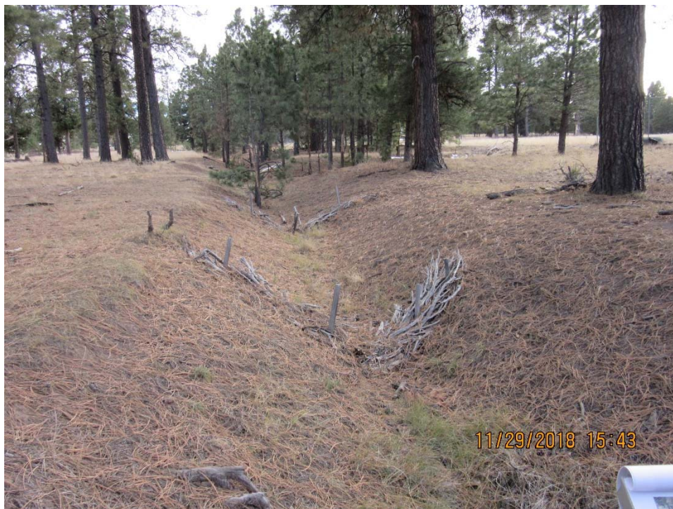
Figure 3 Juniper bale check dams located in drainage channel to 90s Line Pond, November 2018. Note needle cast and vegetation in channel.
